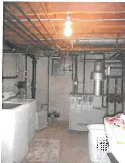
Basement, showing concrete foundation, laundry area, furnace and piping.
