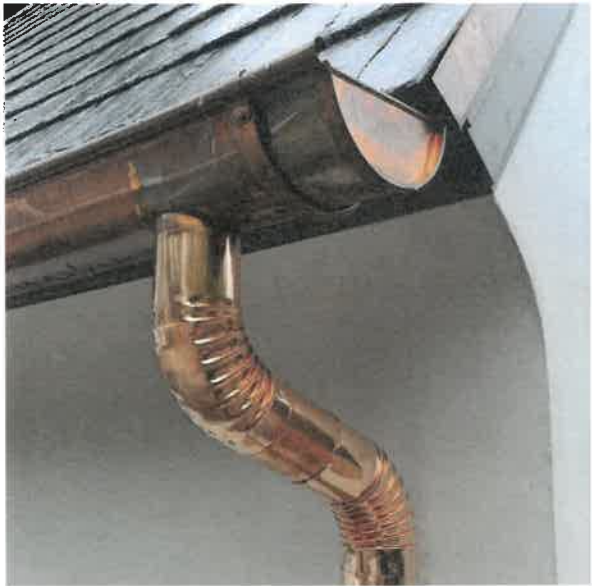
COPPER GUTTER AND DOWNSPOUT
