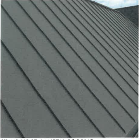
STANDING SEAM METAL ROOFING
