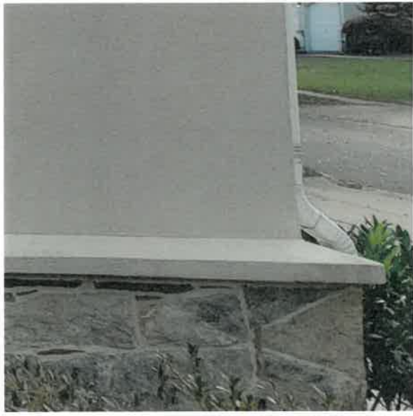
STONE WATER TABLE WITH LIMESTONE SILL
