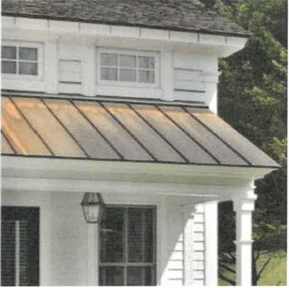
STANDING SEAM COPPER ROOFING
