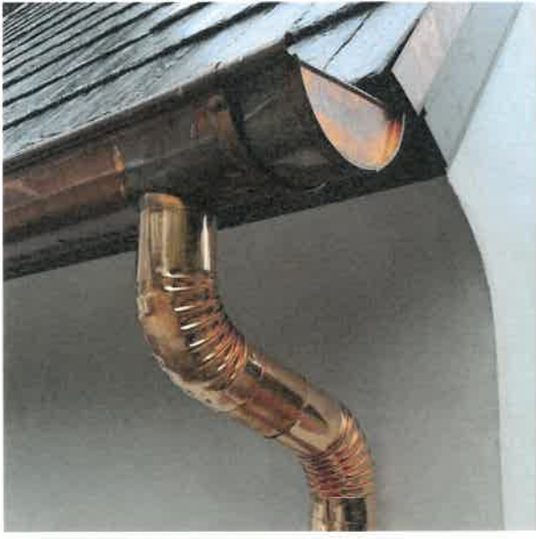
COPPER GUTTER AND DOWNSPOUT
