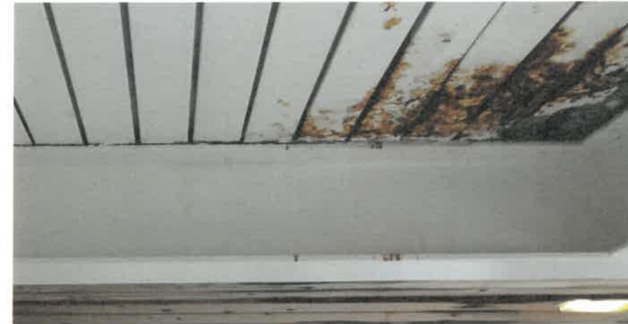
RUSTING OF METAL DECK AND SPALLING OF CONCRETE AT BALCONY FLOOR
