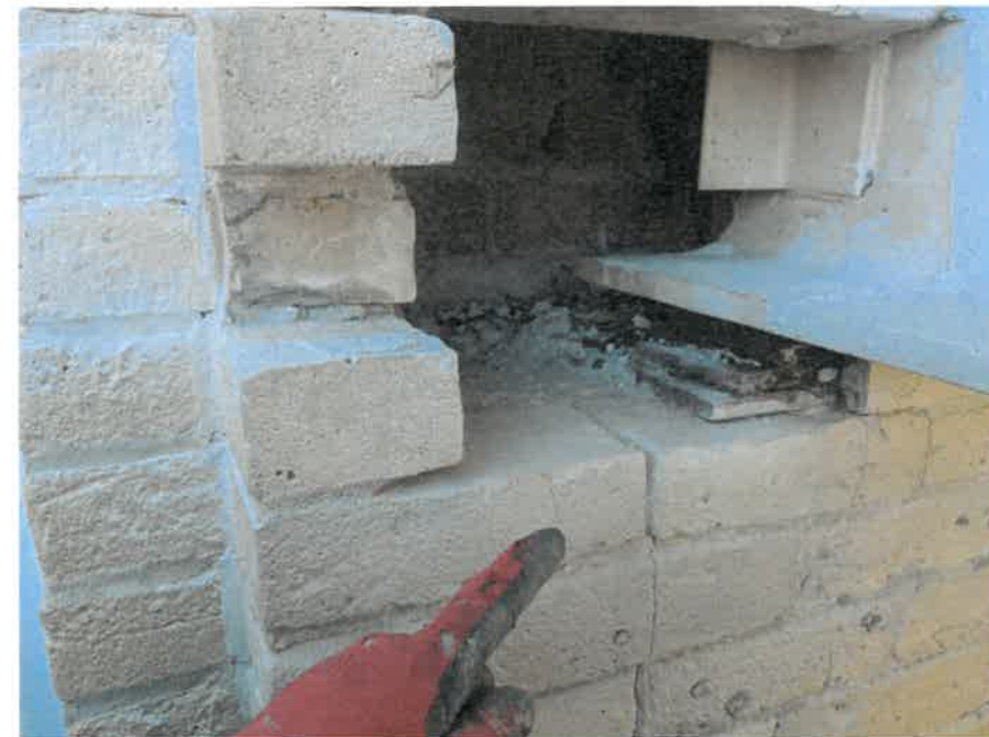
DETERIORATION AT PORCH STEEL EMBEDMENT
