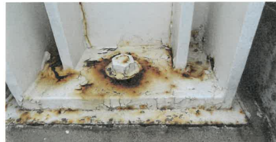
DETERIORATION AND RUSTING AT COLUMN BASE PLATES
