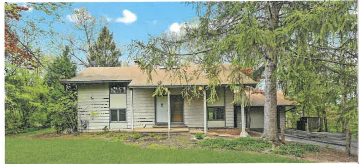
EXISTING BUILDING FRONT PHOTO
