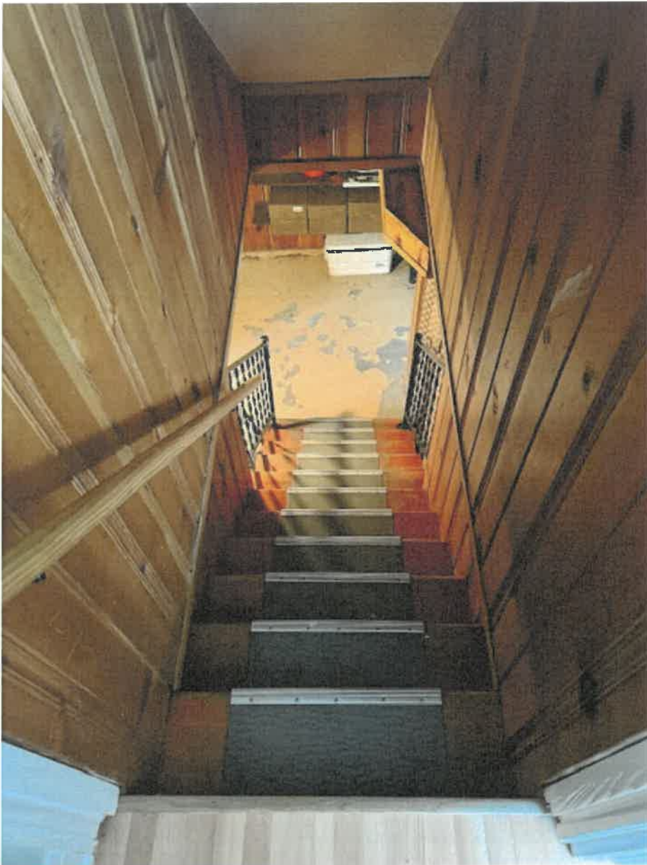
Photo K: Soffit protruding into head-room space over the staircase.
