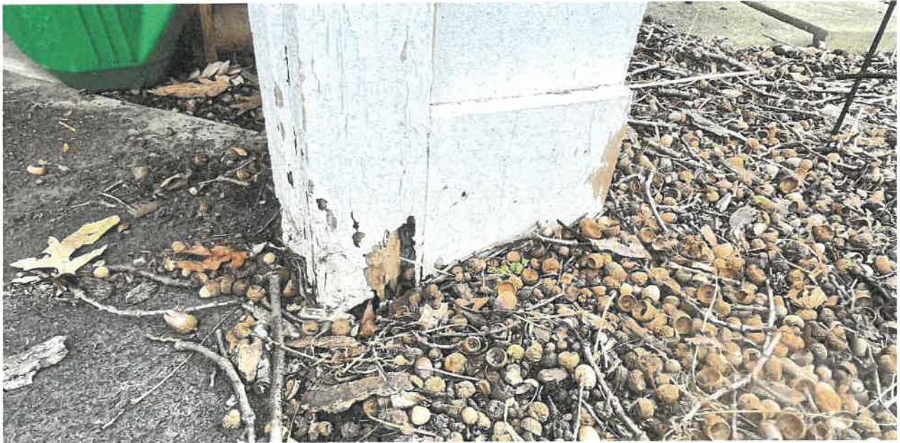
Photo N: The exterior wood on the garage is deteriorated and rotted.
