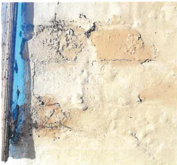
Photos G1 & G2: Efflorescence on foundation walls.
