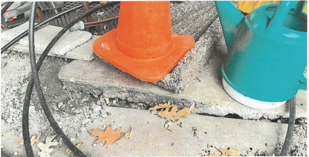
Photo 01: The garage slab is cracked and has significantly upheaved in several locations.
