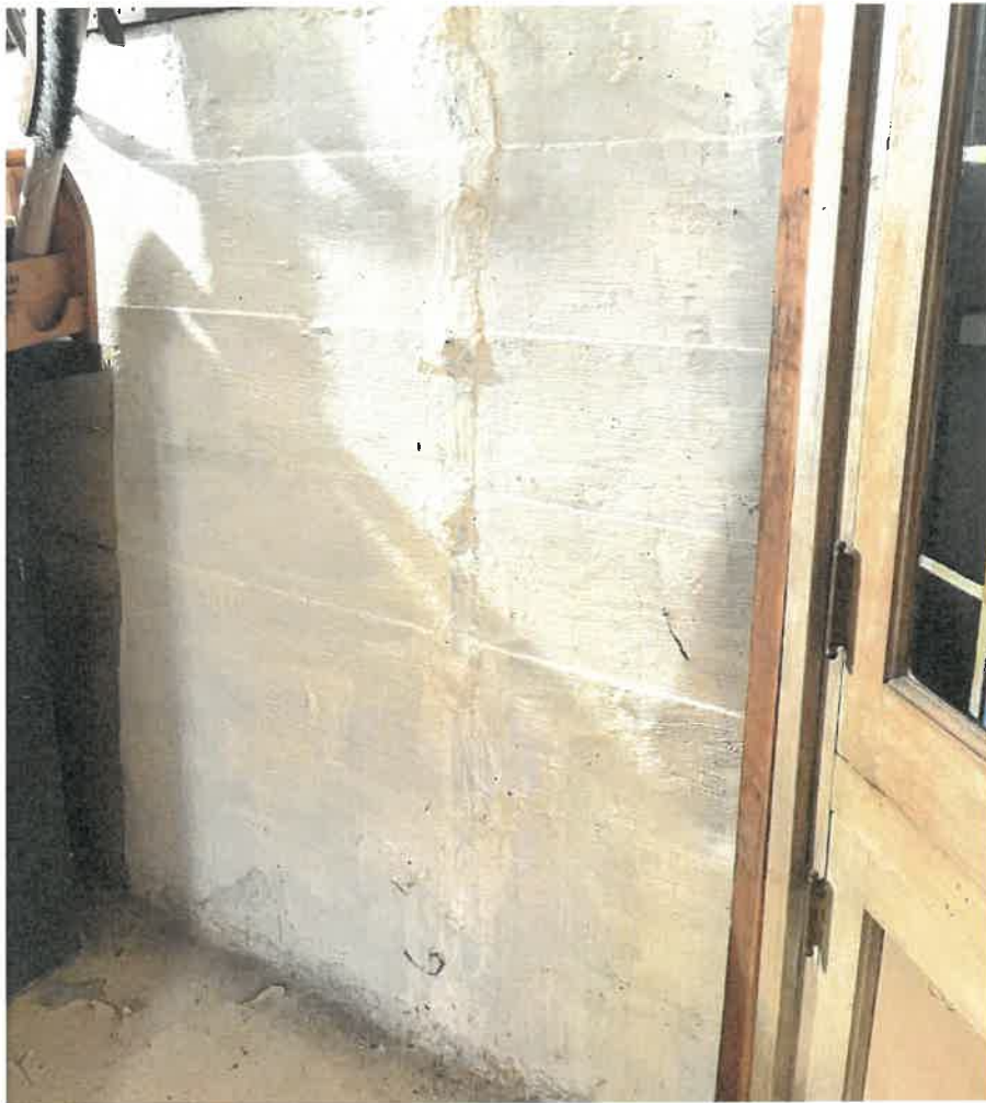
Photo F: Crack in the front foundation wall has been patched.
