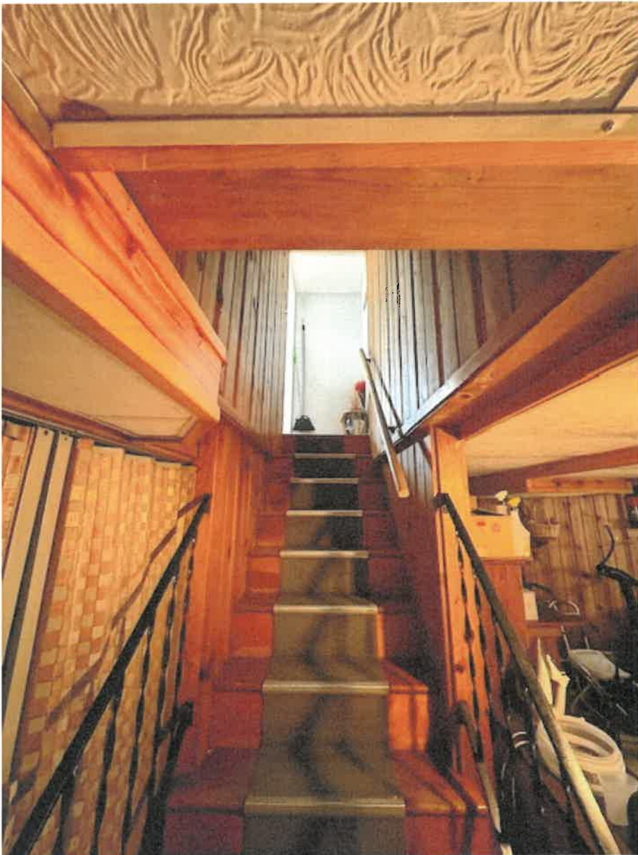
Photo L: Staircase with risers and treads that are not code compliant.
