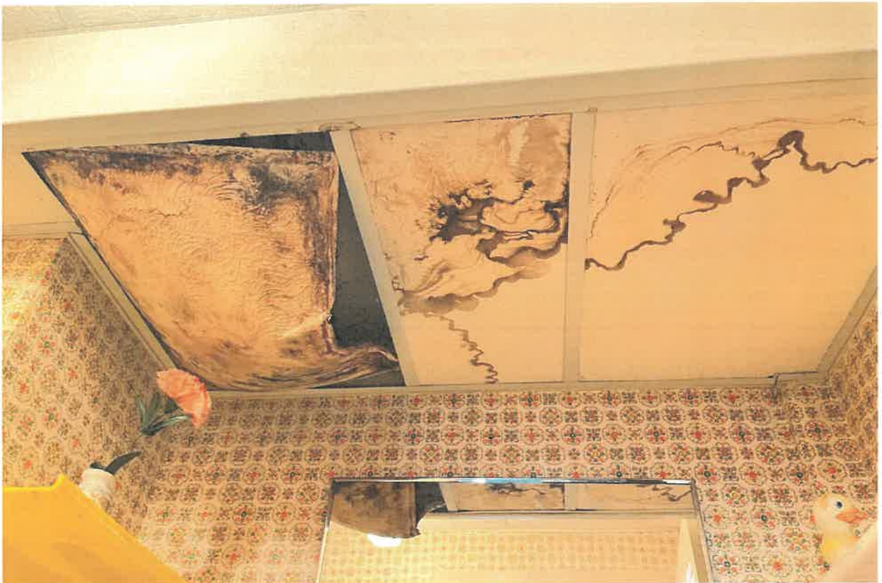
Photo H: Water damage at the ceiling.
