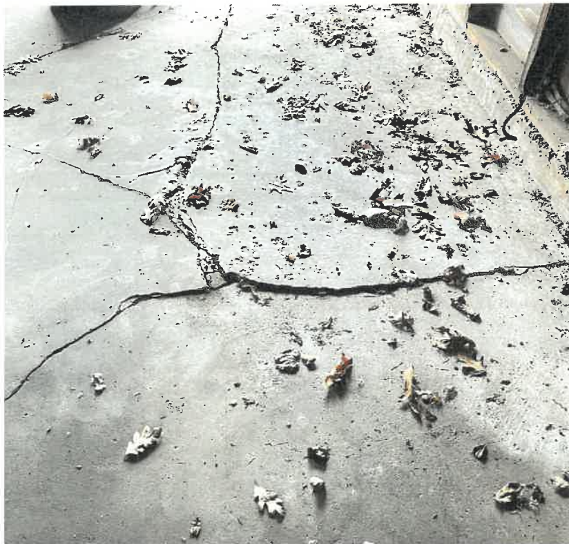
Photo 02: The garage slab is cracked and has significantly upheaved in several locations.
