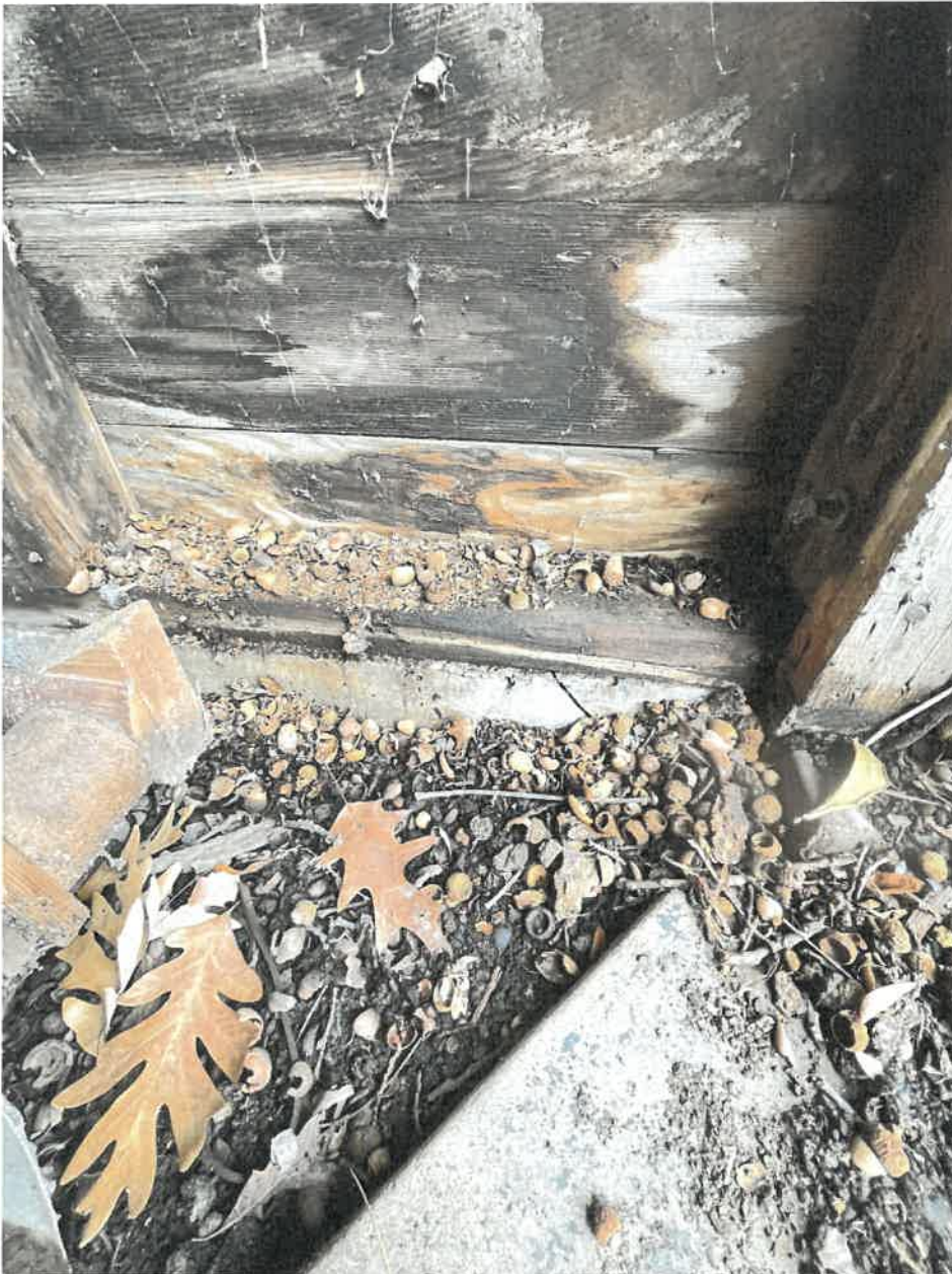
Photo P: The garage sill plates are wet and rotten, and the garage walls are wet and holding moisture.
