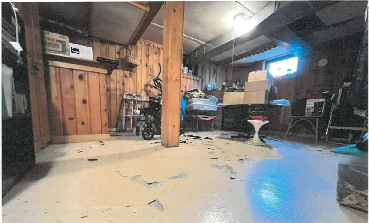
Photo C: Basement slab is upheaving in several areas (at the column in this photo).
