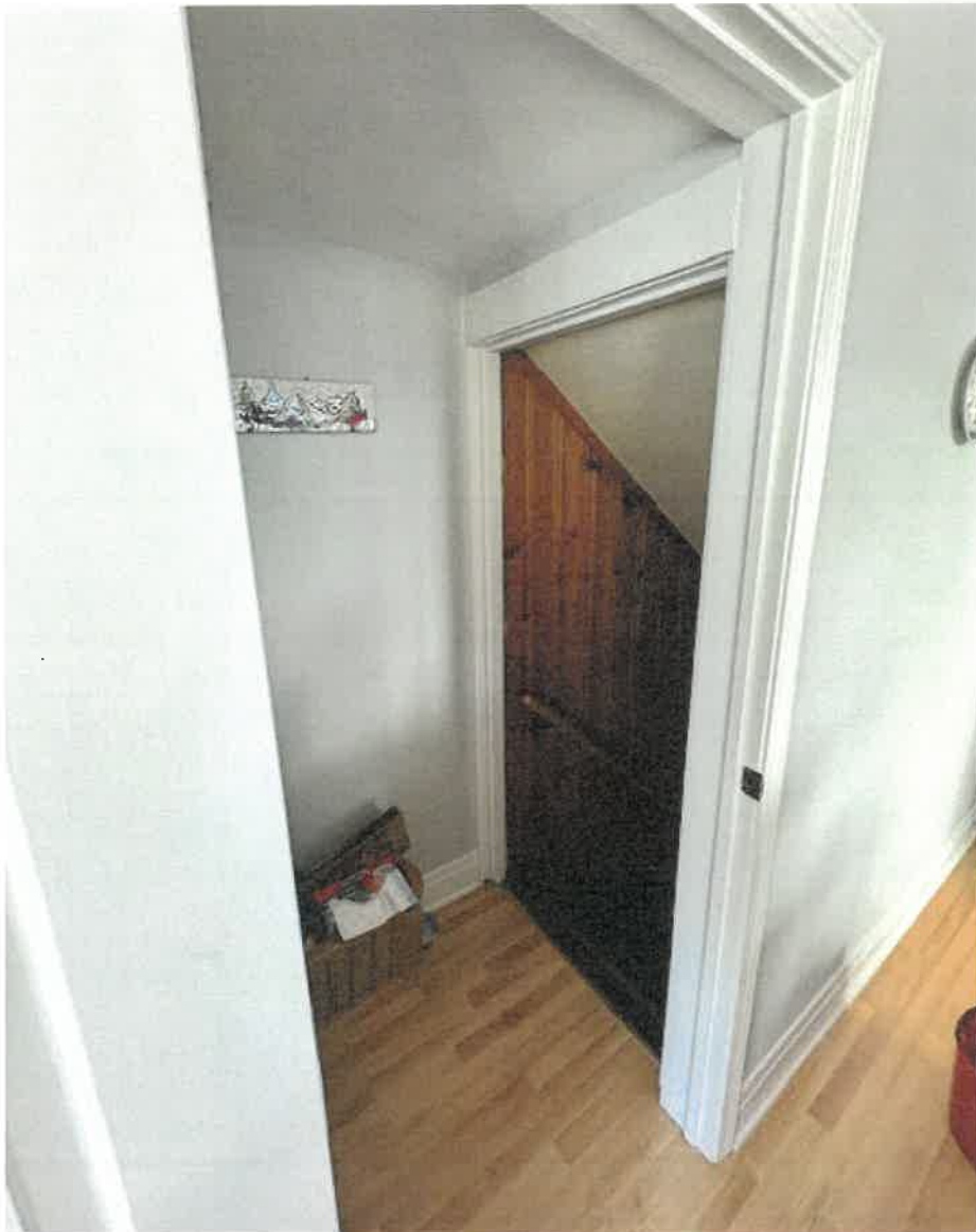
Photo J: Inadequate headroom/ceiling height at staircase to the basement.
