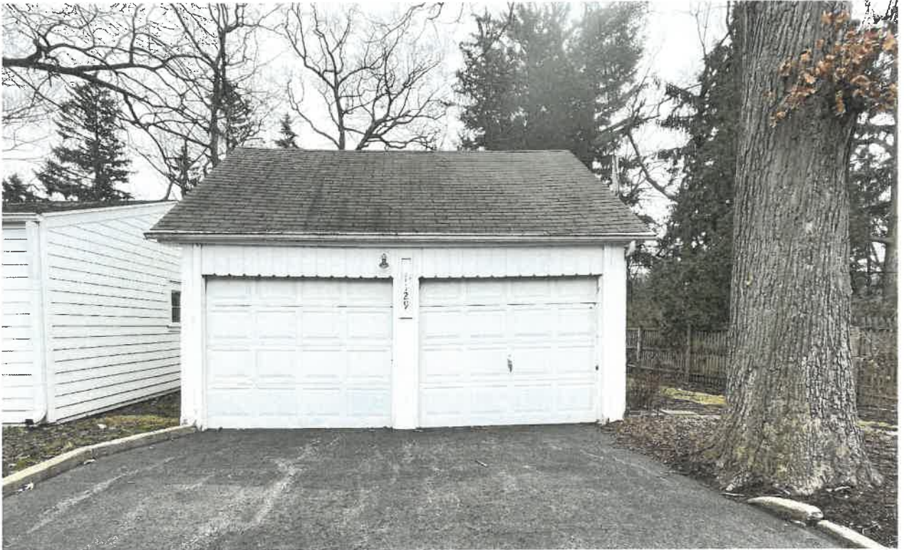
Photo M: The garage has visibly settled.
