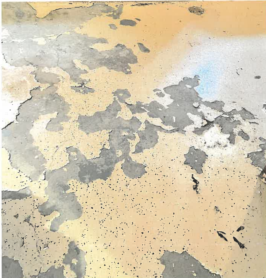
Photo E: Moisture underneath slab is causing floor finish to peel.
