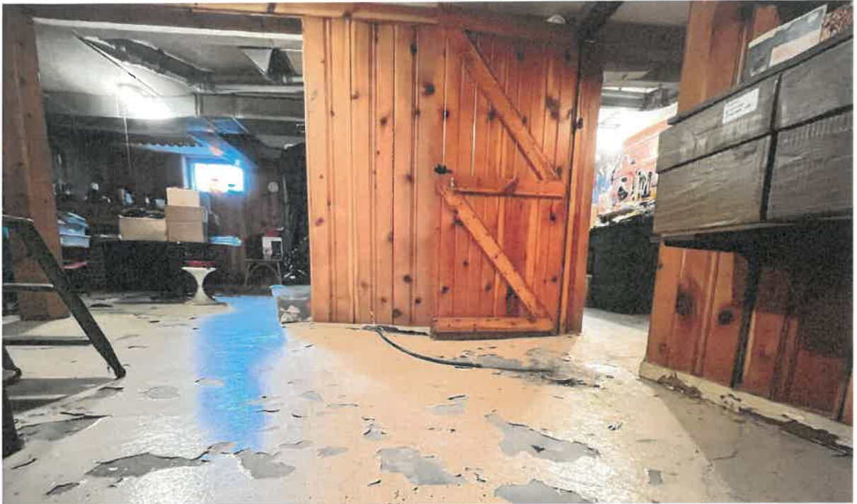
Photo D: Severely sloping slab throughout the basement.
