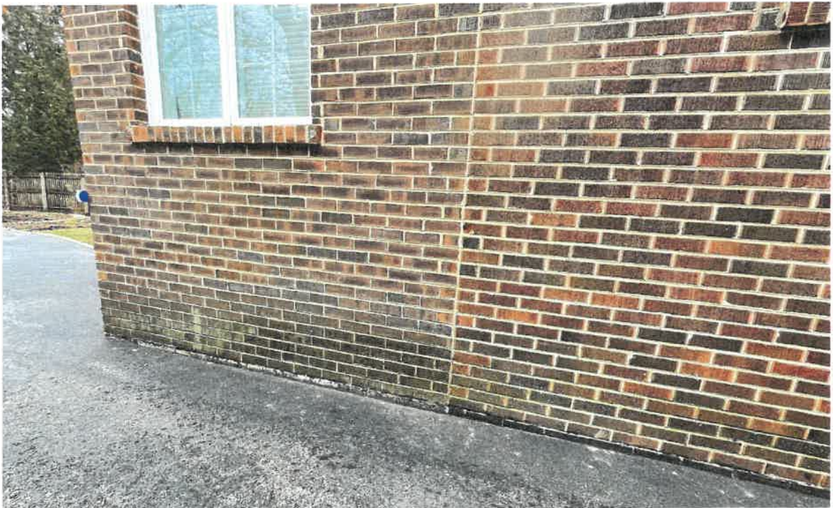
Photo A: Discolored bricks along the driveway.
