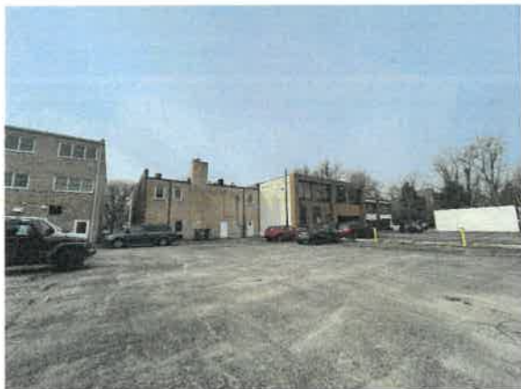
Photo 13: adjacent parking lot behind building, looking northwest
