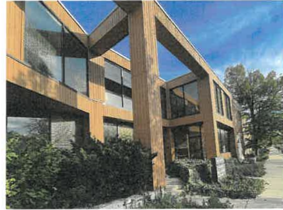
Photo 6: front of building from sidewalk, looking south
