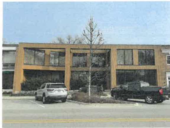
Photo 1: front, west elevation
