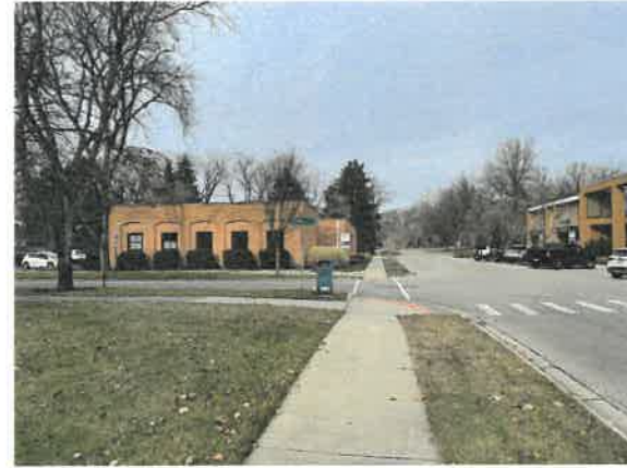
Photo 11: looking north up street, 1401 on the right
