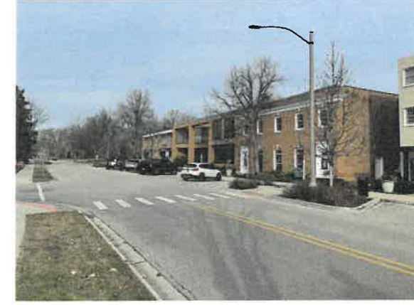
Photo 8: from street, looking northeast at 1401 and adjacent buildings
