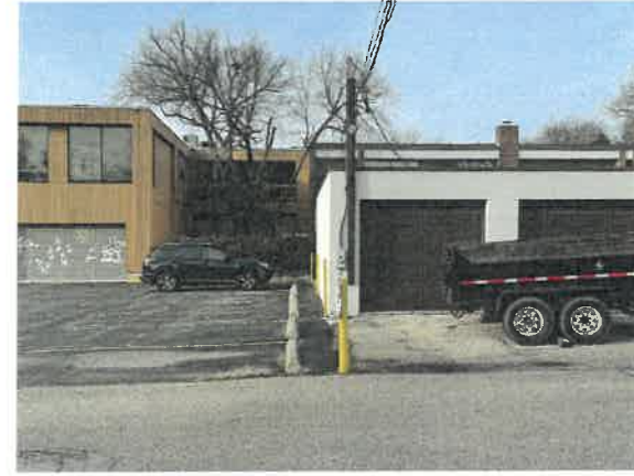
Photo 3: rear, partial east elevation
