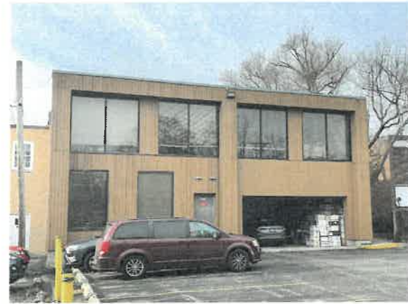
Photo 2: rear, partial east elevation
