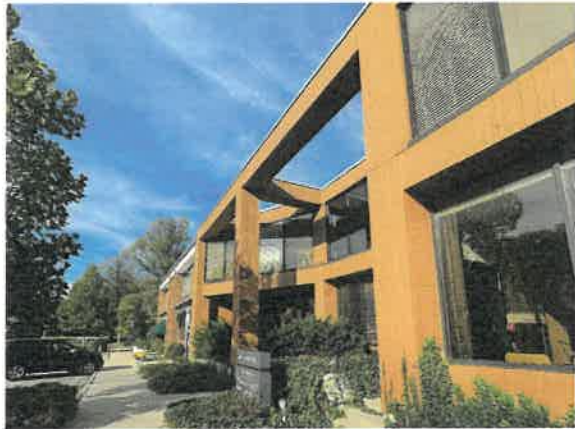
Photo 5: front of building from sidewalk, looking north
