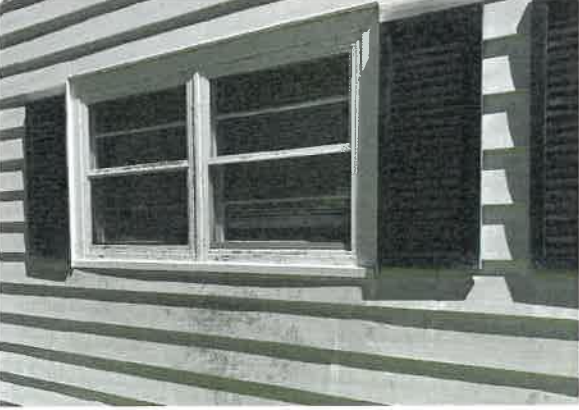
DETERIORATING WINDOWS AND SIDING THROUGHOUT EXTERIOR
