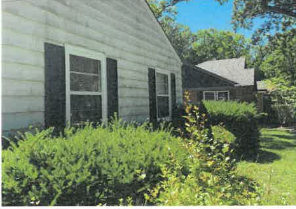
DETERIORATING WINDOWS AND SIDING THROUGHOUT EXTERIOR
