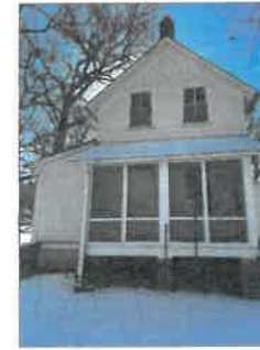
North Elevation of Existing Residence
