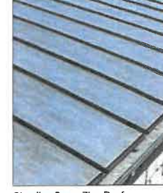
Standing Seam Zinc Roof
