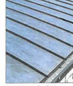
Standing Seam Zinc Roof
