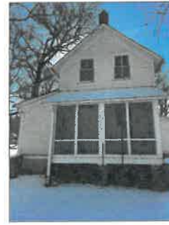
North Elevation of Existing Residence
