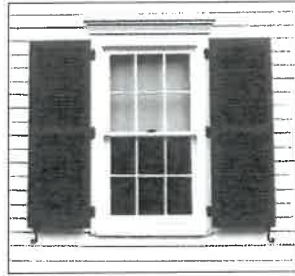
Proposed Shutters: Historically Correct Wood Louvered w/ Cast Pintel Hinges & Shutter Dogs
