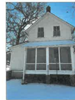
North Elevation of Existing Residence
