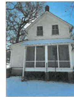
North Elevation of Existing Residence
