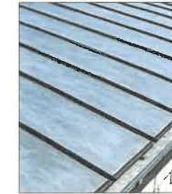
Standing Seam Zinc Roof
