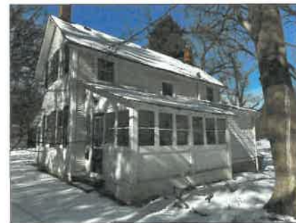
East Elevation of Existing Residence
