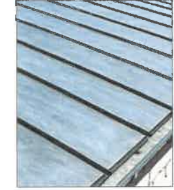
Standing Seam Zinc Roof
