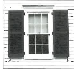
Proposed Shutters: Historically Correct Wood Louvered w/ Cast Pintel Hinges & Shutter Dogs
