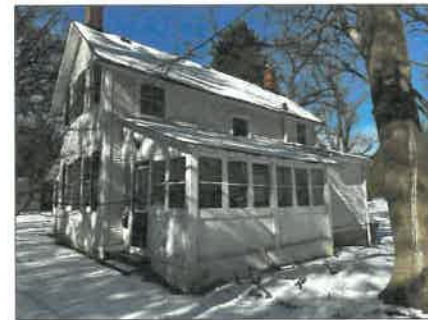
East Elevation of Existing Residence
