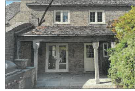
7 From East - Covered Dining Room Area
