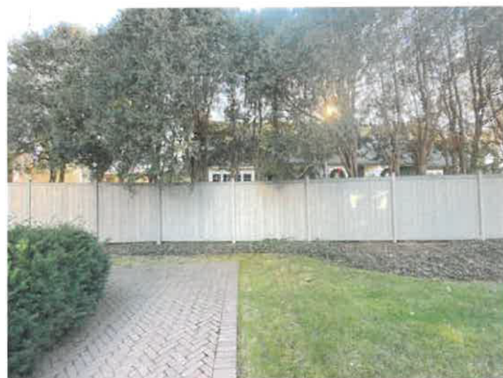
BACK FENCE, LOOKING INTO NEIGHBOR'S LOT - #4
