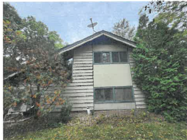
EXISTING SIDE VIEW
