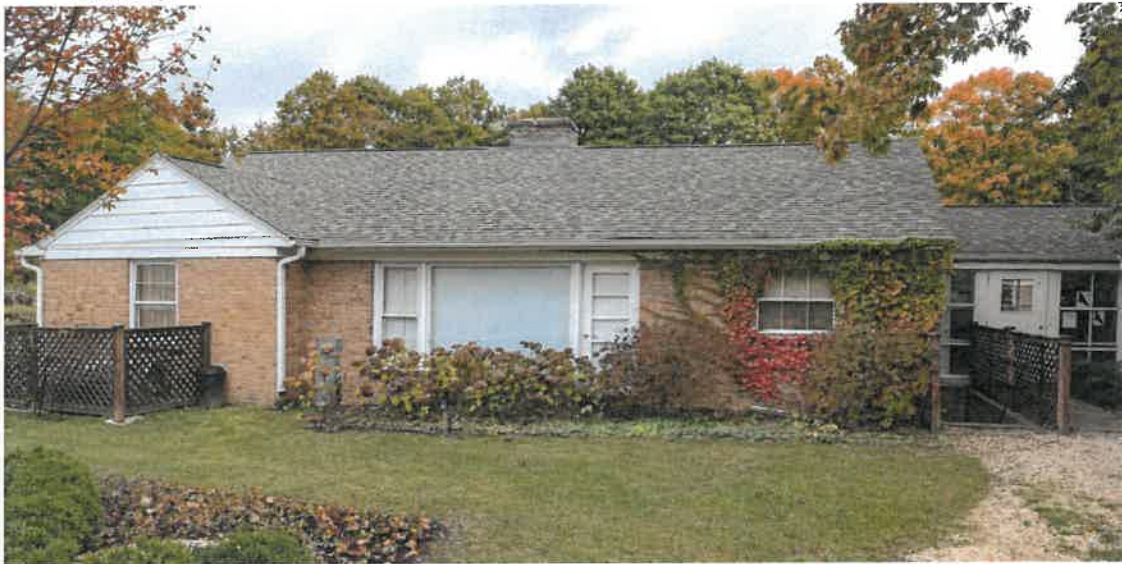
Existing condition of internal to site entry
