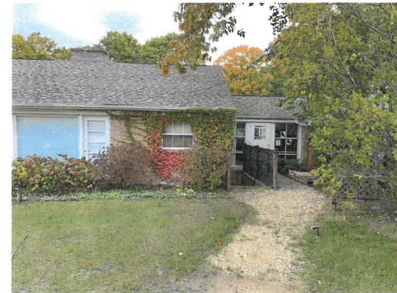
EXISTING WEST ELEVATION - PARKING LOT VIEW
