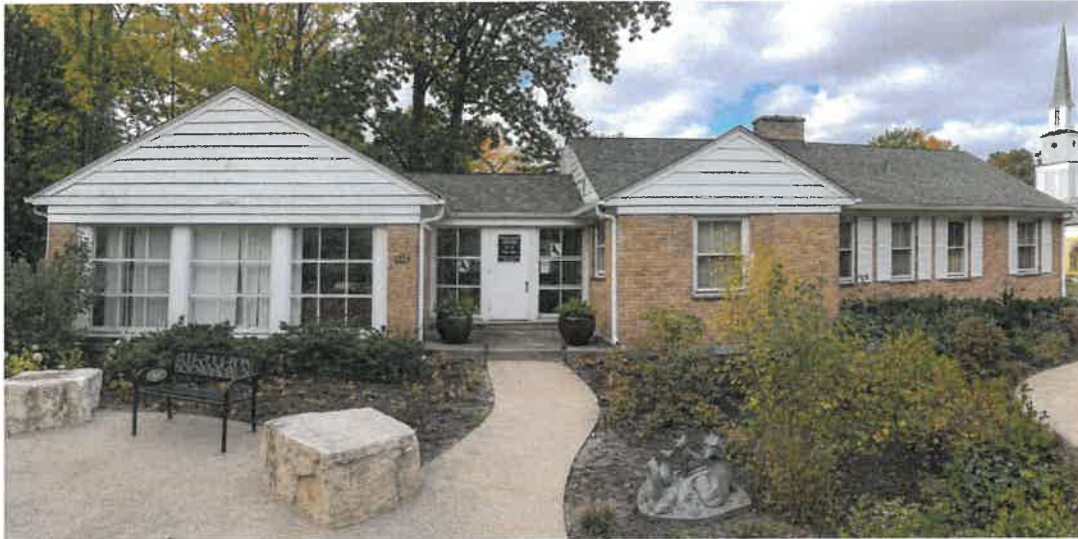
Existing condition Washington Street Elevation
