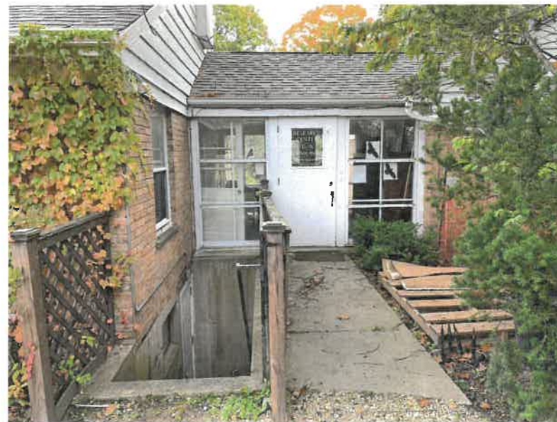
EXISTING WEST ELEVATION - PARKING LOT VIEW
