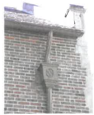
Typical slate roof with decorative scupper box and twisted copper downspout
