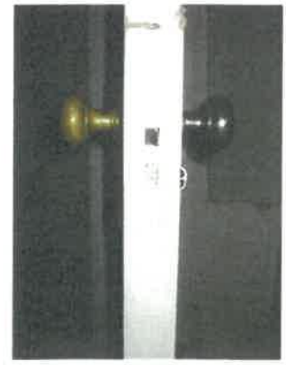
Typical hardware at coach house
