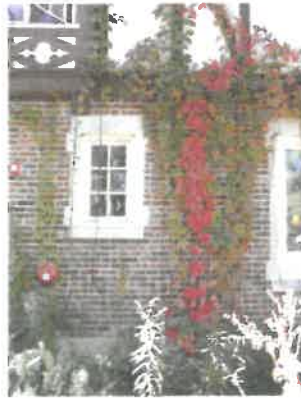
Small window at north elevation of secondary wing
