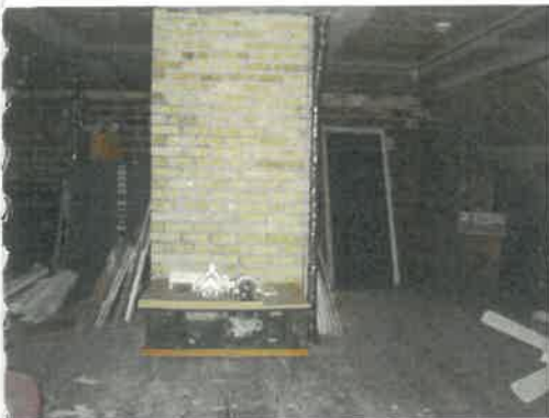
Detail of chimney at 3rd floor attic
