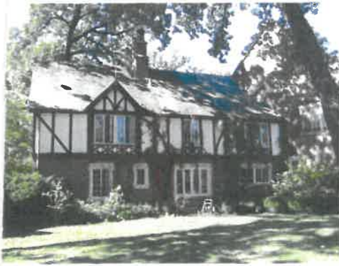
North elevation, secondary wing
