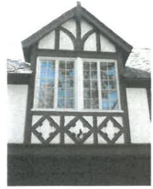
Detail of large dormer at north elevation of coach house
