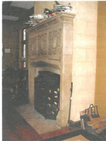
Figure 19. Fireplace at living room with faux-finished plaster walls. (BHC)
