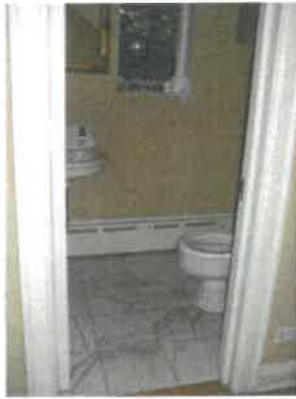
Toilet room at kitchen hallway
