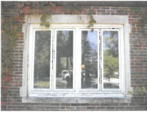
Replaced windows at secondary wing
