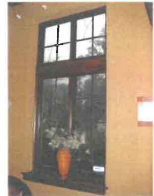
Window at living room
