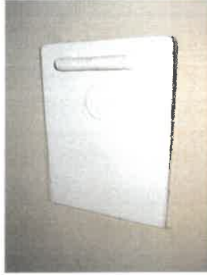
Second floor incinerator chute
