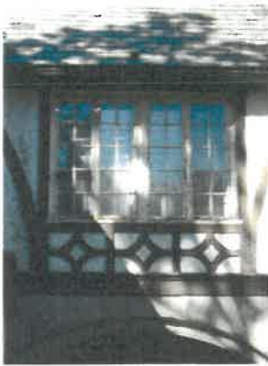
Rough stucco and decorative half-timbering at west elevation of porte cochere (also occurs at west elevation of porte cochere)
