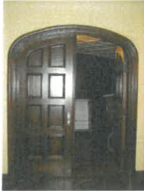
Typical Tudor arch doorway showing rough plaster walls, wood baseboards and heavy paneled doors with hammered metal hardware.
