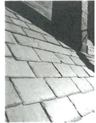
Detail of slate roof at coach house
