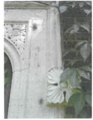
Detail of south elevation stonework at doorway
