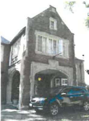
View of the front facing gable of the porte cochere
