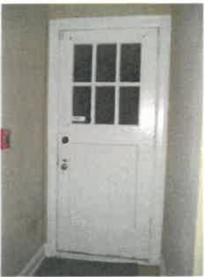
Exterior door at east elevation of secondary wing
