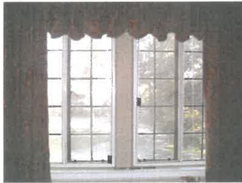
Typical multi-paned, steel casement windows
