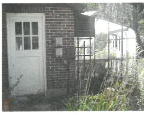
Detail of greenhouse attached at the south elevation of coach house
