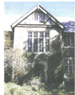
Detail of the projecting front facing gable at the south elevation of the main wing
