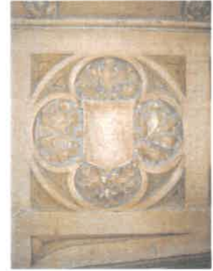
Detail of stone quatrefoil at fireplace in living room
