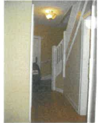
Former servan'ts stairs at kitchen
