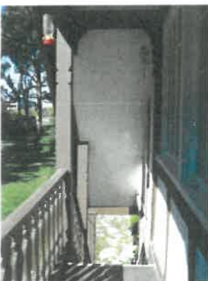
Detail of coach house balcony, looking west
