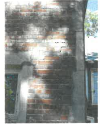
Variegated brick walls with stone trim and quoining
