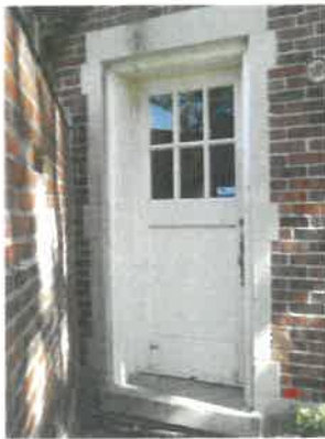
Detail of doorway at east elevation of secondary wing
