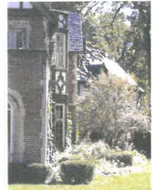
Detail showing Tudor Revival style building materials: variegated brick, rough stucco with half timbering, slate roof, multi-paned casement windows, and decorative stonework.
