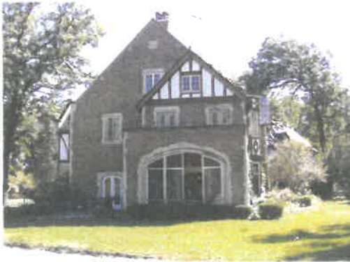
West elevation of the main wing
