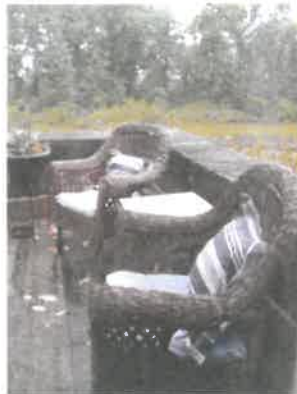
Detail of exterior balcony beyond master bedroom
