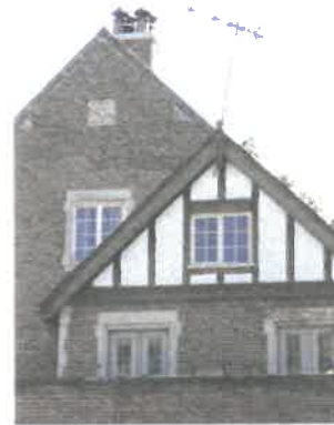
Detail of the west elevation of the main wing, showing gable extension with half timbering and balcony of master bedroom
