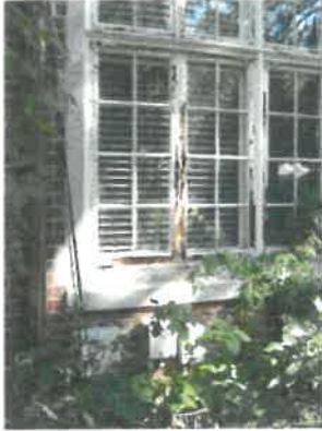
Typical steel frame, multi-paned, casement windows
