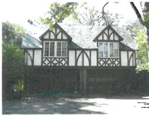
Coach house, north elevation, showing first floor garage entrance
