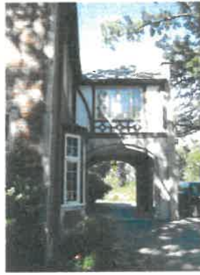
View of east elevation of porte cochere
