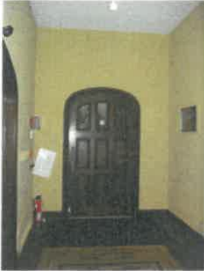
Main door at north elevation
