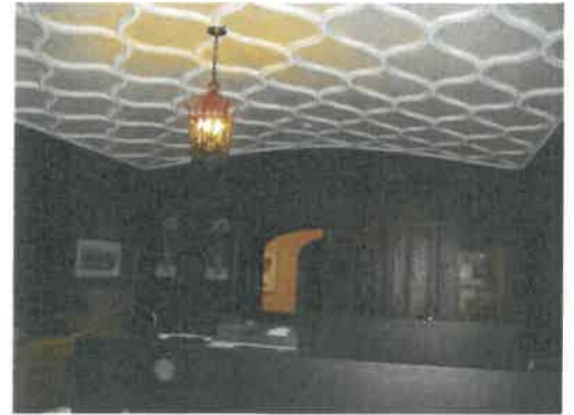
Dining room with wall panelling and curved plaster ceiling with decorative strapwork
