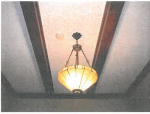
Detail of plaster ceiling at second floor mezzanine
