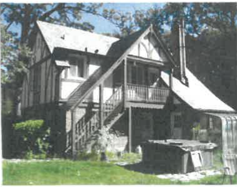
Coach house, south elevation with entrance to apartment at second floor
