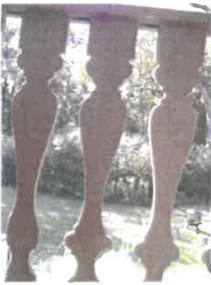
Detail of brackets at coach house balcony
