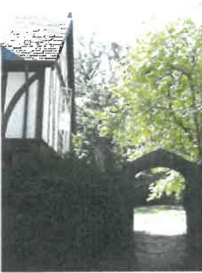
Coach house west elevation, showing attached brick and stone wall connection to main house
