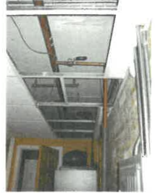
Detail of ceiling at first floor coach house
