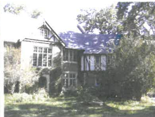
South elevation at the main wing and secondary wing
