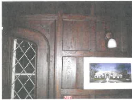
Detail of woodwork at library, showing French doors with diamond patterned leaded glass
