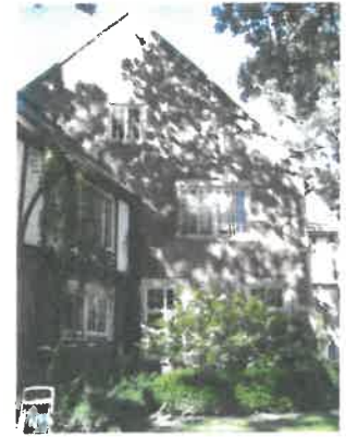
east elevation of the main wing (where it connects to the secondary wing)
