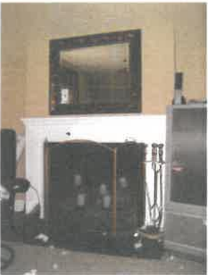
Detail of fireplace at living room at coach house
