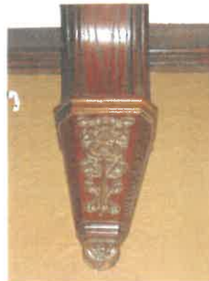
Decorative wood bracket at exposed ceiling beams at living room
