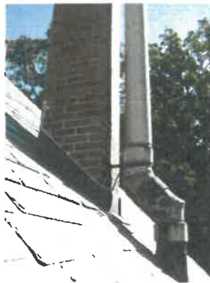
Detail of chimney at coach house
