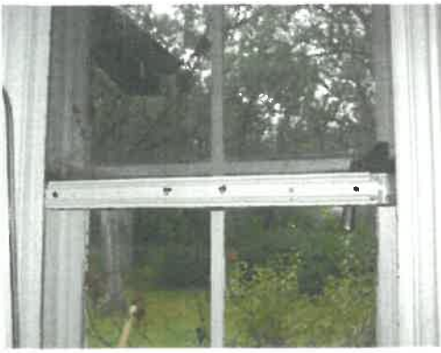
Detail of pull-down shutters at master bedroom windows
