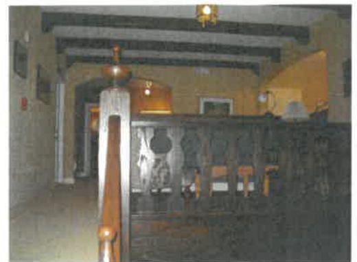
Second floor mezzanine
