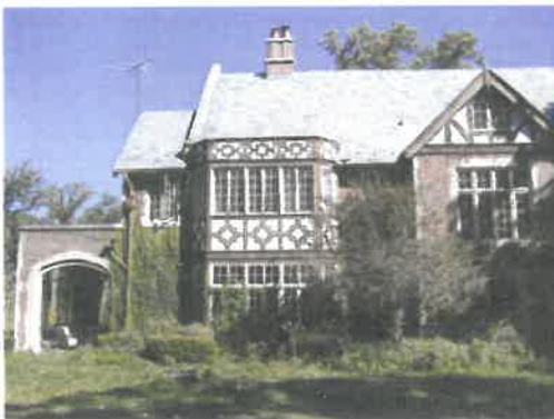
South elevation of the main wing at the west side
