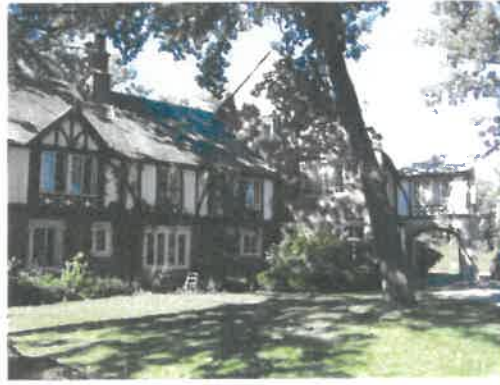
north elevation, secondary wing and main wing
