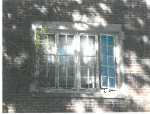
Typical multi-paned, steel, casement windows
