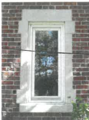
Small replaced window at north elevation of secondary wing
