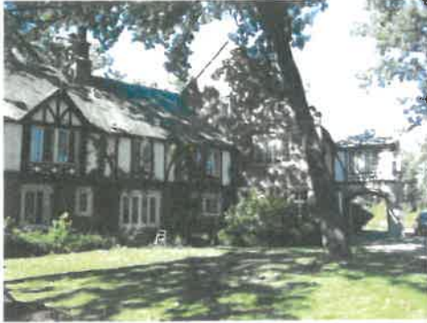
Figure 16. David Everitt House, view of secondary wing and main wing with porte cochere. (BHC)
