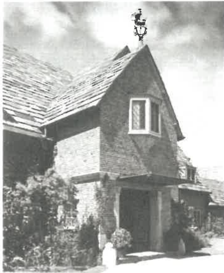
Figure 12. West View Farms, the Robert P. Lamont house, front entrance.
