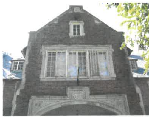
Detail of the front facing gable of the porte cochere
