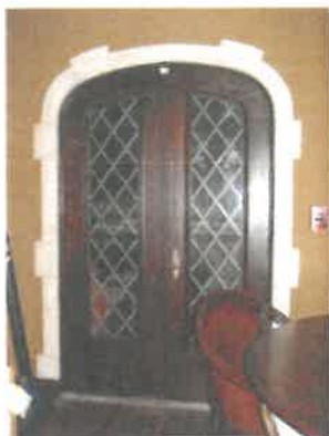
Detail of French doors at living room with faux-plaster quoins
