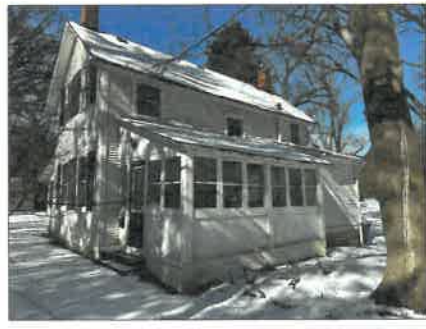
East Elevation of Existing Residence
