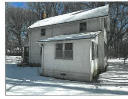
West Elevation of Existing Residence
