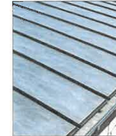
Standing Seam Zinc Roof
