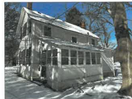
East Elevation of Existing Residence
