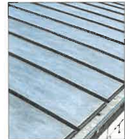
Standing Seam Zinc Roof
