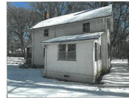
West Elevation of Existing Residence
