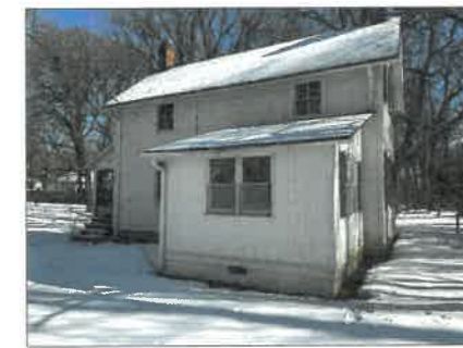
West Elevation of Existing Residence
