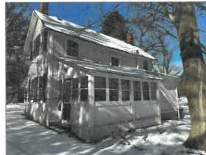
East Elevation of Existing Residence
