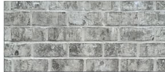
Proposed Face Brick Cherakee (Ansley Park) w/ Regular Mortar Joints
