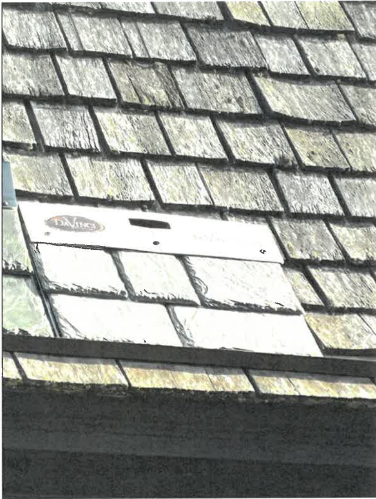
Image of DaVinci "Weathered Green", Multi-Width Slate sample on existing cedar roof
