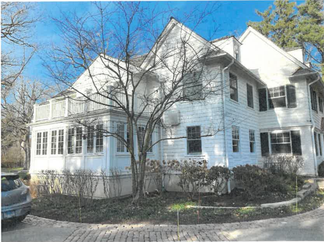
View showing side (south) façade of home
