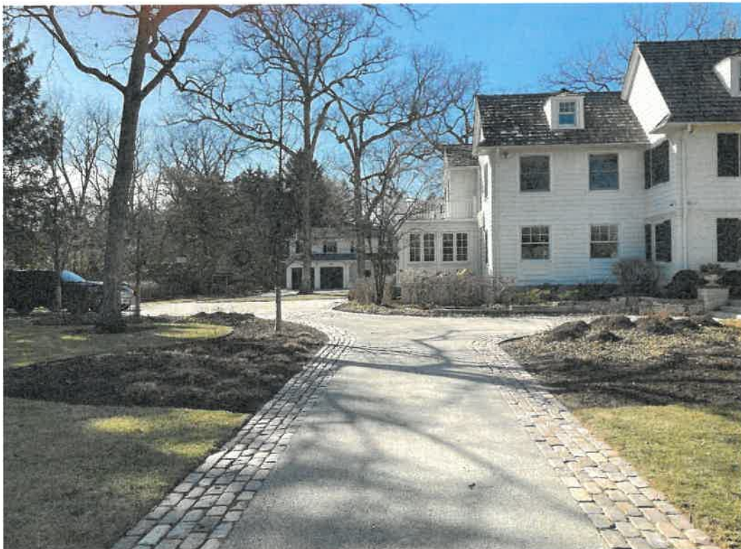
View from Elm Tree Rd showing coach house beyond (left) and house (right)
