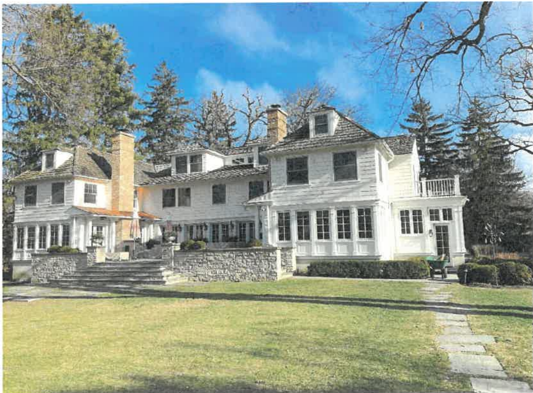
View showing rear (west) façade of home
