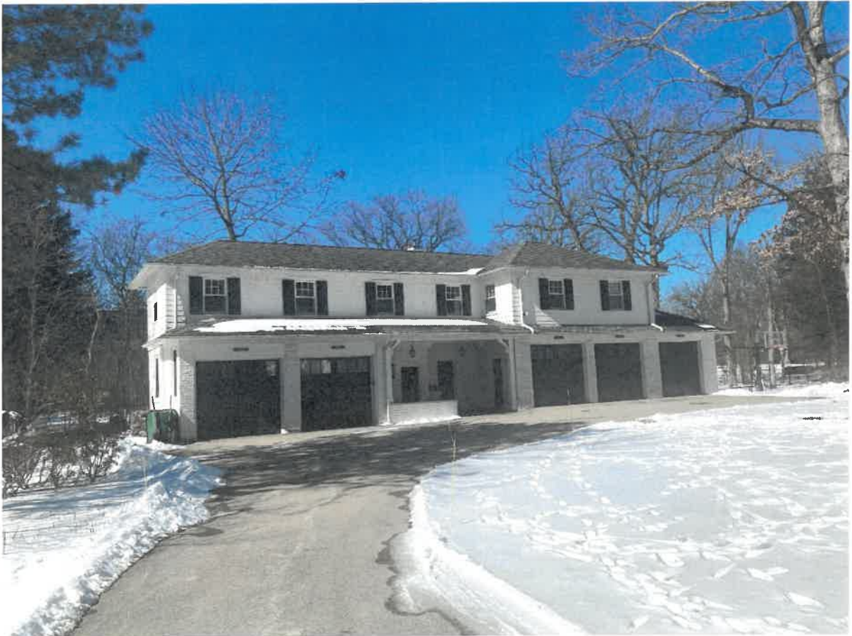
Garage Structure for the Marvin Hughitt Frost Estate House, Photo 2025
