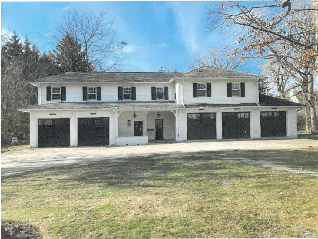
View showing front (east) façade of coach house
