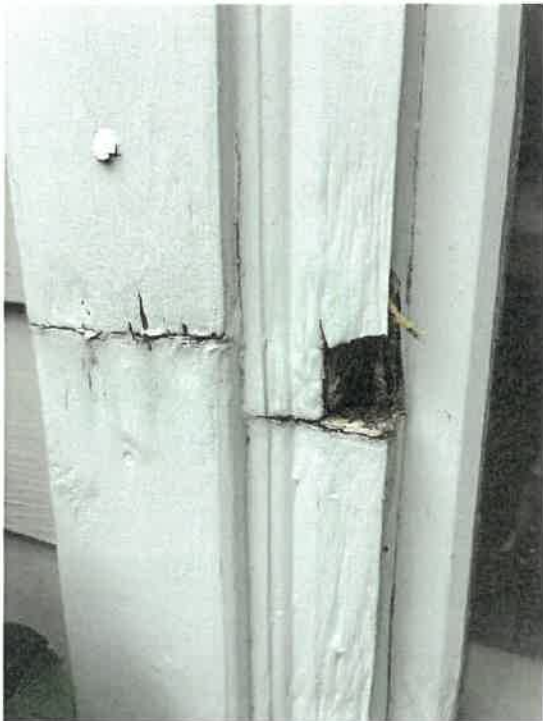
Wood window condition
