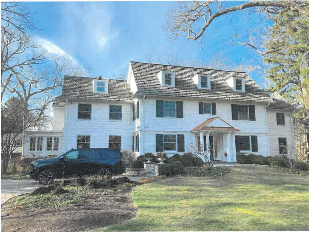
View showing front (east) façade of home
