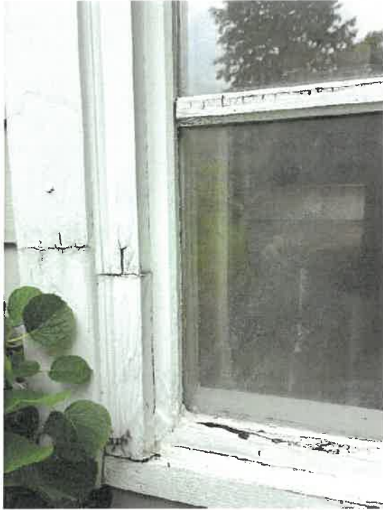
Wood window condition
