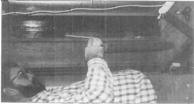
Maintaining a historic window may include work as basic as replacing a sash cord.
