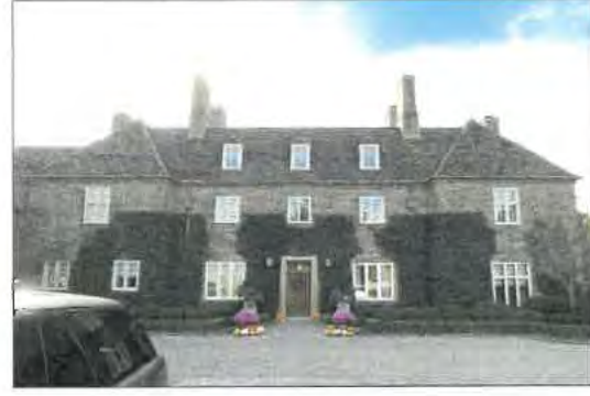
11 From North - Front Entry
