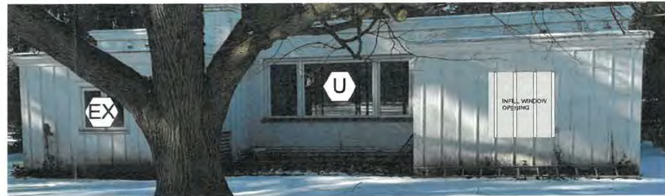
VIEW 4 REPLACE WINDOW UNIT 'U' WITH NEW WINDOW . 'EX' WINDOW TO REMAIN. REMOVE EXISTING WINDOW AND INFILL WITH SIMILAR EXTERIOR SIDING
