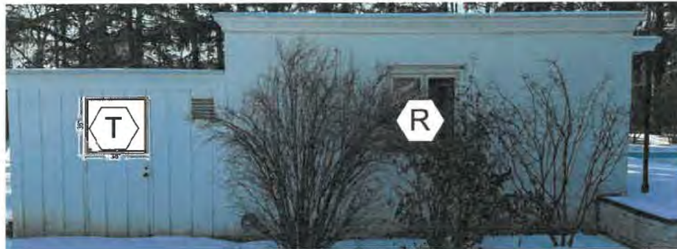
VIEW 3 REPLACE WINDOW UNIT 'T' WITH NEW WINDOW REPLACE EXISTING DOOR WITH NEW FIXED WINDOW PATCH IN SIDING TO MATCH EXISTING.
