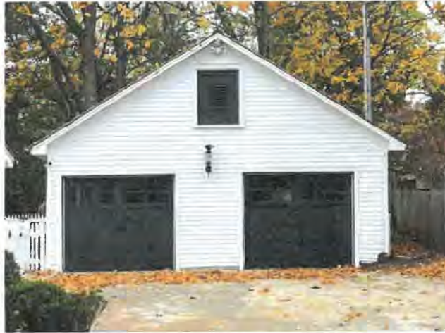
Existing Garage (east façade) with unbalanced left-side garage door location.
