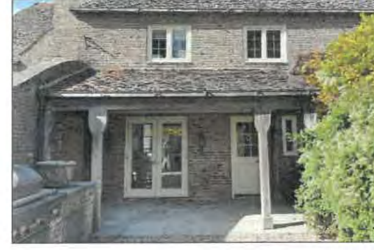
7 From East - Covered Dining Room Area
