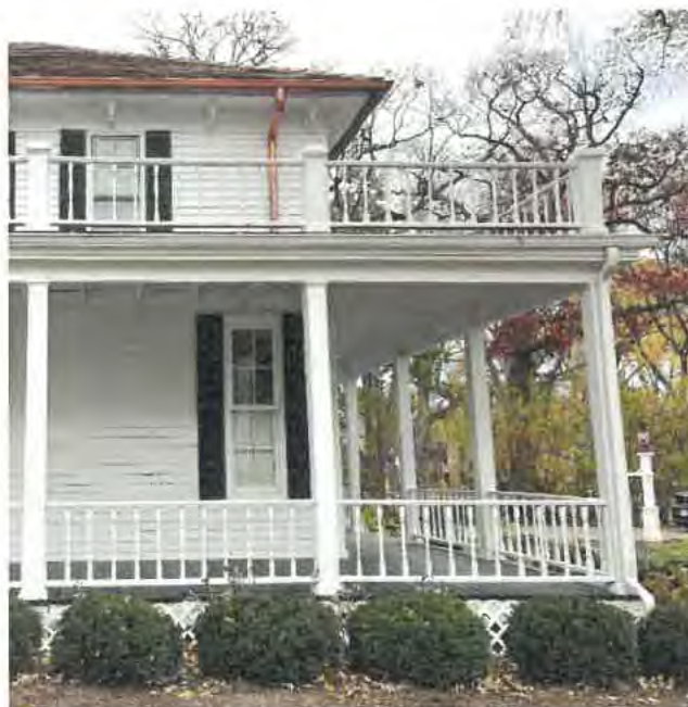
Existing Front Porch as viewed from the side (south).
