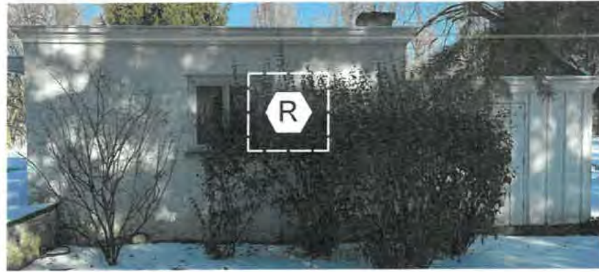
VIEW 1 REPLACE WINDOW UNIT 'R' WITH NEW WINDOW IN NEW LOCATION, PATCH AND PAINT SURROUNDING MASONRY TO MATCH EXISTING
