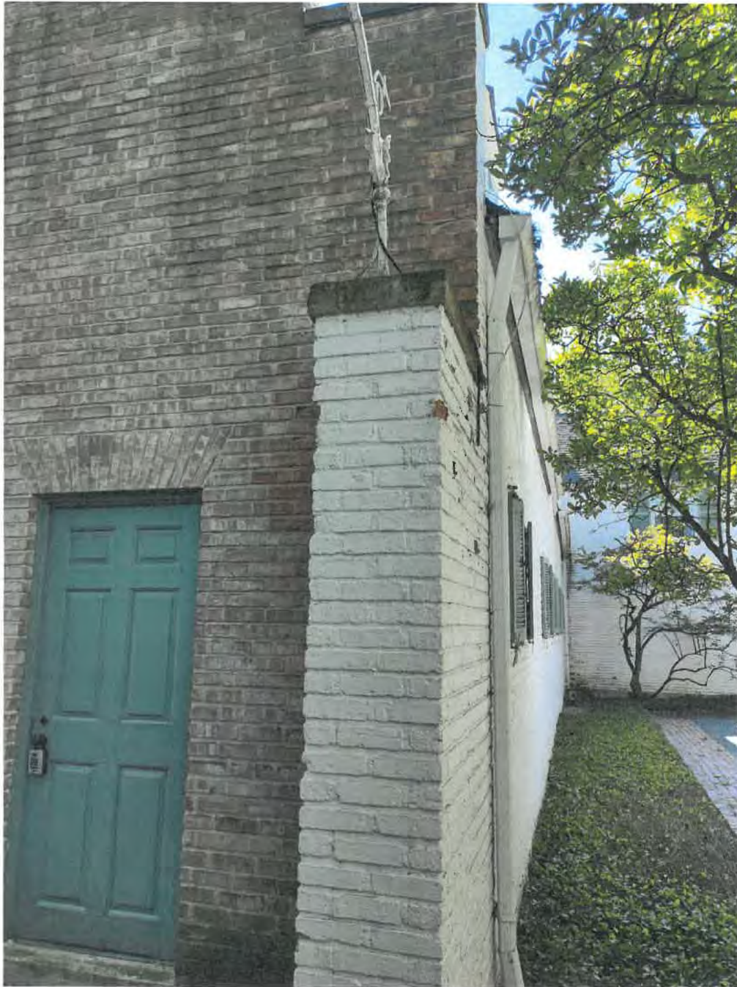
EXISTING PHOTO- NORTH ELEVATION PAINT TRANSITION
