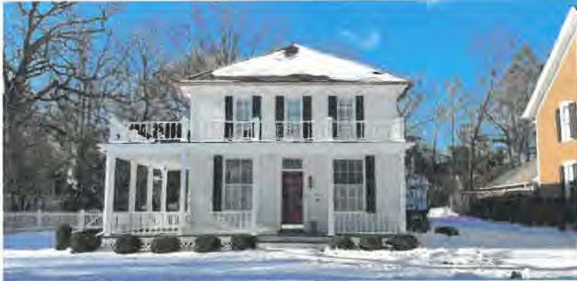
Existing Front Façade (east). Notice the two wider first floor windows, each with one very narrow shutter.
