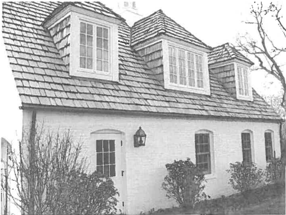
View of Addition's North Elevation, Facing Southwest on November 15, 2007
