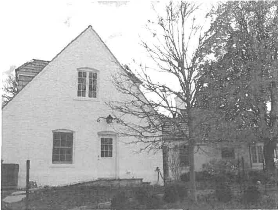
View of Addition's West Elevation and Hyphen, Facing Southeast on November 15, 2007
