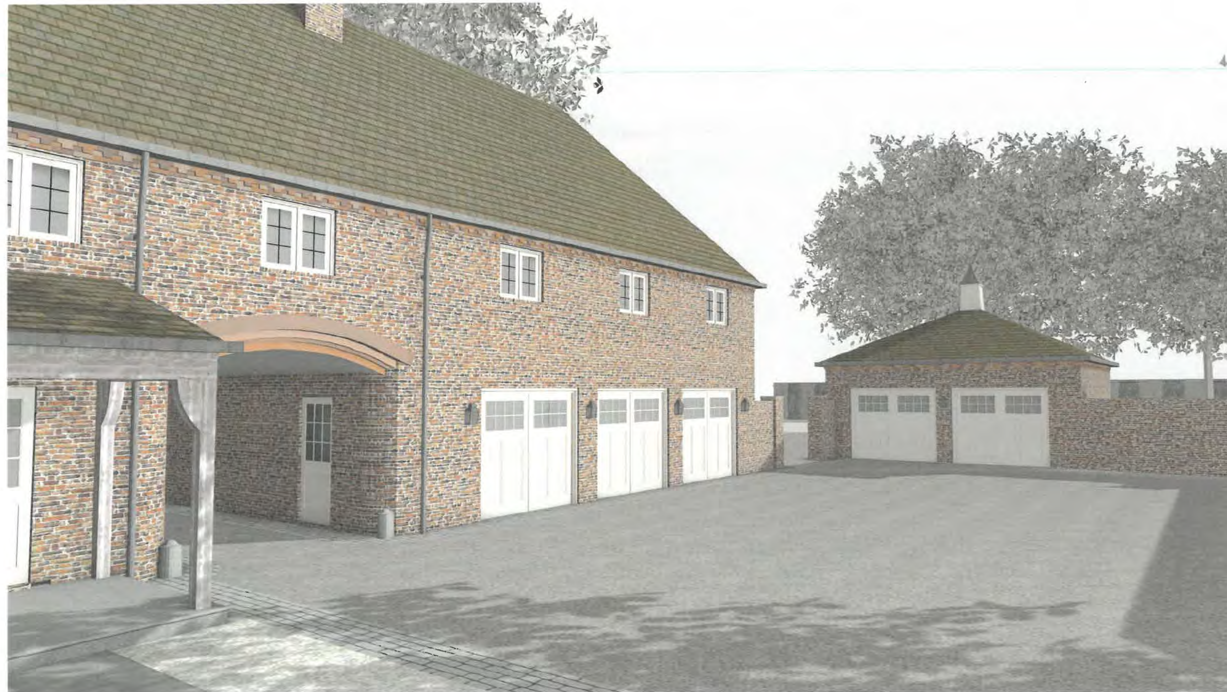
VIEW FROM THE SOUTH OF THE SERVICE COURT
