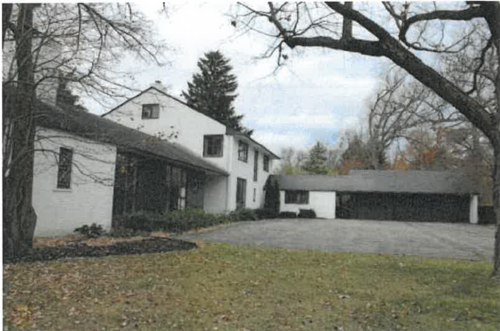
Front façade, view northwest.
