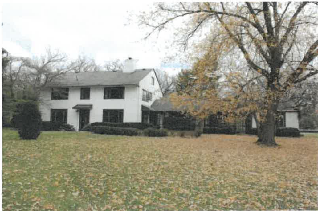
Rear façade of house, view northeast.
