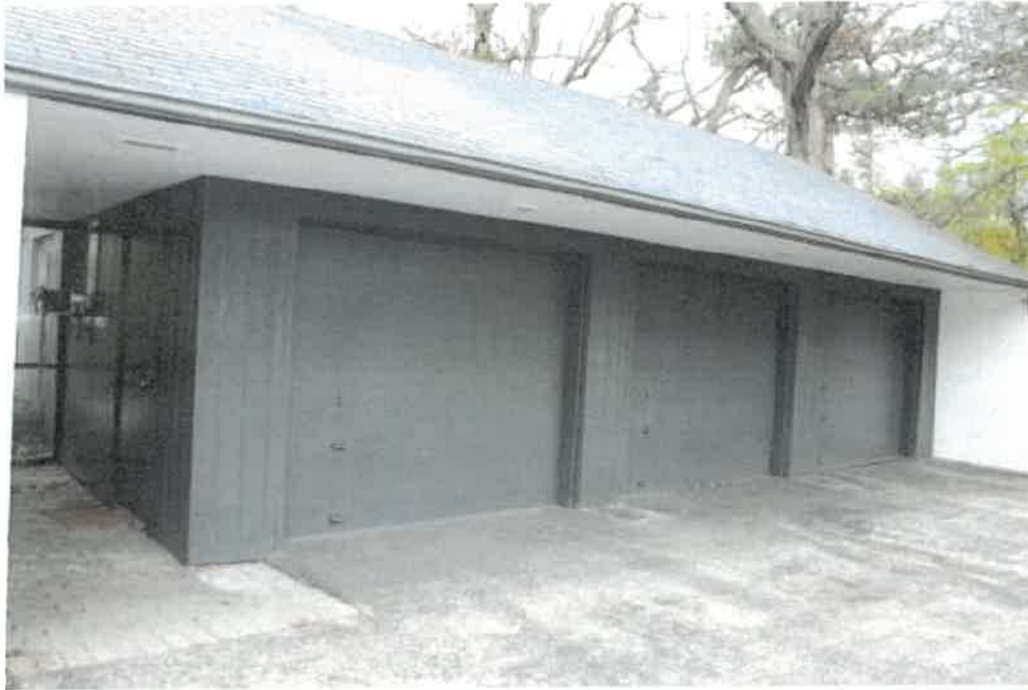
Overhead doors of attached three-car garage.
