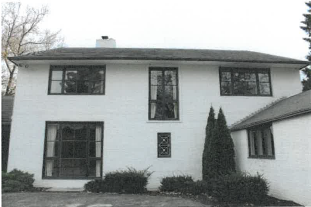
Front façade of main block, view southwest from driveway.
