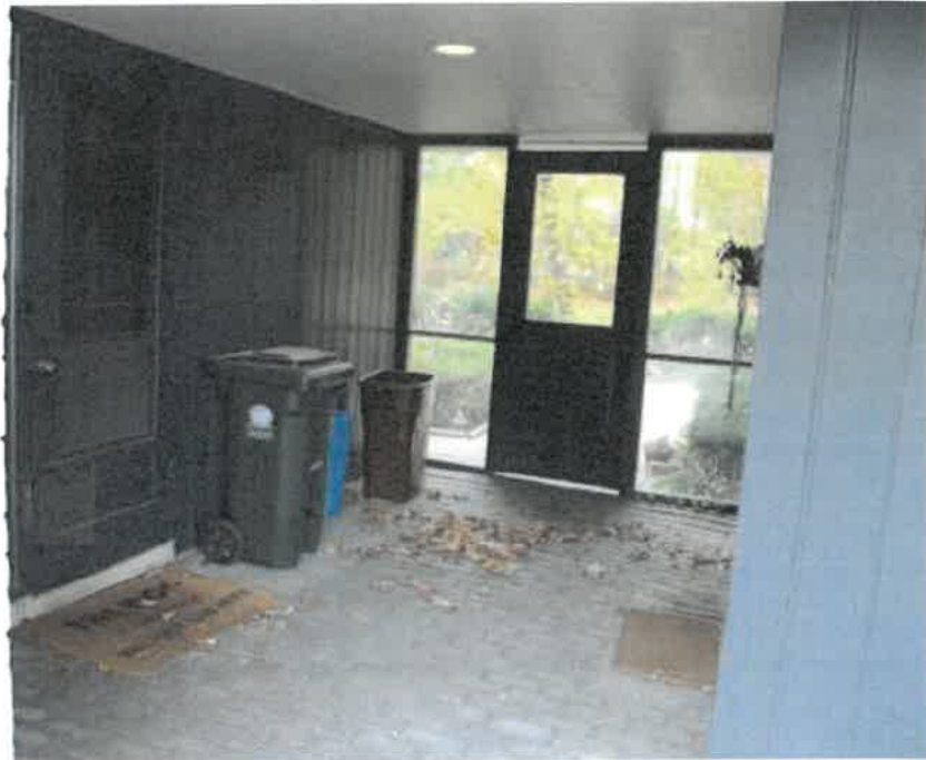
Covered breezeway between house and three-car garage with entrance to the breakfast room wing on the left.
