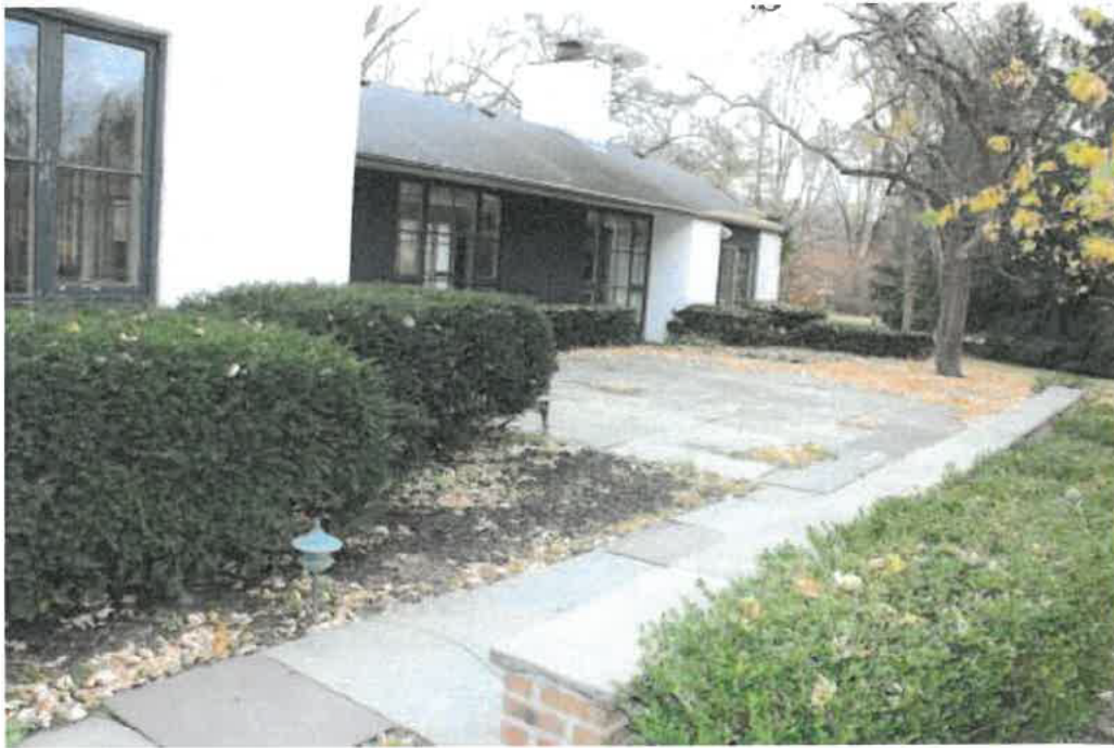
Rear façade of house, view southeast toward terrace.
