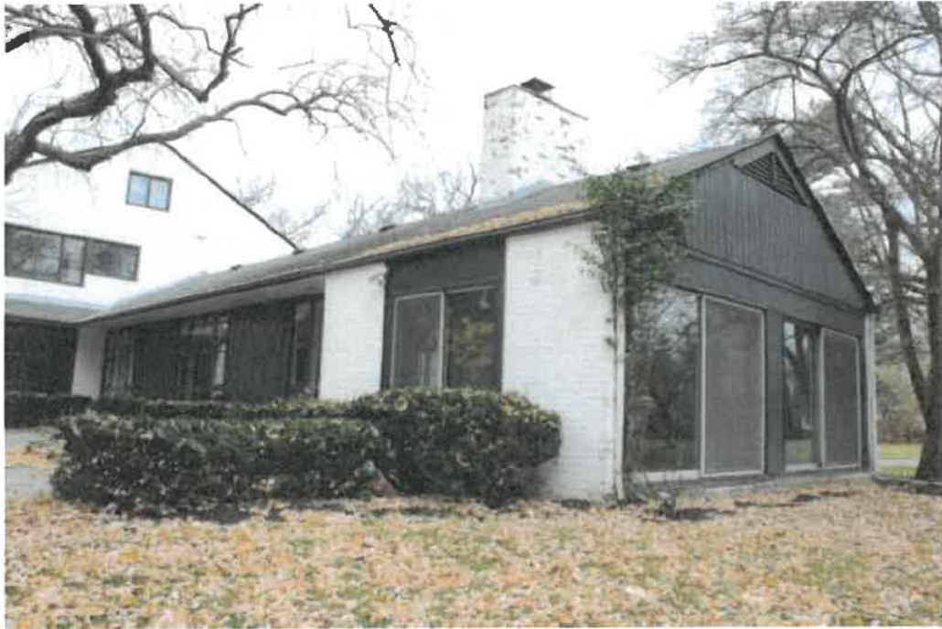
Sunporch/living room wing, view north.
