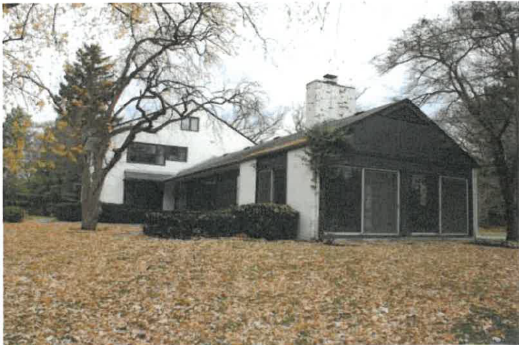
Sunporch/living room wing in foreground, view north.
