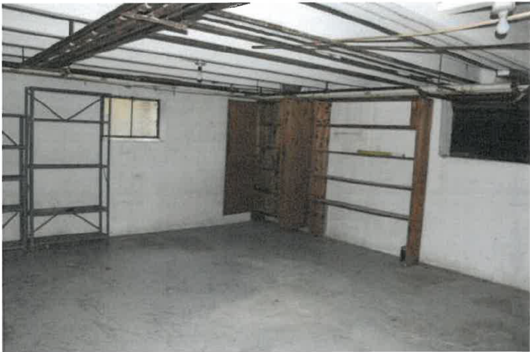
Unfinished basement storage room.
