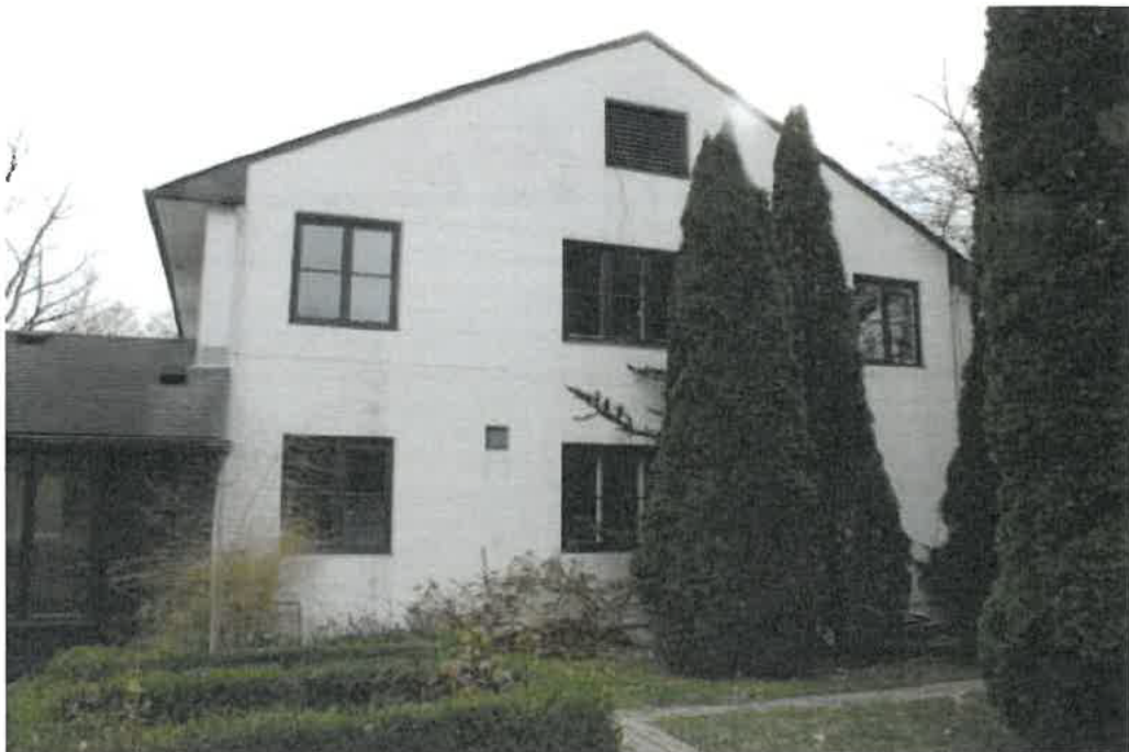
West façade of main block, view southeast.
