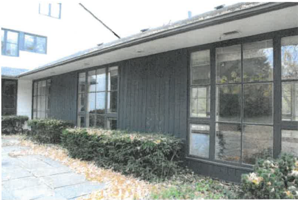
Rear façade of living room.
