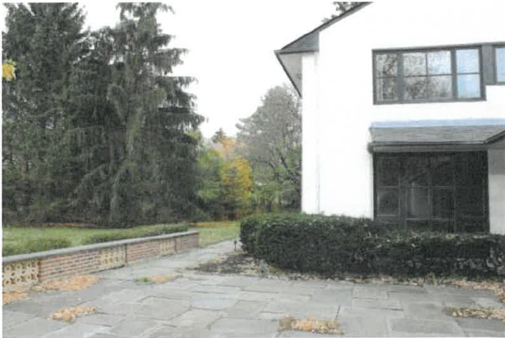
East façade of two-story main block, view northwest.
