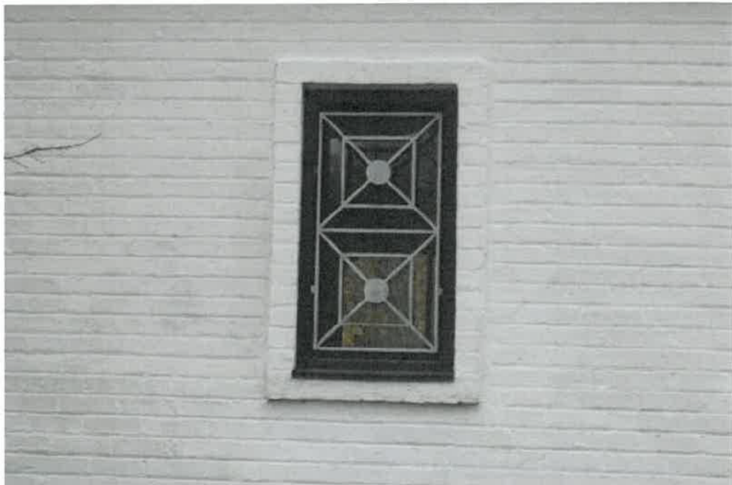
Front façade of main block, window detail.
