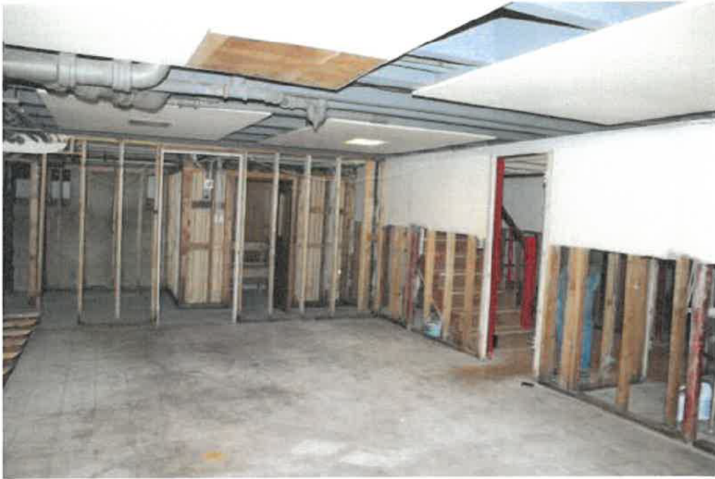
Unfinished basement storage room.
