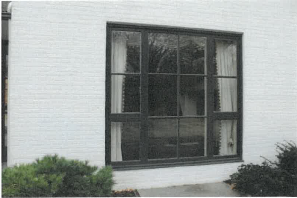
Front façade of main block, window detail.
