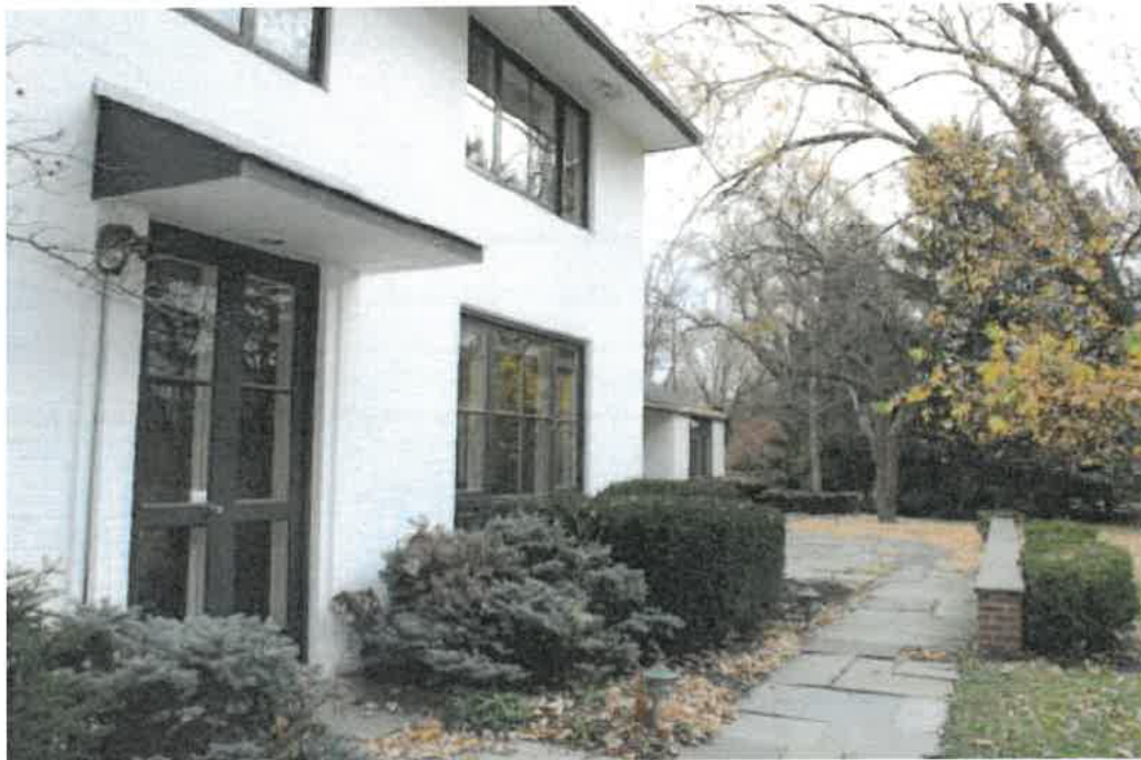
Rear façade of main block, view southeast toward terrace.
