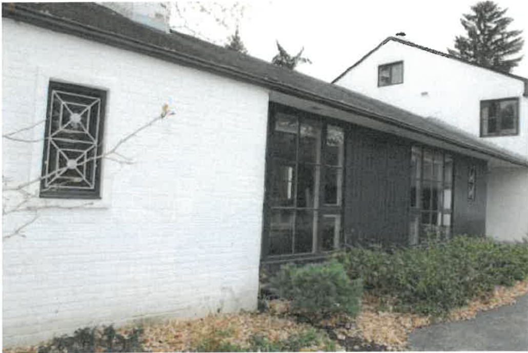
Front façade of living room, view northwest.
