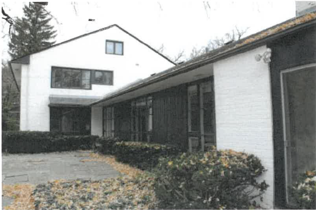
East façade of two-story main block with living room/sunporch wing in foreground.
