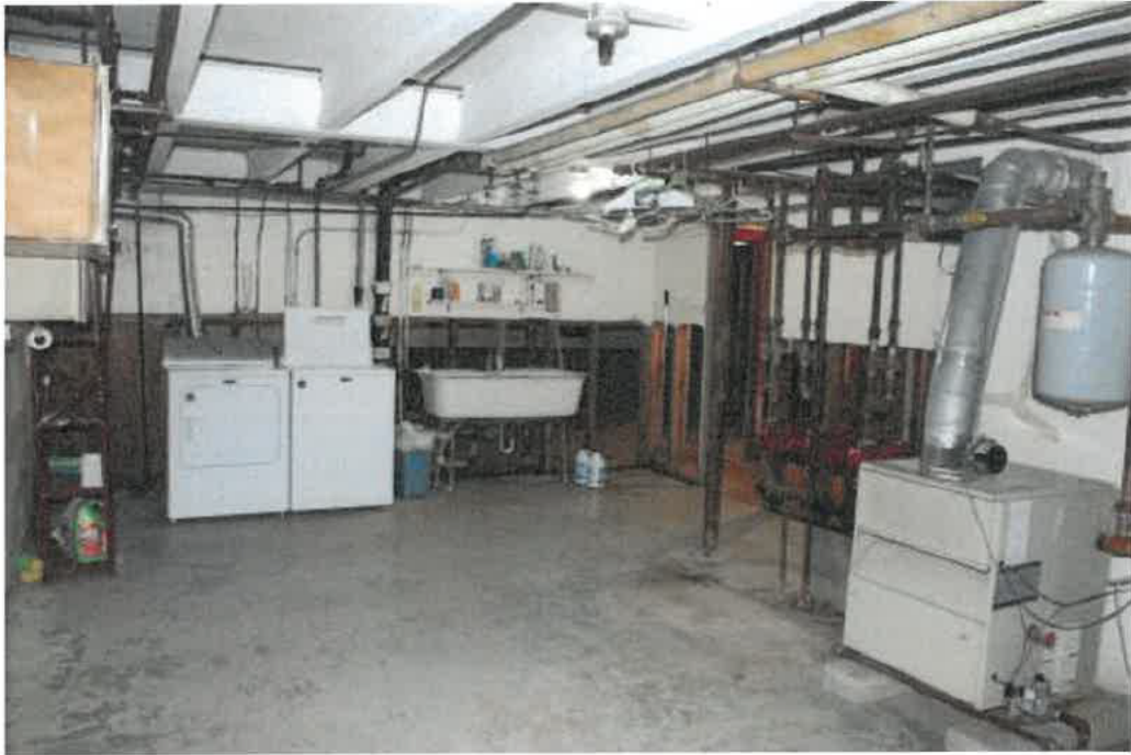
Unfinished basement laundry/mechanical room.
