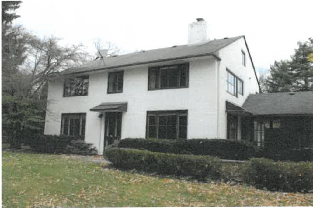
Rear façade of main block, view northeast.
