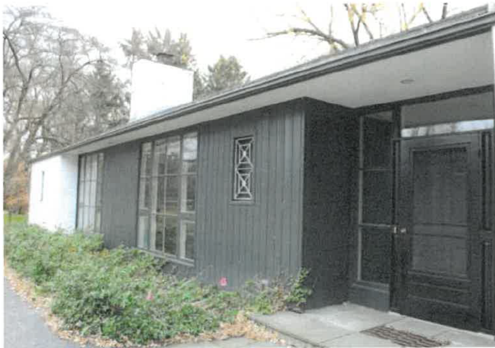
Front façade of living room/sunporch wing, showing main entrance on the right.
