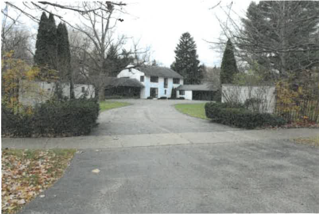
Front façade from street showing truncated brick walls flanking driveway.
