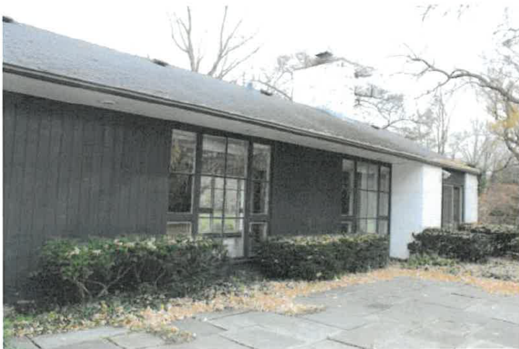
Rear façade of the living room/sunporch wing, view southeast.
