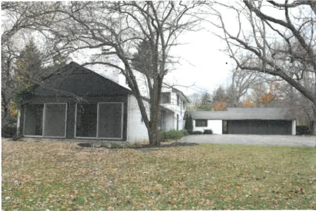
East façade of sunporch on the left, view northwest.
