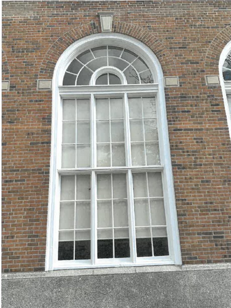
Photo 1 - View of Typical Window Type F
