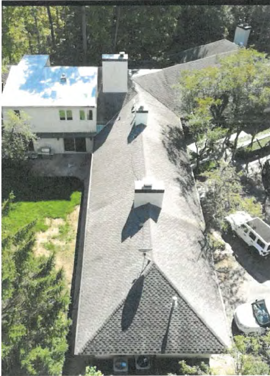
Arial View of Roof – Looking South
