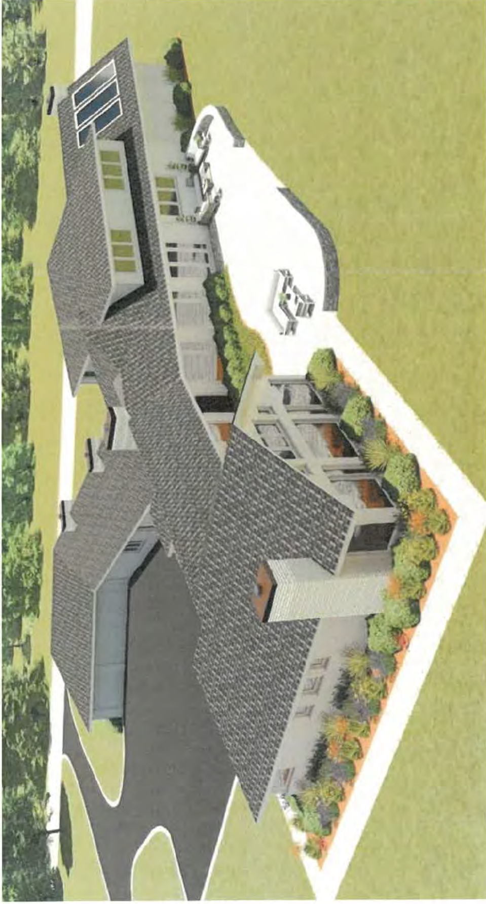
Arial View – Looking Northeast
