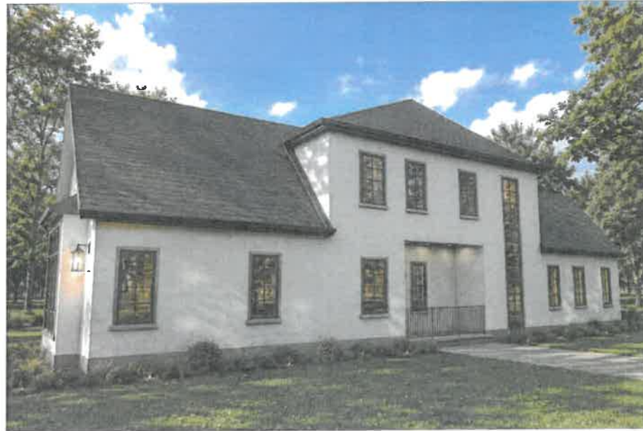
SIDE VIEW (WEST SIDE)
