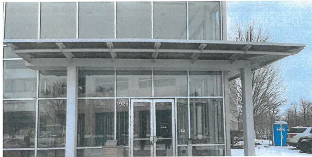
EXISTING CONDITIONS AT ENTRY CANOPY
