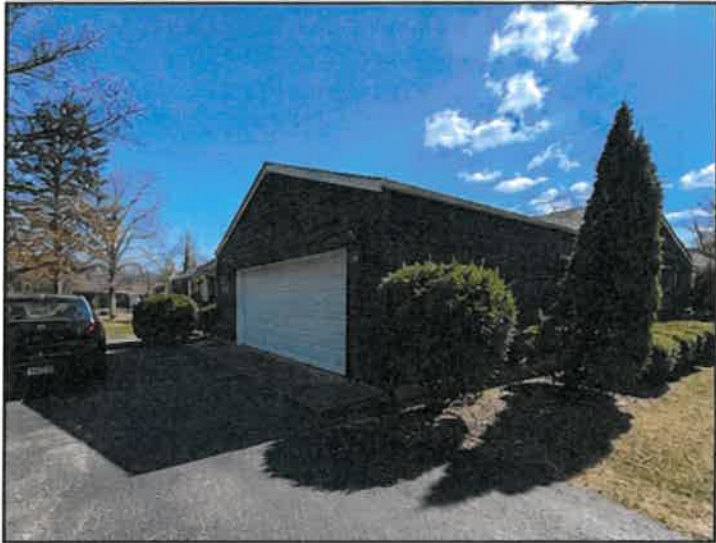
2 DRIVEWAY / GARAGE VIEW (LOOKING EAST)
