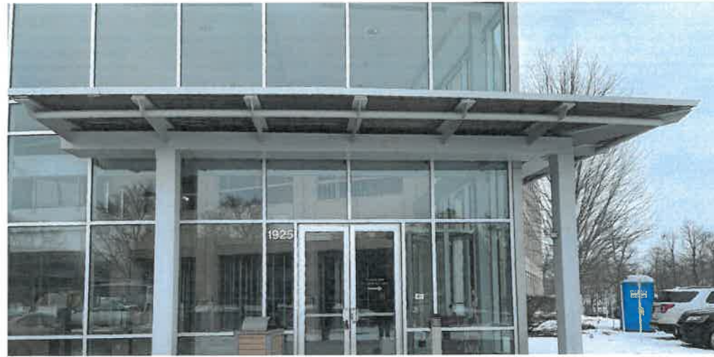
EXISTING CONDITIONS AT ENTRY CANOPY
