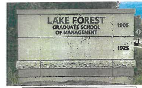
EXISTING MARQUEE - EAST ELEVATION
