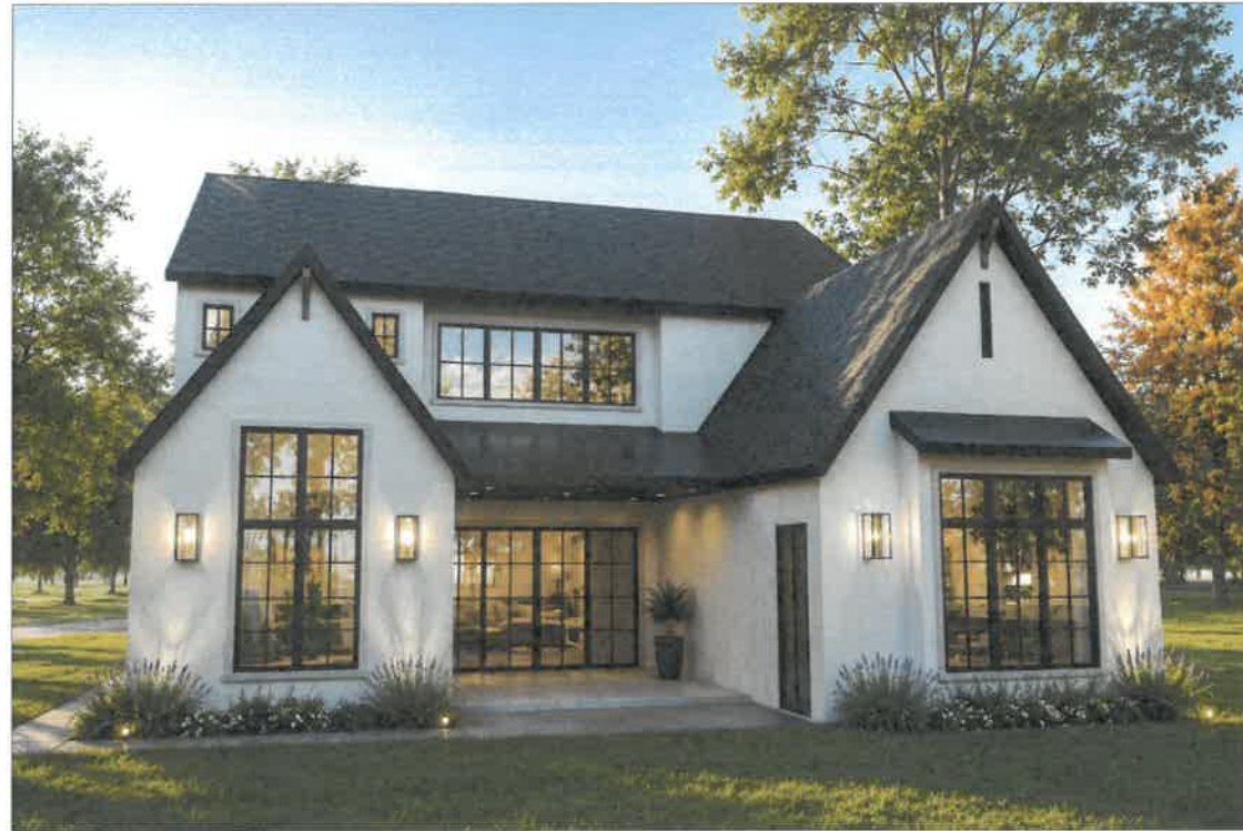
REAR VIEW (NORTH SIDE)
