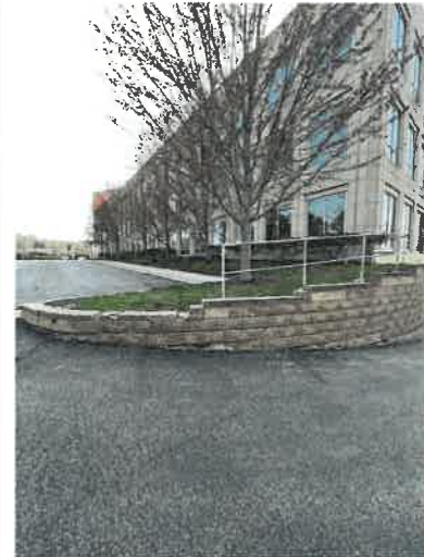
GARAGE ACCESS RAMP RETAINING WALL
