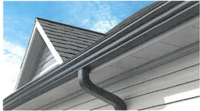
Gutter and Downspouts
