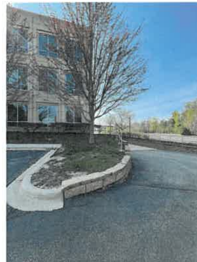
GARAGE ACCESS RAMP RETAINING WALL
