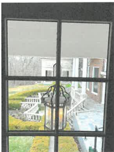
Photo 5: Looking out bedroom window at portico beam.
