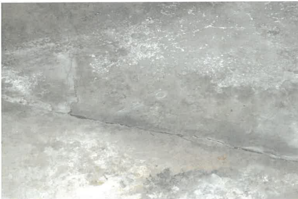
Photo No. 6 – Garage slab cracking and settlement.
