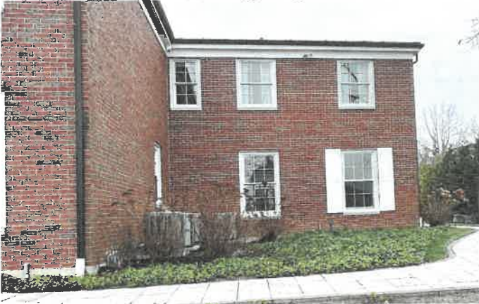
Photo 6: View of rear of garage.
