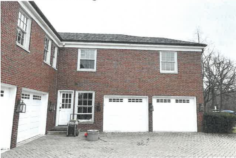
Photo 7: View of Garages
