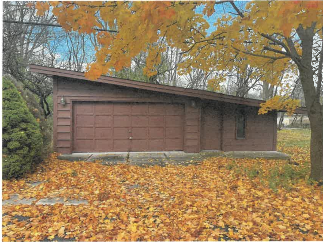
EXISTING GARAGE FROM SOUTH
