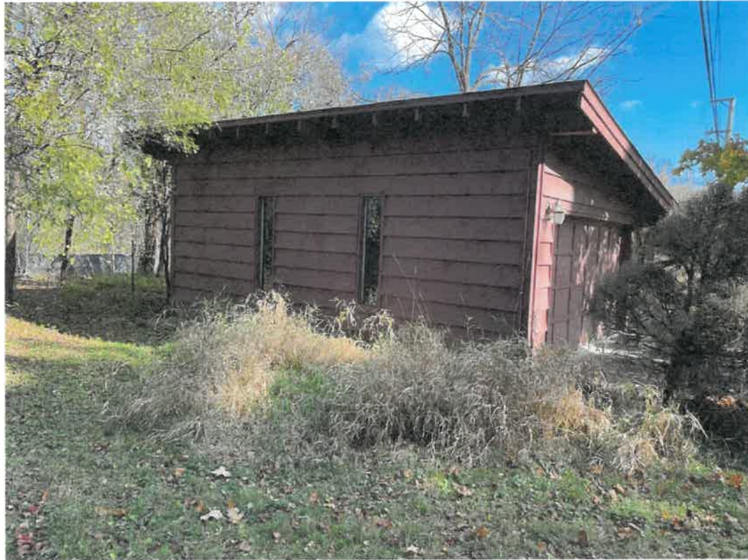
EXISTING GARAGE FROM WEST
