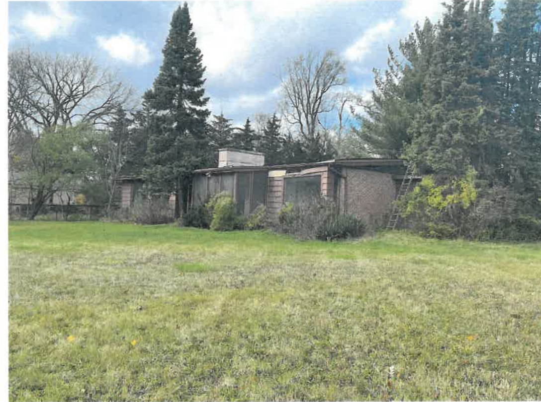
EXISTING HOUSE FROM SOUTH EAST
