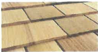
CEDAR SHAKE ROOF
