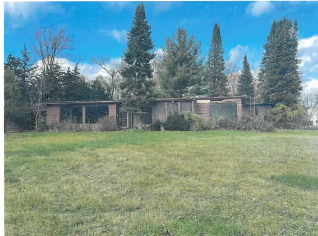
EXISTING HOUSE FROM SOUTH
