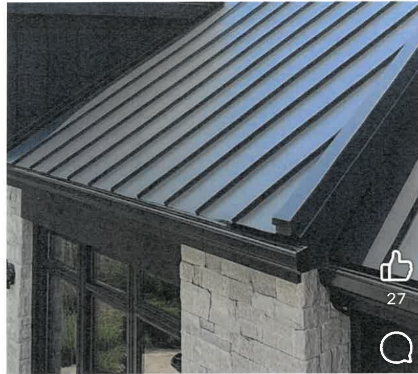
STANDING SEAM METAL ROOF
