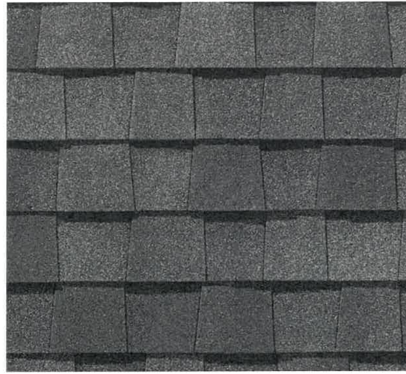
ASPHALT SHINGLE ROOFING
