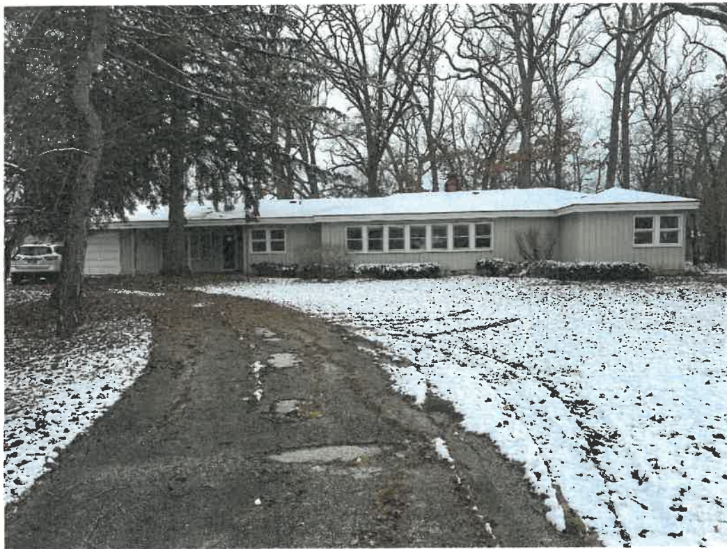
Existing Front Elevation – Southwest Elevation
