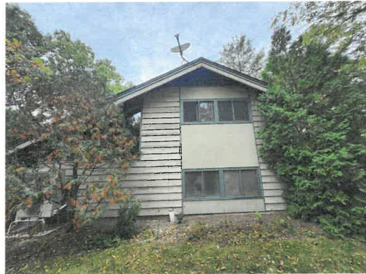
EXISTING SIDE VIEW
