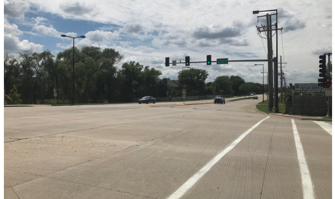
Photo of the signalized intersection of Half Day Road/Main Street/Prairie Road (view west). At its intersection with Main Street/Prairie Road, Half Day road provides two through lanes and a dedicated left-turn lane in each direction.
