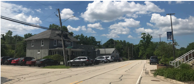
Photo of the intersection of Easton Avenue/Main Street (view north). The stairs on the far right of the photo serve as a primary pedestrian access point to the Prairie View Metra station; however, pedestrian accommodations to/from the stairs (e.g., sidewalk, crosswalk) are not provided.
