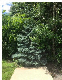
Photo of sidewalk terminus on the east side of Prairie Road north of Noah's Landing.
