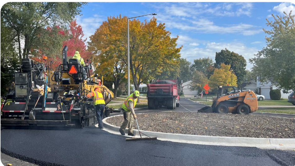
Pictured: The surface layer of asphalt pavement being layed on a section of road in the final phase of the Thompson Brandywyn Project.
