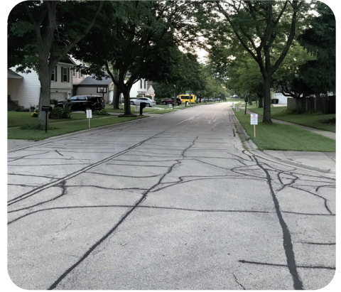
Crack Sealing
