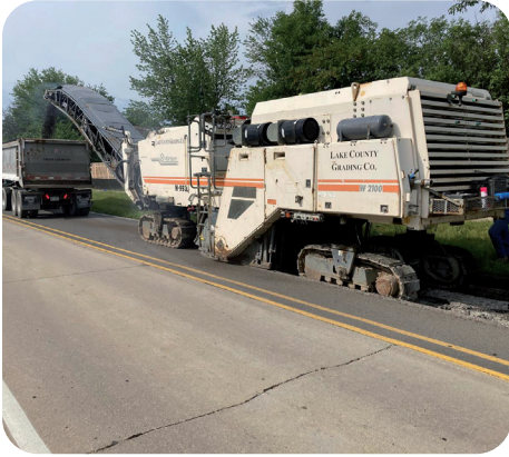
Asphalt removal grinding
