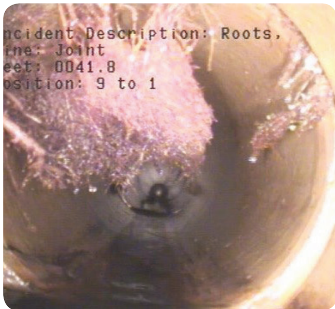
Plant Roots Inside Leaking Pipe
