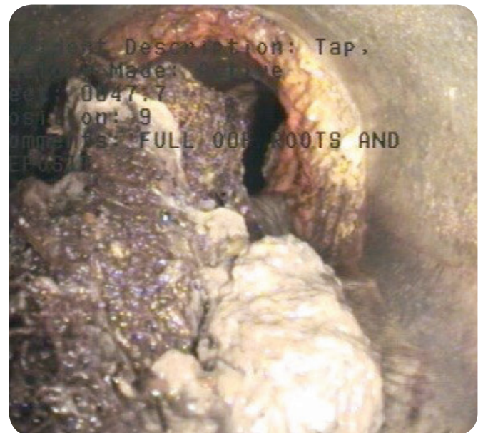
Ruptured Sewer Pipe
