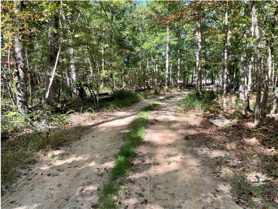
Figure 11: View northwest along proposed access & utility easement.
