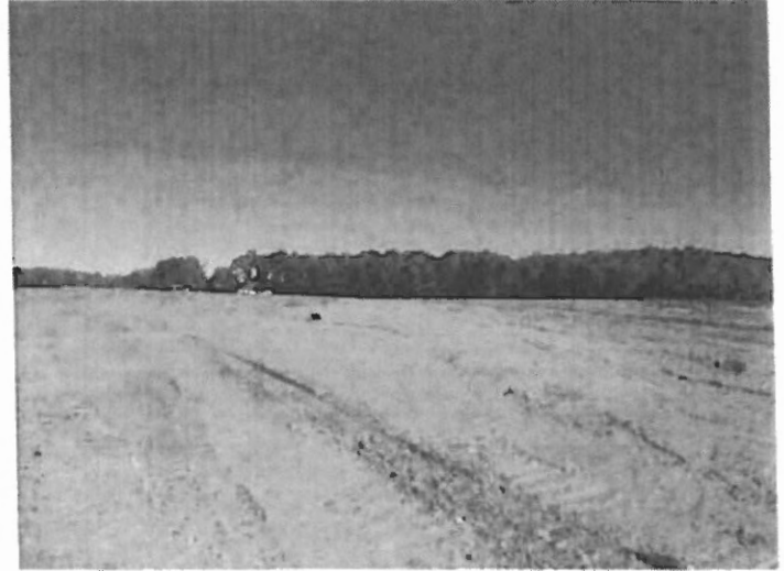
Photo 2 Area of clearing and grubbing
