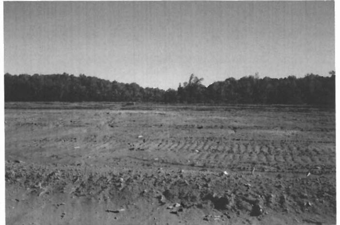
Fig. 6 Description: Evidence land disturbance occurred. No ESC measures installed or observed.
