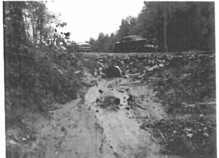
Photo 56 Recently construction stream crossing. Pipe is countersunk to an appropriate depth. Bank stabilization needed Orientation S
