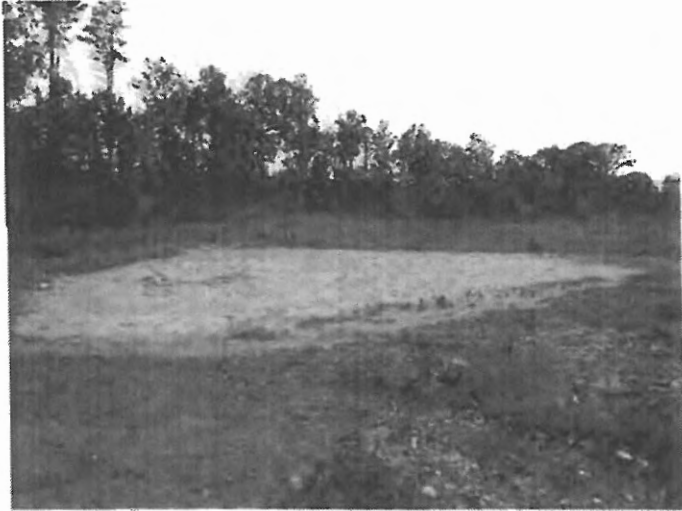
Photo 45 Constructed stormwater basin Orientation W
