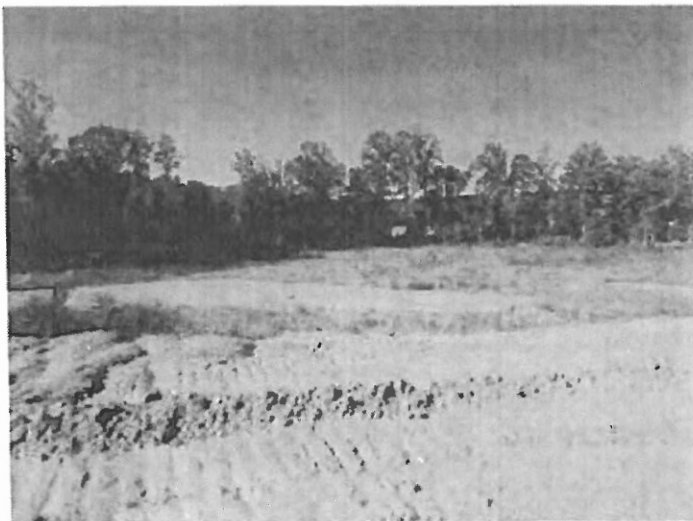
Photo 3 Area of clearing and grubbing with stormwater basin in the background
