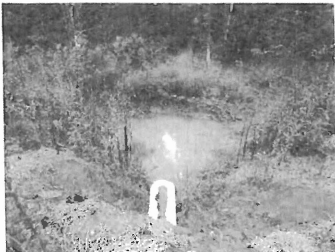
Photo 47 Constructed stormwater basin outfall Orientation S
