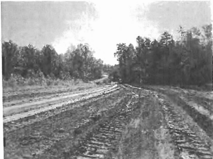
Photo 5 Area of clearing and grubbing
