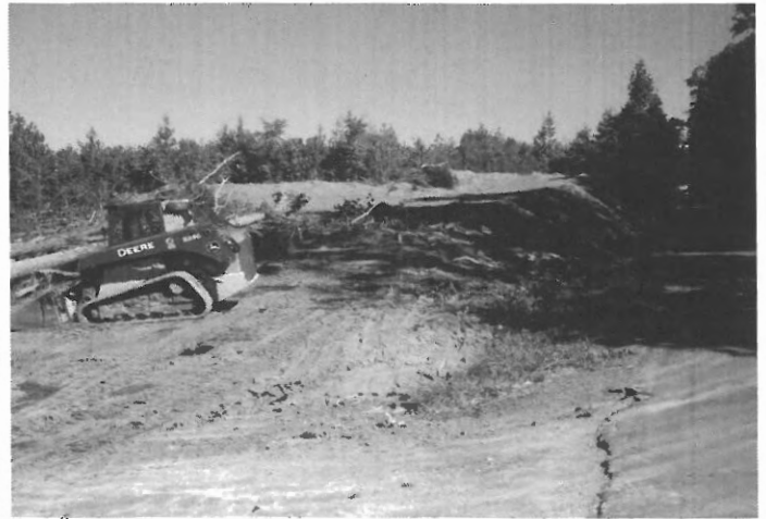
Fig. 2 Description: Area to the right side of the entrance. Trees have been cut down and area has been graded.
