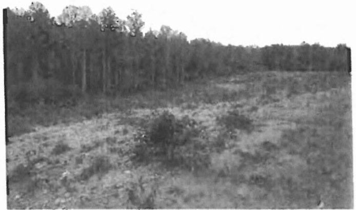
Photo 22 Area of clearing and grubbing Orientation SE
