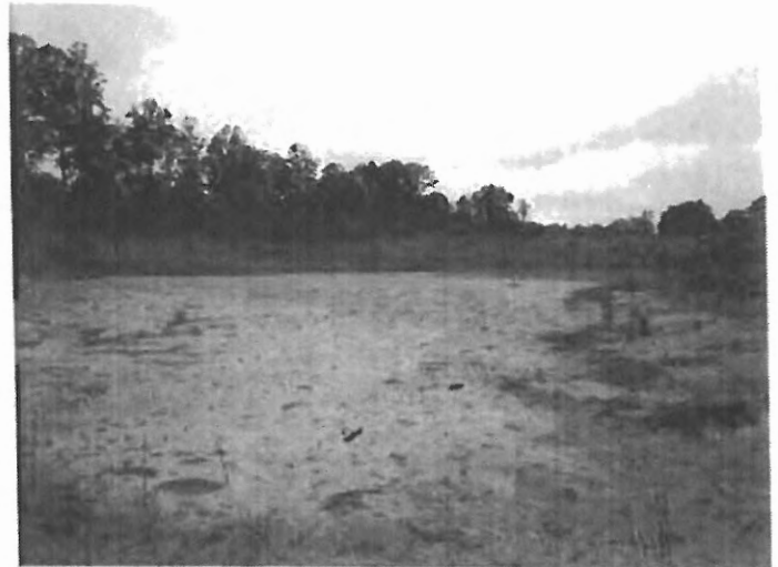
Photo 46 Constructed stormwater basin Orientation W
