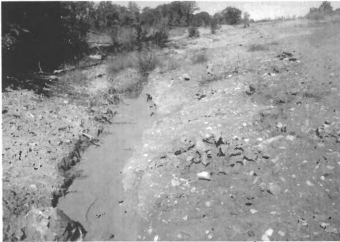
Fig. 9 Description: Evidence of land disturbance occurred. No ESC measures installed or observed.
