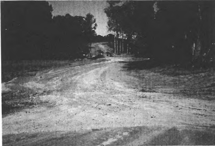
Fig. 1 Description: Site entrance.
