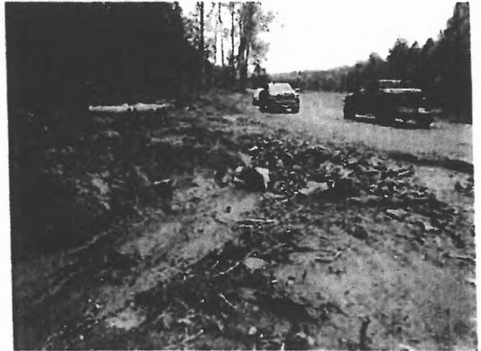
Photo 18 Stream crossing area at Dunker Creek
