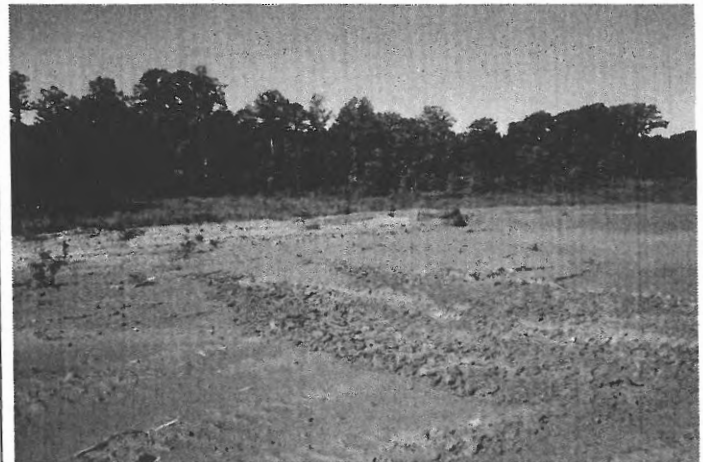
Fig. 4 Description: Evidence of Land disturbance.
