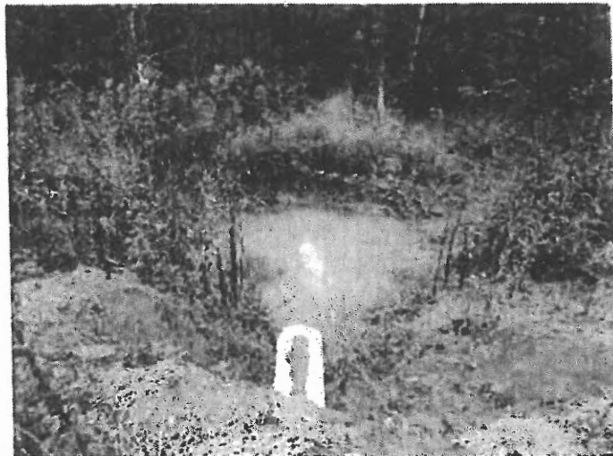
Photo 47 Constructed stormwater basin outfall Orientation S
