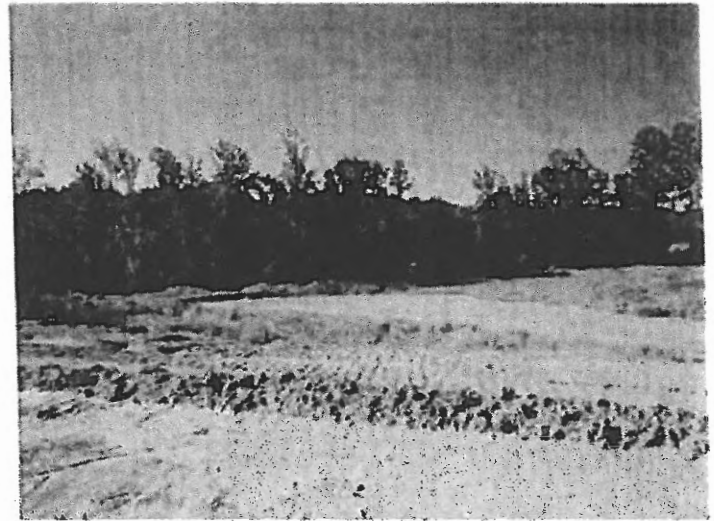
Photo 4 Area of clearing and grubbing with stormwater basin in the background
