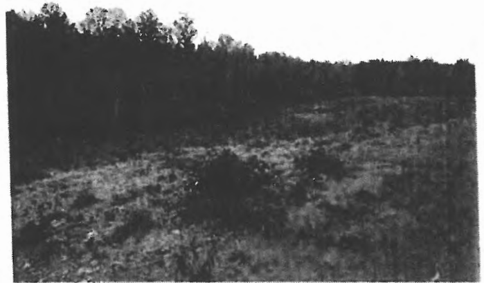
Photo 22 Area of clearing and grubbing Orientation SE
