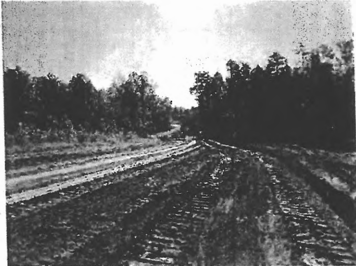
Photo 5 Area of clearing and grubbing
