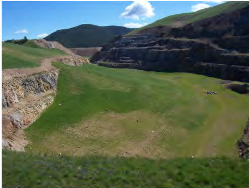
FIGURE 3-24 Highwalls remaining adjacent to backfilled, contoured, and vegetated surfaces at the Zortman-Landusky Mine, Montana.
