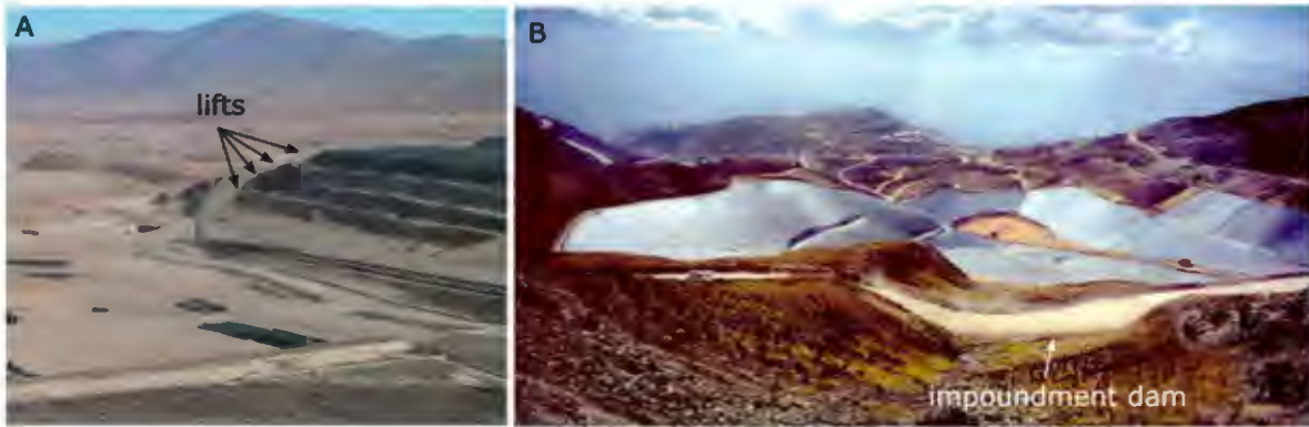
FIGURE 3-17 (A) Expanding heap-leach operation with multiple lifts. (B) Valley-fill heap leach operation, with impoundment dam toward the bottom of the image. SOURCE: Images from Bleiwas (2012).
