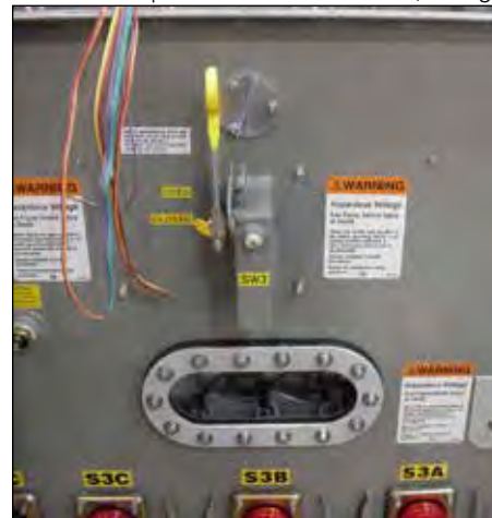
Figure 8. VFI transformer with visible break.
