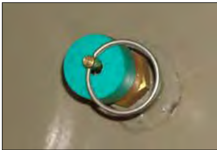
Figure 4. Automatic Pressure relief valve.
