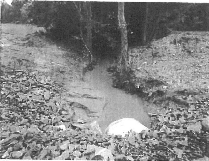
Photo 57 Dunker Creek with sediment observed. Maintenance needed. Orientation S
