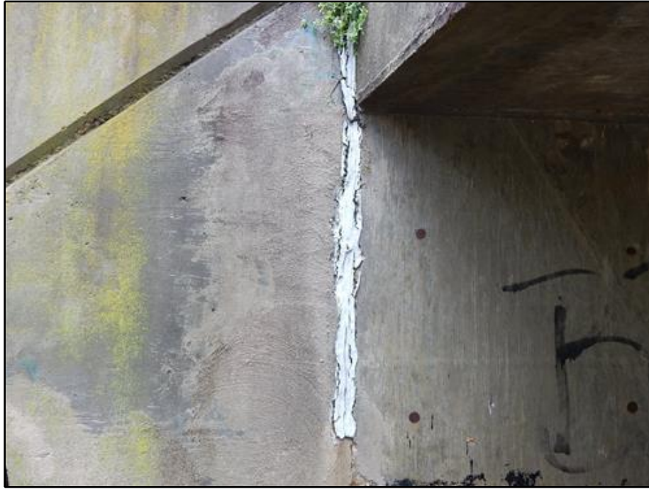
15. Wingwall - Deteriorating Joint Material between Northwest Wingwall and North Abutment
