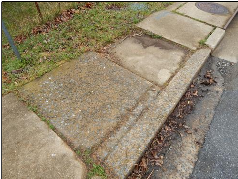
8. Sidewalk - Typical Scaling and Full-length Longitudinal Crack in Panel 2 of Northeast Sidewalk
