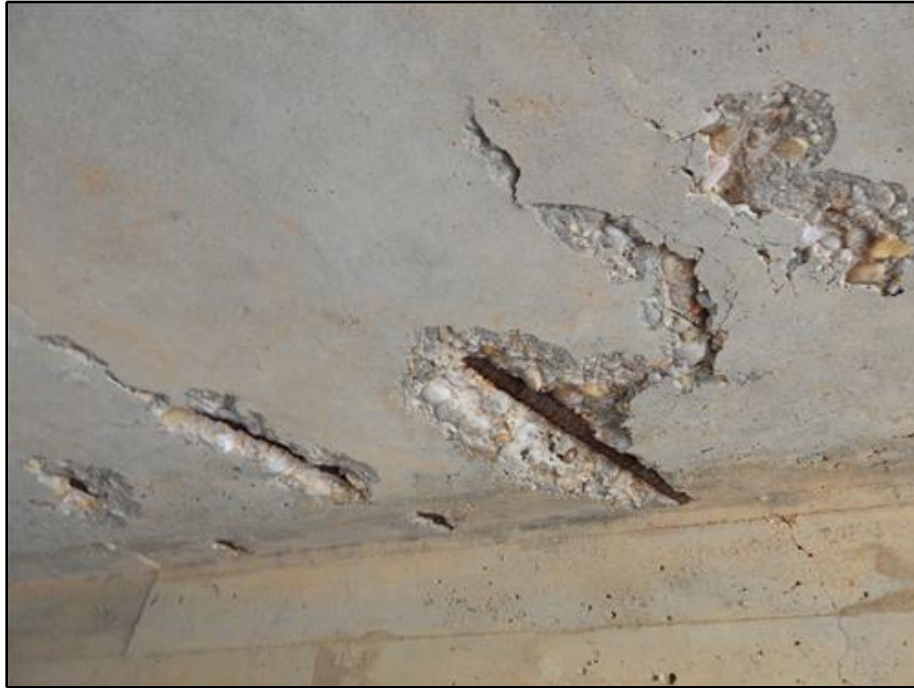
7. Deck - Adjacent Spalls with Exposed Reinforcement in Top Slab of Span 1
