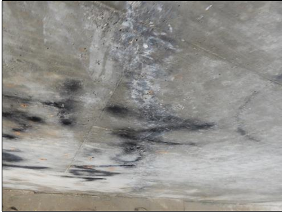
7. Deck - Full-width Longitudinal Crack with Efflorescence in Soffit
