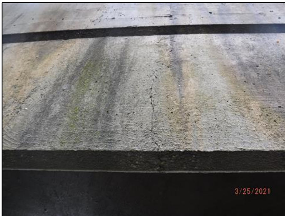
8. Cracks in South Fascia Near Midspan
