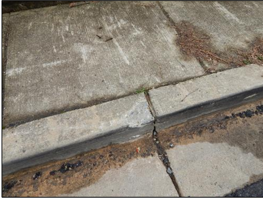
7. Curb - Spall at South Curb
