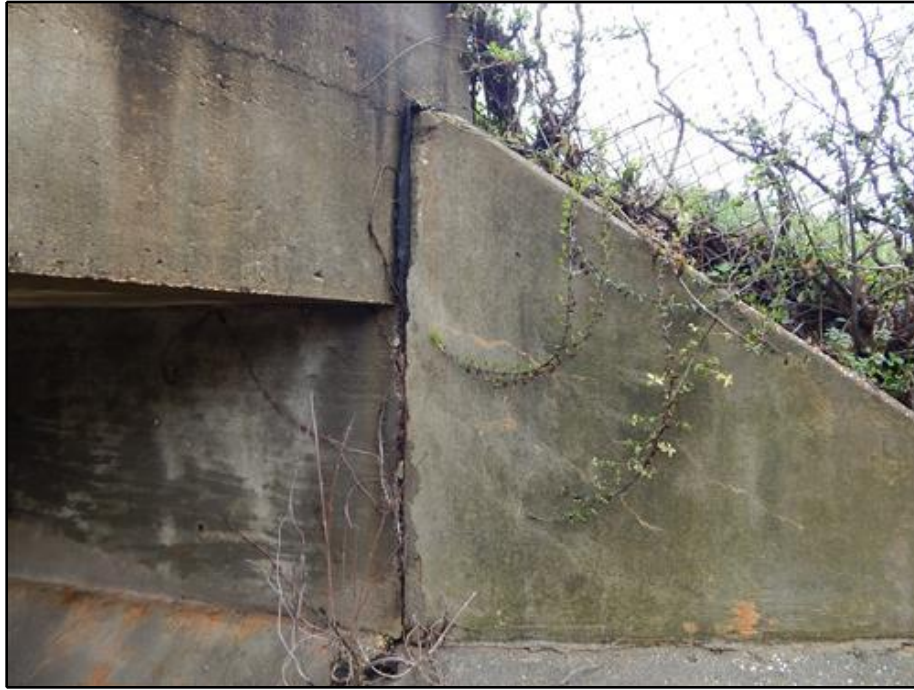
15. Wingwall - Bulging Joint at Southeast Wingwall
