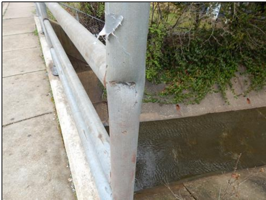
14. Railing - Dent in Post at South End of East Railing
