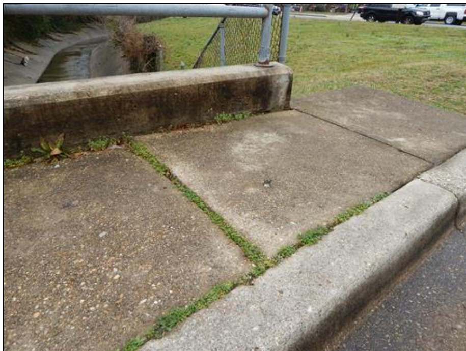
8. Sidewalk - Spall and Settlement in Panel of Northeast Sidewalk
