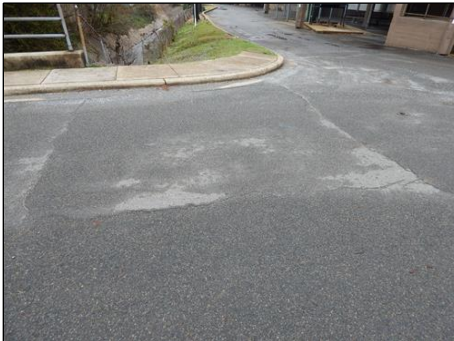
24. Approach - Longitudinal and Transverse Cracks in South Approach Pavement
