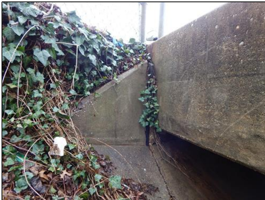
20. Wingwall - Bulging Joint Material at Southeast Wingwall
