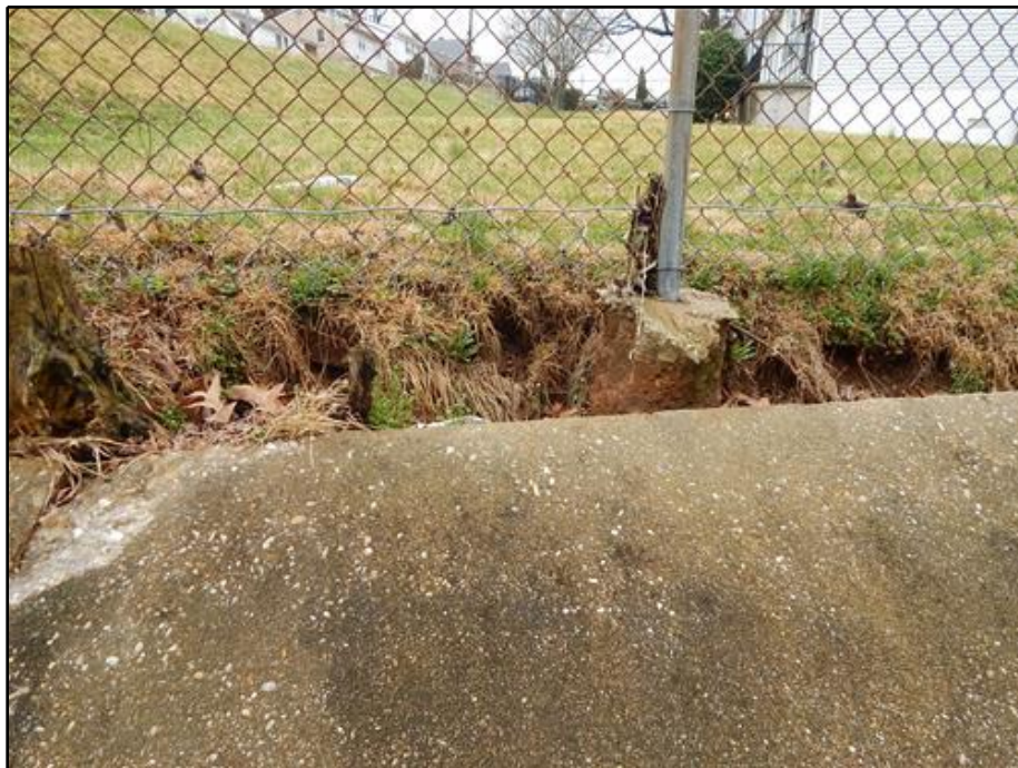
18. Fence - Exposed Fence Post Foundation at Northwest Fence
