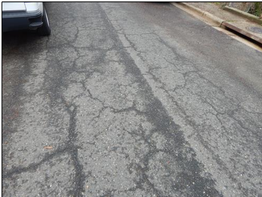
26. Approach - Map Cracking in East Approach
