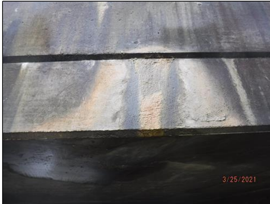
9. Water Staining on North Fascia at Midspan
