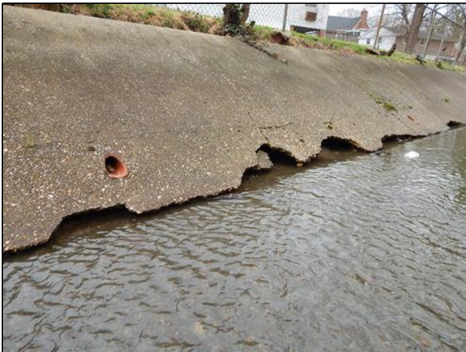
14. Slope Protection - Abrasion along Bottom of Northwest Slope Protection
