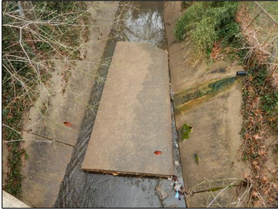
15. Slope Protection - Washed Out Southwest Slope Protection Panel
