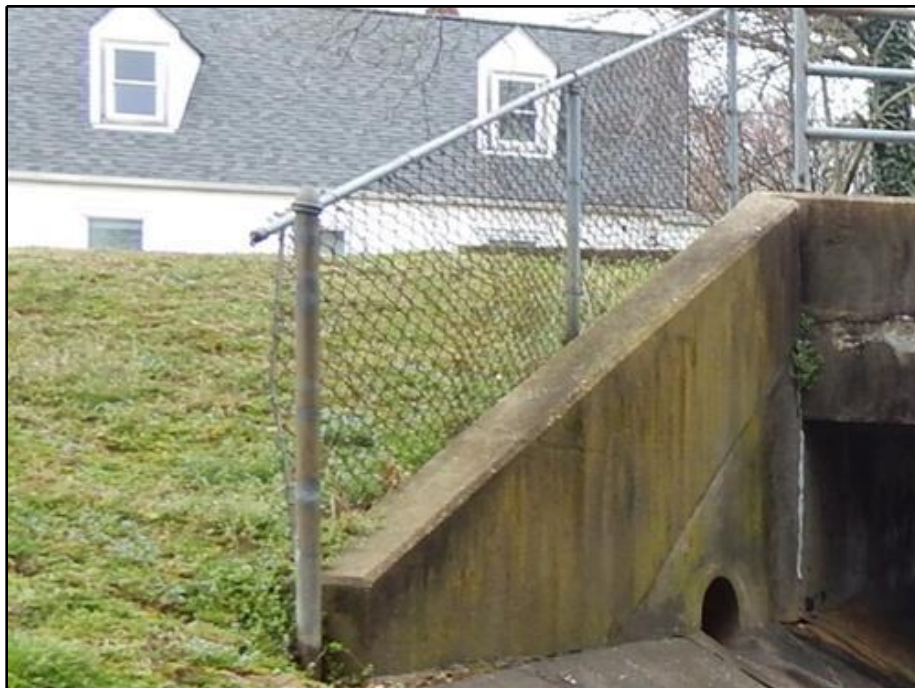
16. Wingwall - Disconnected Top Rail of Fence along the Northwest Wingwall
