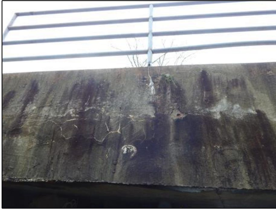
11. Parapet - Cracks with Efflorescence along Exterior Face of East Parapet
