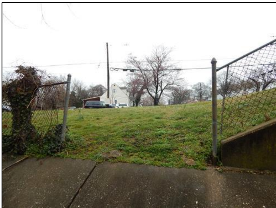
20. Fence - Missing Section of Northwest Fence
