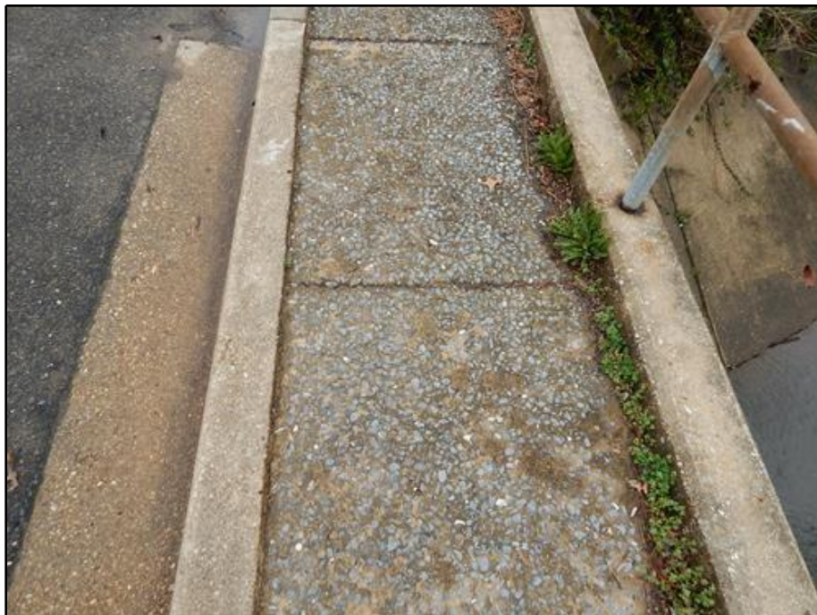
14. Sidewalk - Typical Scaling Throughout North Sidewalk
