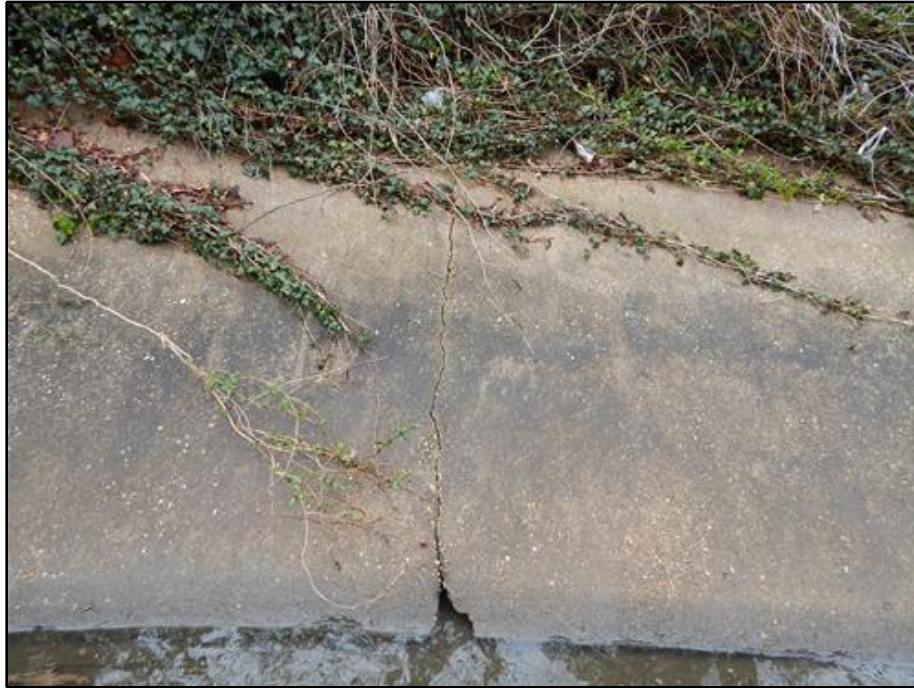
17. Slope Protection - Full-height Crack with Bottom Spall in Southeast Slope Protection
