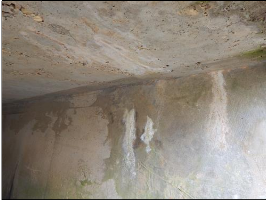
21. Pier - Vertical Cracks with Efflorescence in Pier
