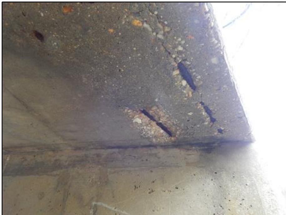
8. Deck - Adjacent Spalls with Exposed Reinforcement in Top Slab of Span 1 at the South End
