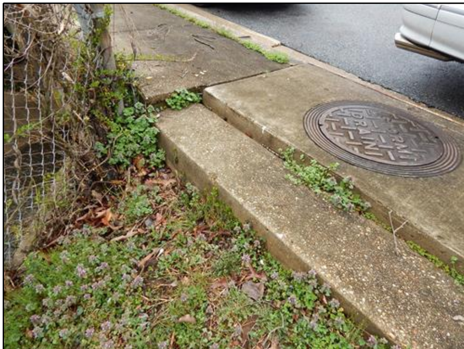
10. Sidewalk - Settlement of Southeast Sidewalk at Storm Drain Inlet
