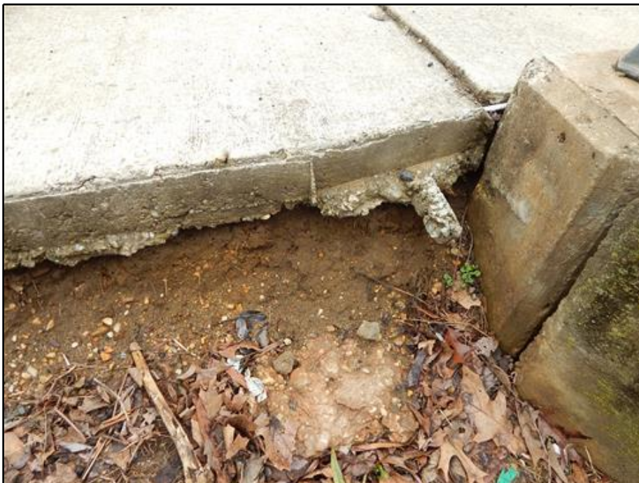
20. Sidewalk - Undermining of Northeast Sidewalk
