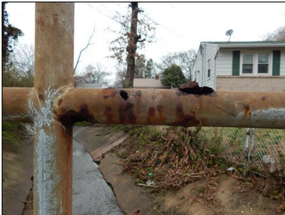
18. Railing - Corrosion Holes in North Railing Posts
