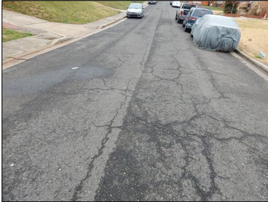
25. Approach - Map Cracking in West Approach
