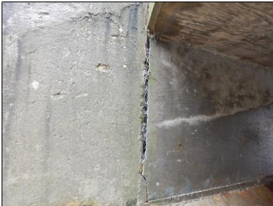
8. Wingwall - Bulging Joint Material at Northeast Wingwall
