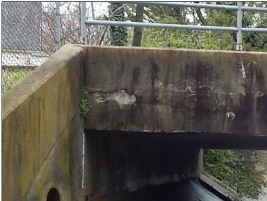
10. Parapet - Area of Failure in Coating at north End of West Parapet
