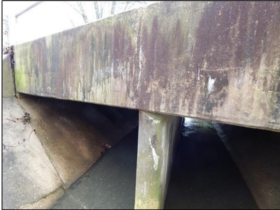
17. Parapet - Vertical Crack with Efflorescence in Exterior Face of North Parapet Extending into Pier
