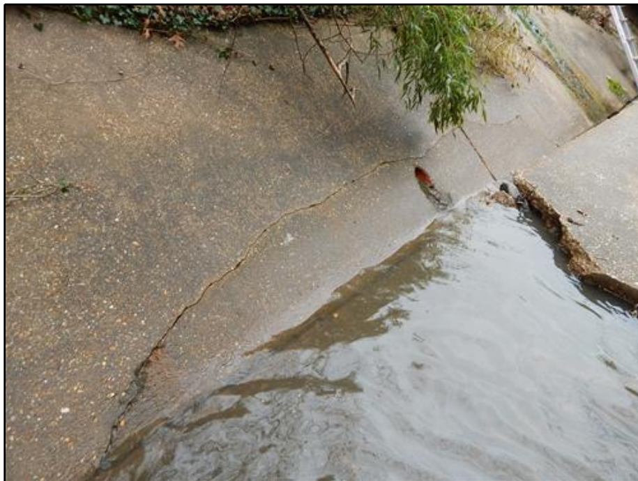
10. Slope Protection - Full-width Transverse Crack in Slope Protection Panels
