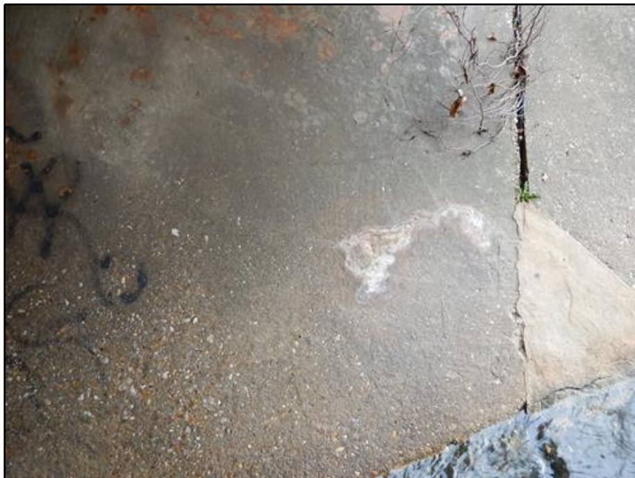
14. Abutment - Crack with Efflorescence in West Abutment
