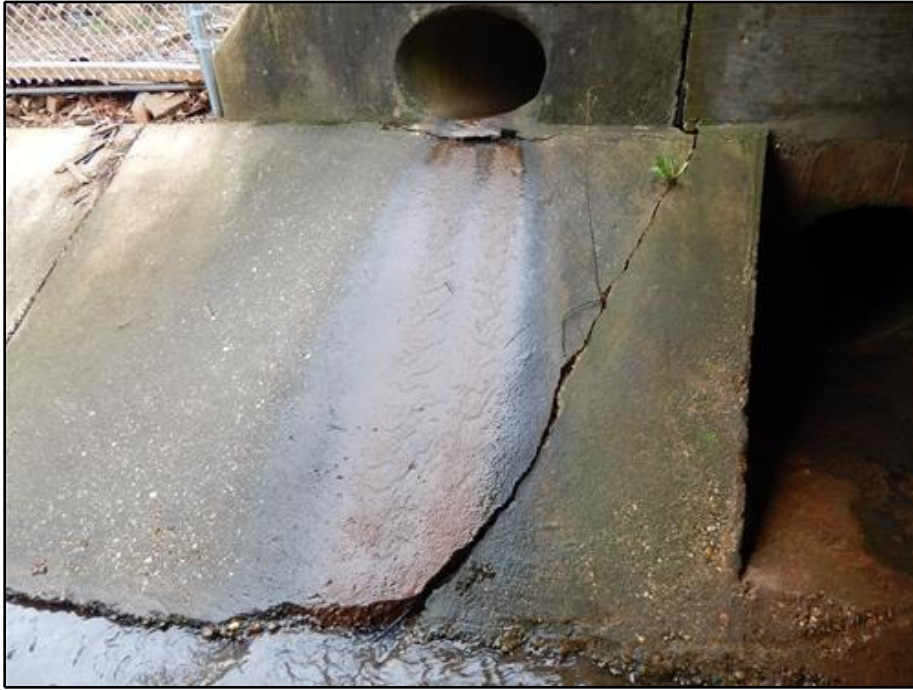
13. Slope Protection - Vertical Crack and Spall at Storm Drain Inlet in Northeast Slope Protection
