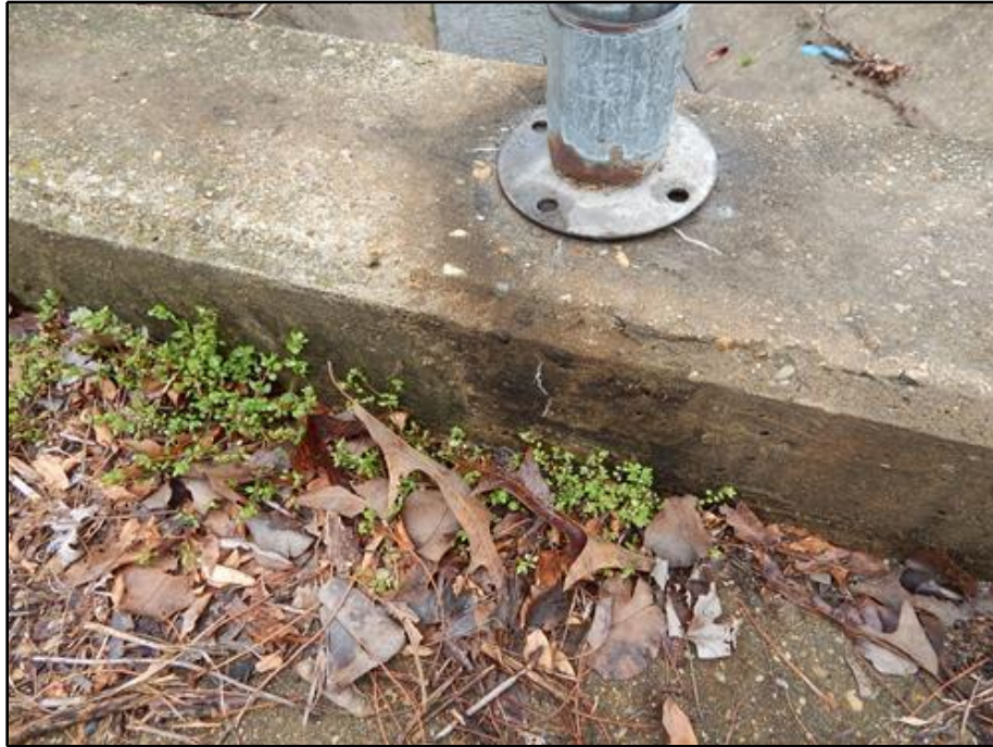
11. Railing - Typical Missing Bolts at Base of Railing Posts
