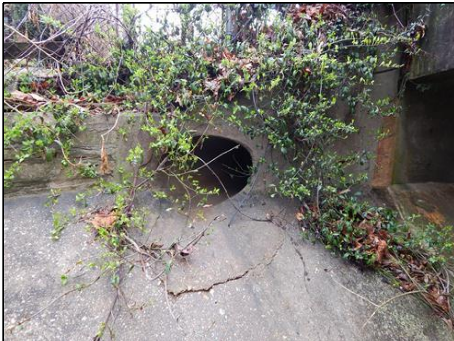
18. Slope Protection - Spall in Northeast Slope Protection Adjacent to Storm Drain Outfall
