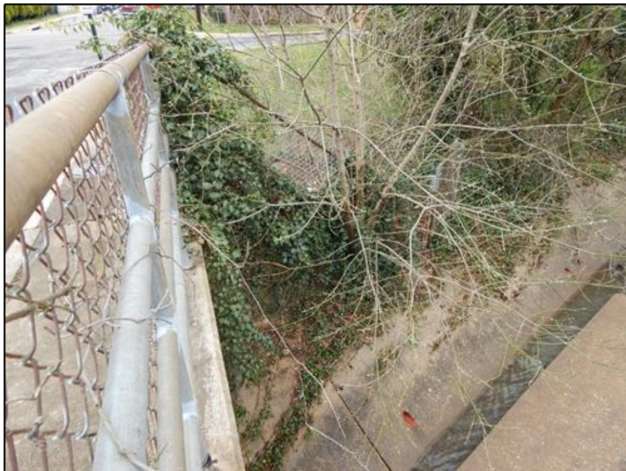
12. Slope Protection - Vegetation Growth along Southeast Slope Protection
