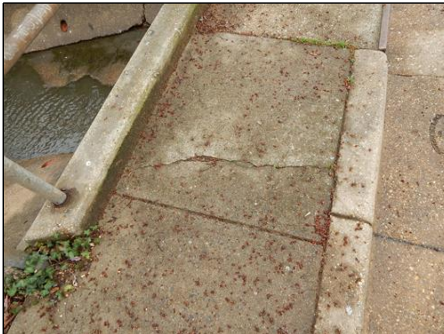
16. Sidewalk - Transverse Crack with Spall in South Sidewalk
