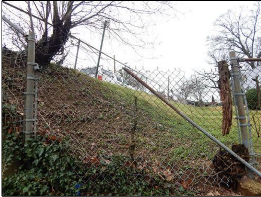
9. Fence - Missing Top Rail at Northwest Fence
