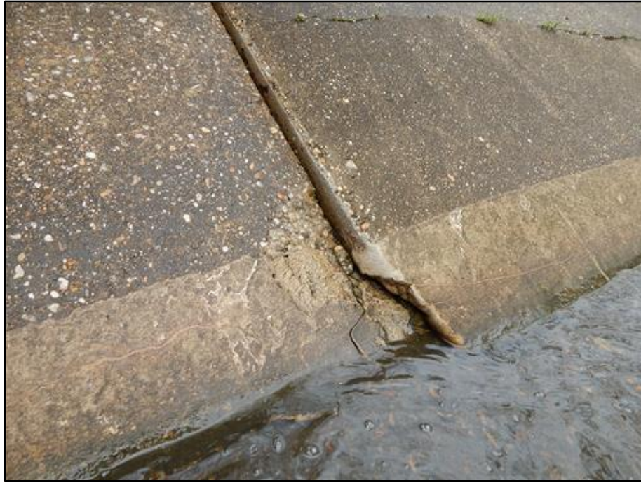
11. Slope Protection - Differential Settlement Between Northwest Slope Protection Panels
