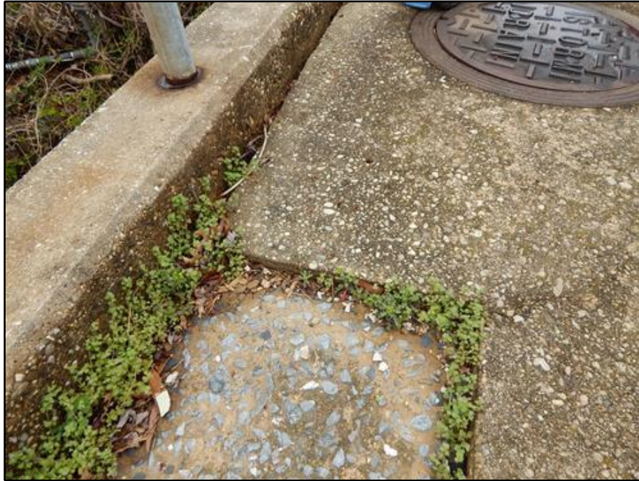
15. Sidewalk - Settlement at the South Sidewalk at Storm Drain Inlet
