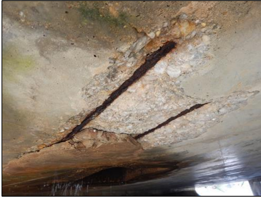
9. Deck - Adjacent Spalls with Exposed Reinforcement in the Top Slab of Span 2 at the North End
