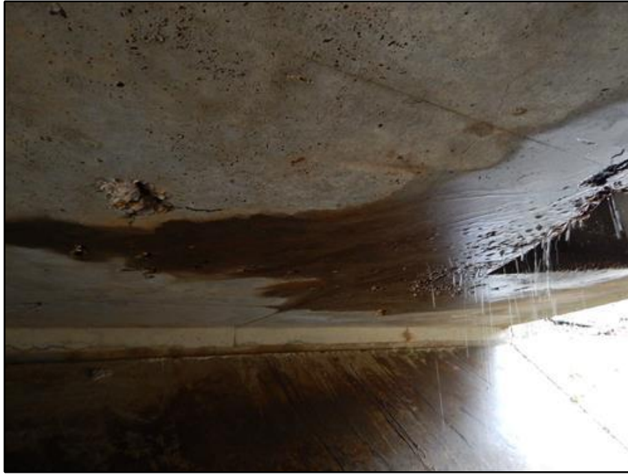
11. Deck - Spall with Exposed Reinforcement in Top Slab of Span 2 10' from North End
