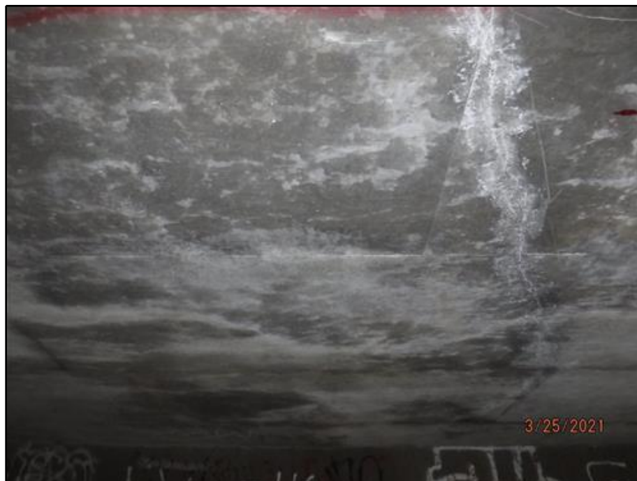
10. Typical Cracking and Efflorescence in Underside of Slab
