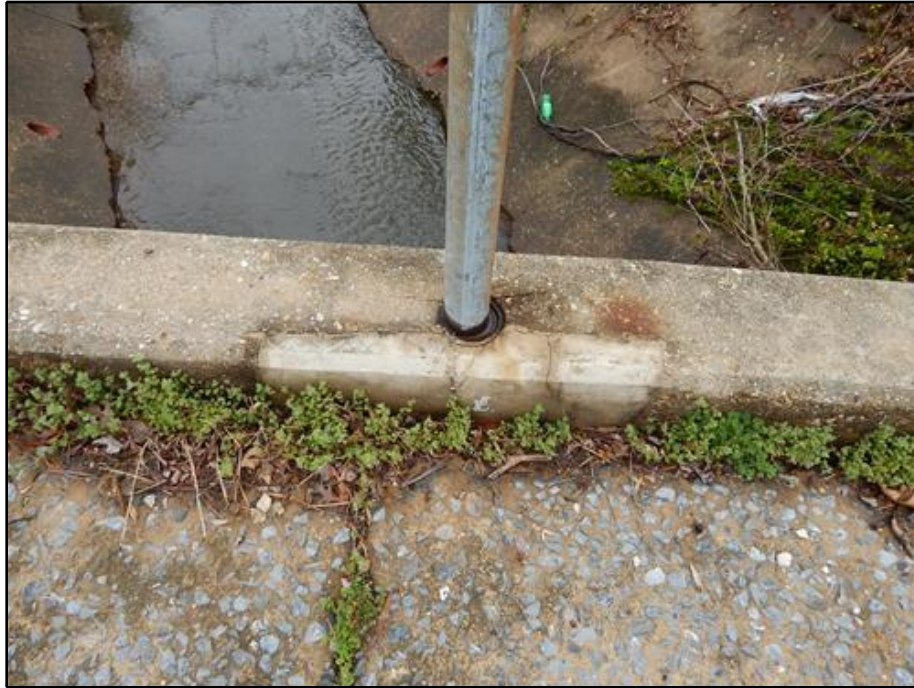
19. Railing - Cracks at Base of Railing concrete Repair
