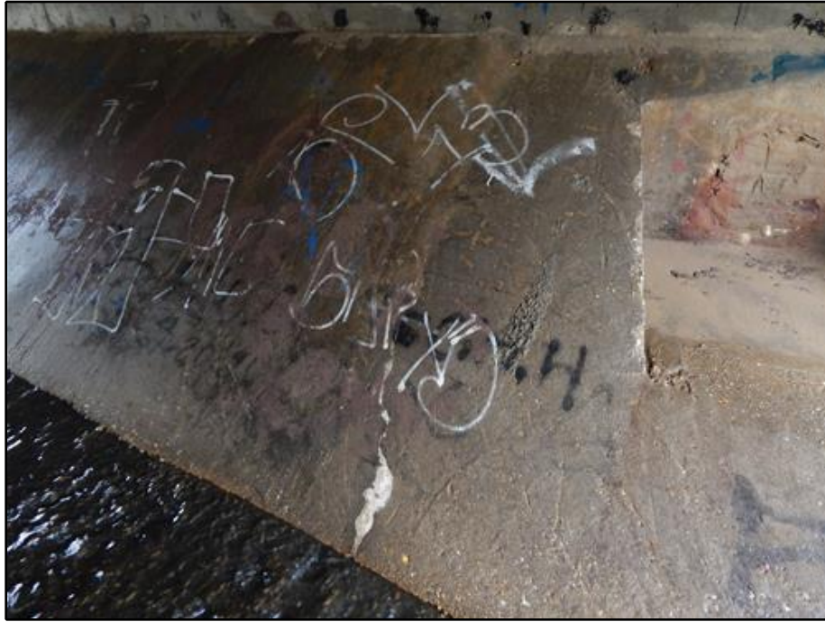
17. Slope Protection - Vertical Crack with Efflorescence at East End of North Slope Protection
