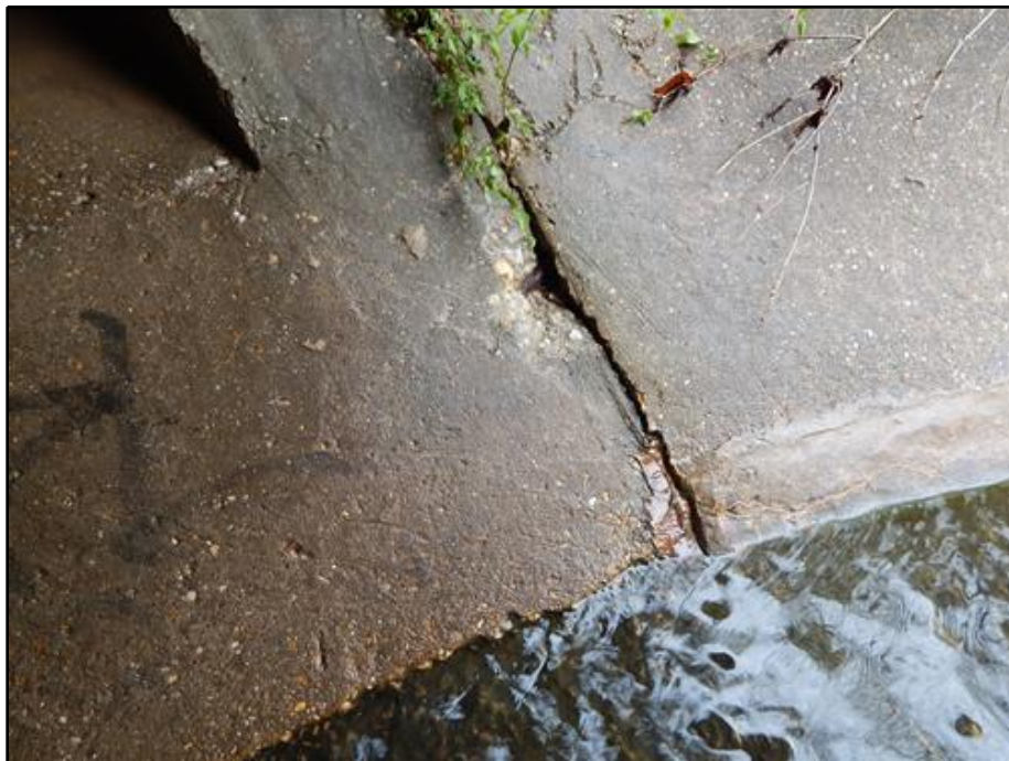
18. Slope Protection - Spall with Exposed reinforcement in North Slope Protection at East End
