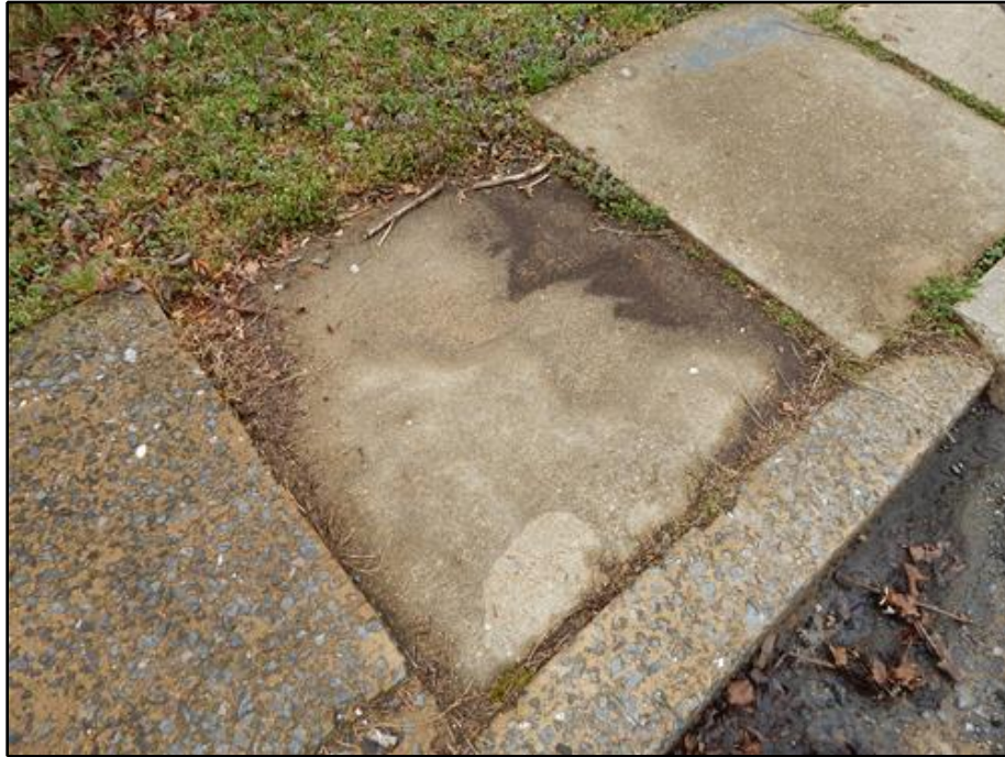
9. Sidewalk - Differential Settlement Between Panels in Northeast Sidewalk
