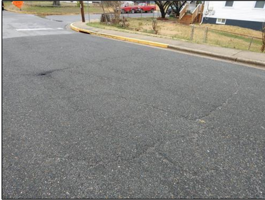
23. Approach - Map Cracking Throughout North Approach Pavement
