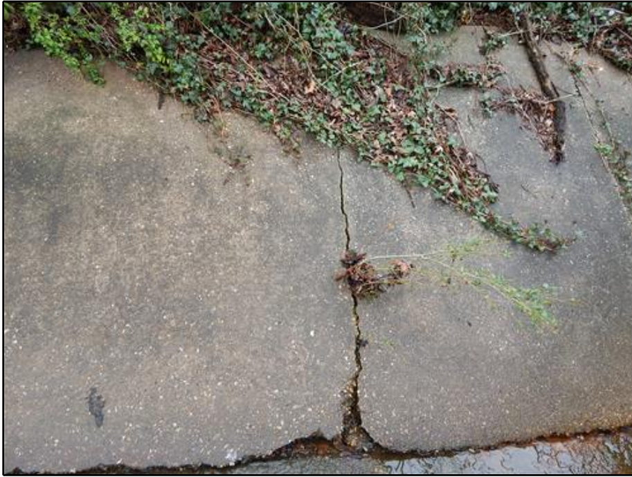
23. Slope Protection - Vertical Failure in Southwest Slope Protection
