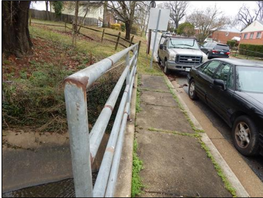
13. Railing - South Railing Leaning to the South
