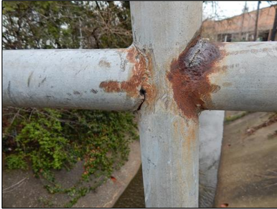
13. Railing - Typical Cracked Welds in East and West Railing
