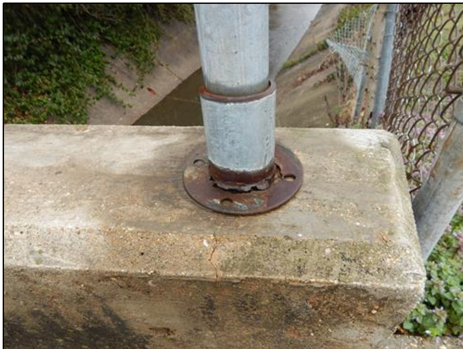
12. Railing - Typical Missing Anchor Bolts at Base of Railing Posts and Section Loss at Base of Post 4 of East Railing
