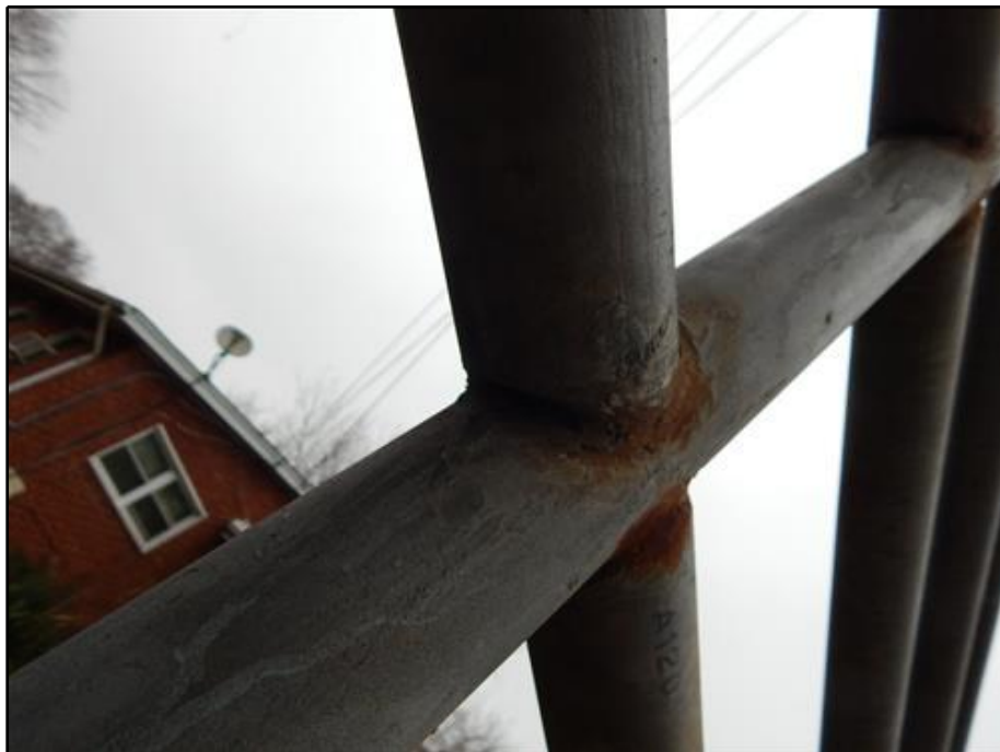
12. Railing - Cracked Weld at Bottom Rail Connection of North Railing
