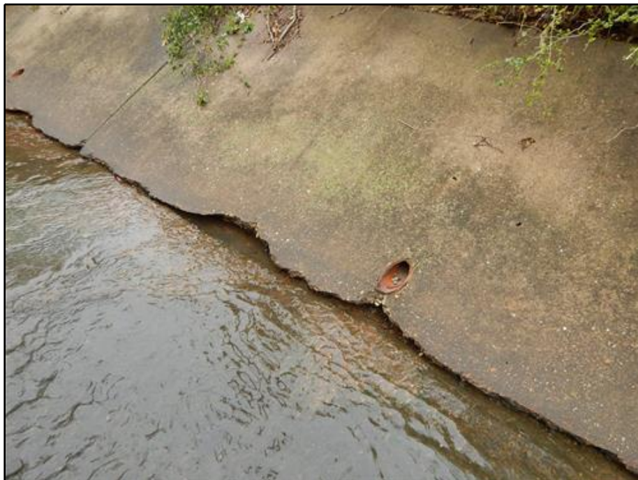
22. Slope Protection - Abrasion and Spalling along the Base of Northeast Slope Protection
