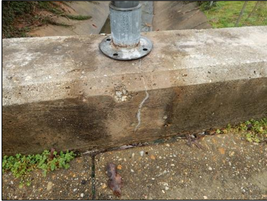
9. Railing - Vertical Crack with Efflorescence in Interior Face of West Parapet
