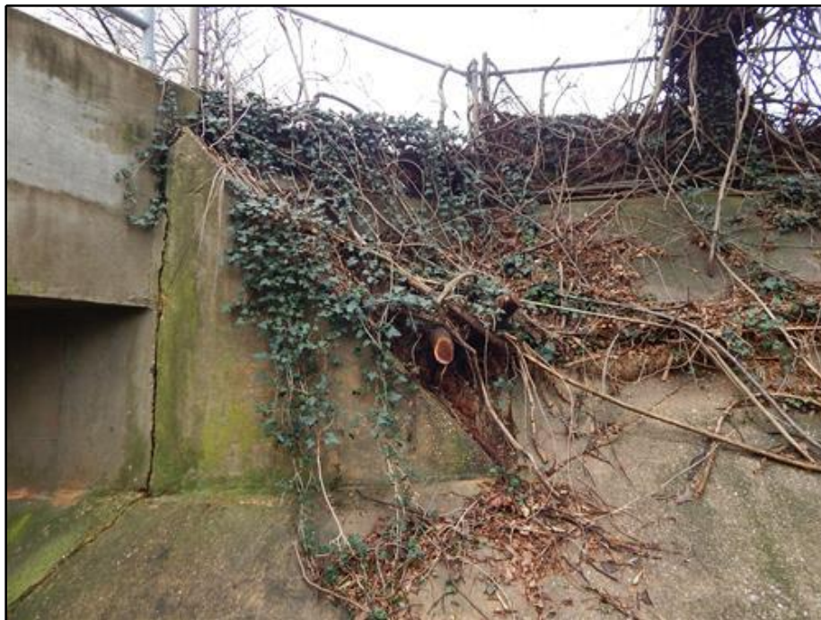
16. Slope Protection - Fractured Northwest Slope Protection Due to Tree Growing Through Concrete
