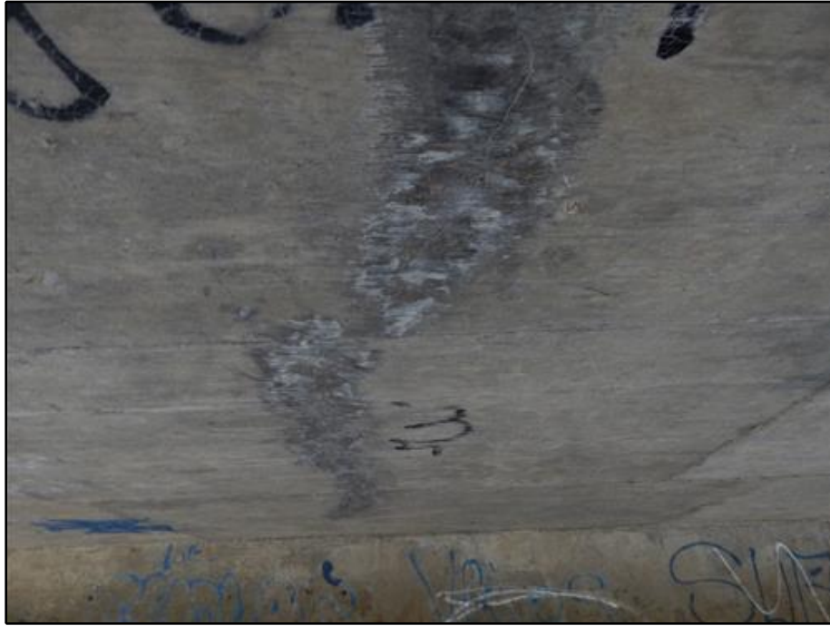
7. Soffit - Full-width Longitudinal Crack with Efflorescence
