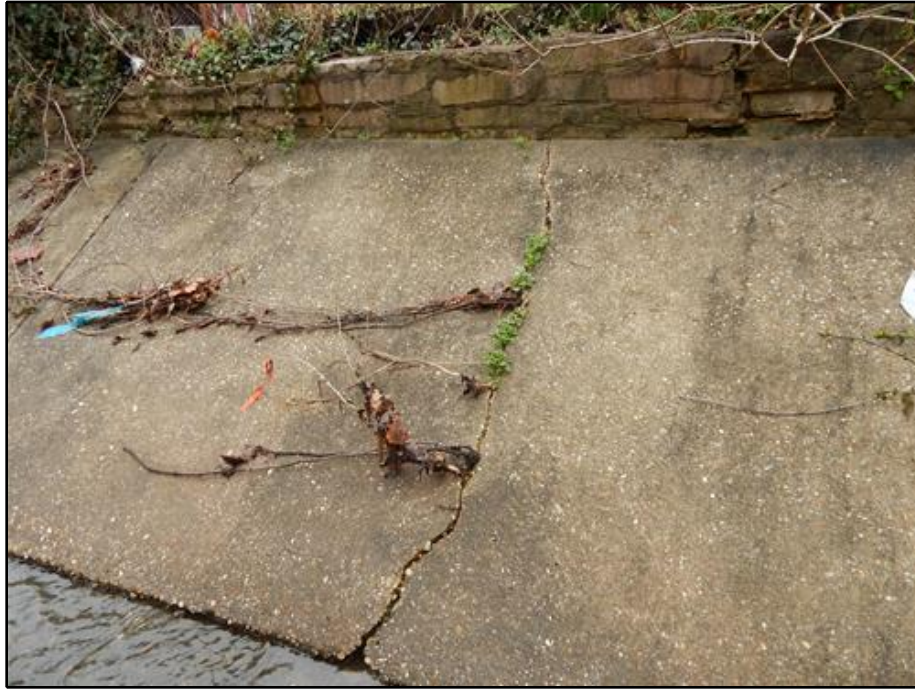
19. Slope Protection - Full-height Crack in Northeast Slope Protection 12' from Bridge
