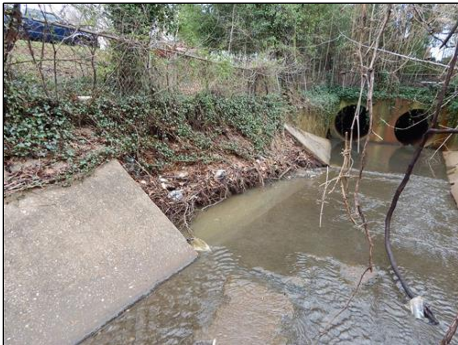
16. Slope Protection - Exposed Groundline Due to Washed Out Slope Protection Panel
