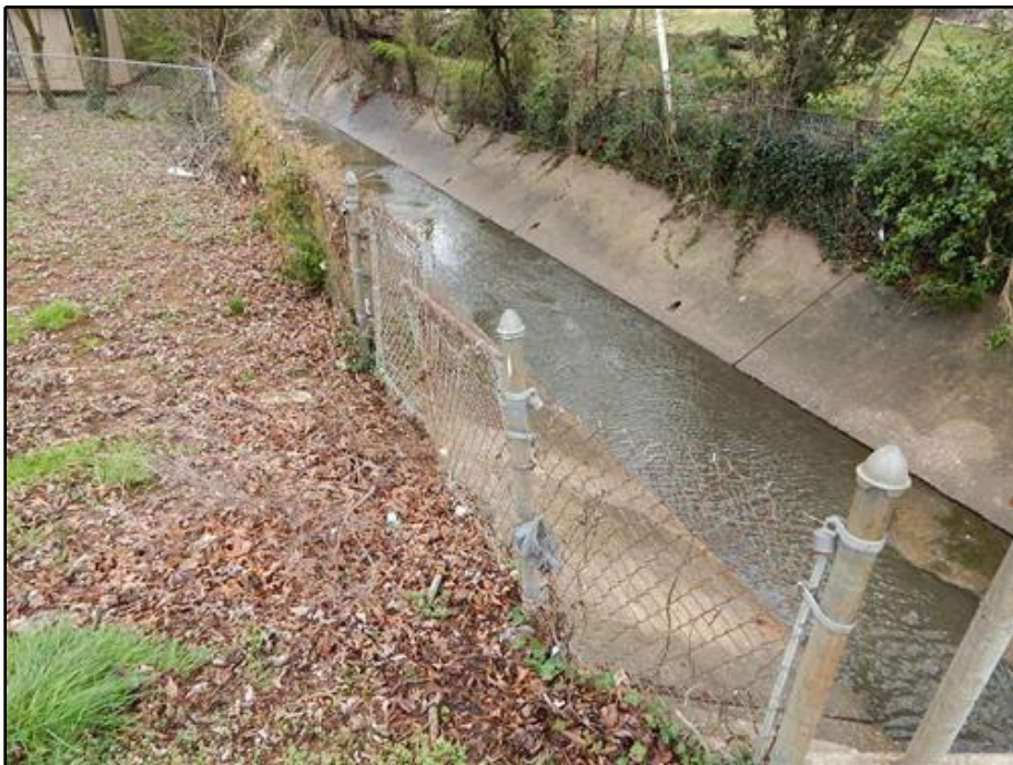
24. Fence - Disconnected Top Rail of Southeast Fence
