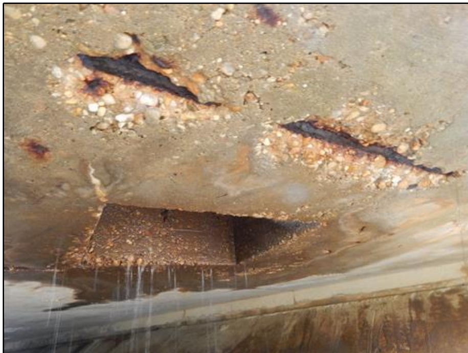
10. Deck - Spalls with Exposed Reinforcement in Top Slab of Span 2 at South End
