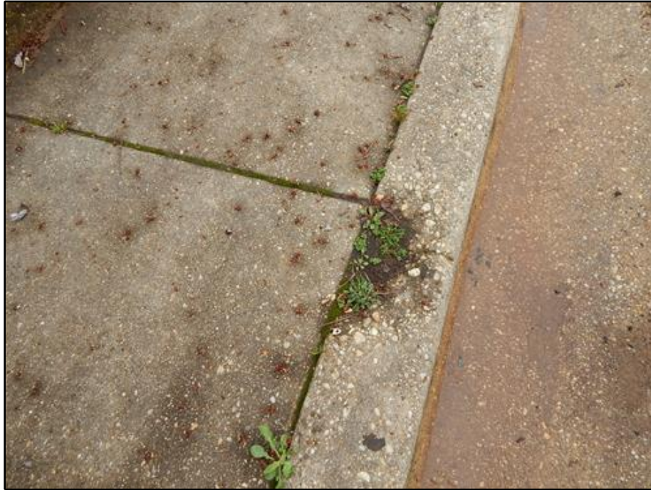
13. Curb - Spall in South Curb
