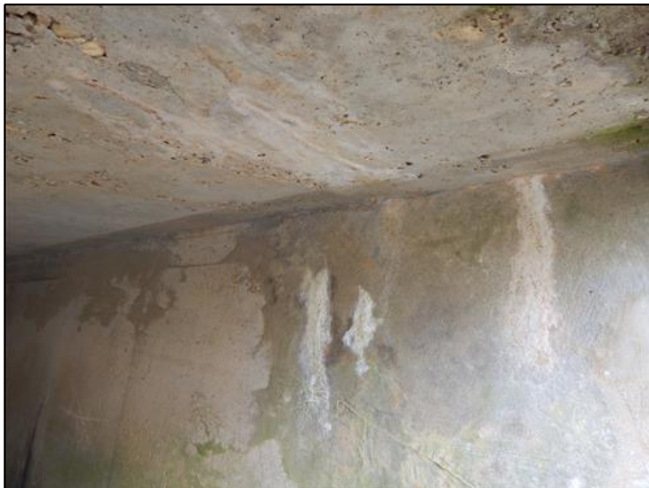
12. Deck - Typical Surface Spalls Throughout Top Slab of Span 2
