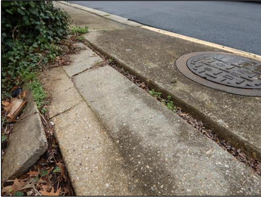
19. Sidewalk - Settled Sidewalk Panel adjacent to Southeast Storm Drain Inlet
