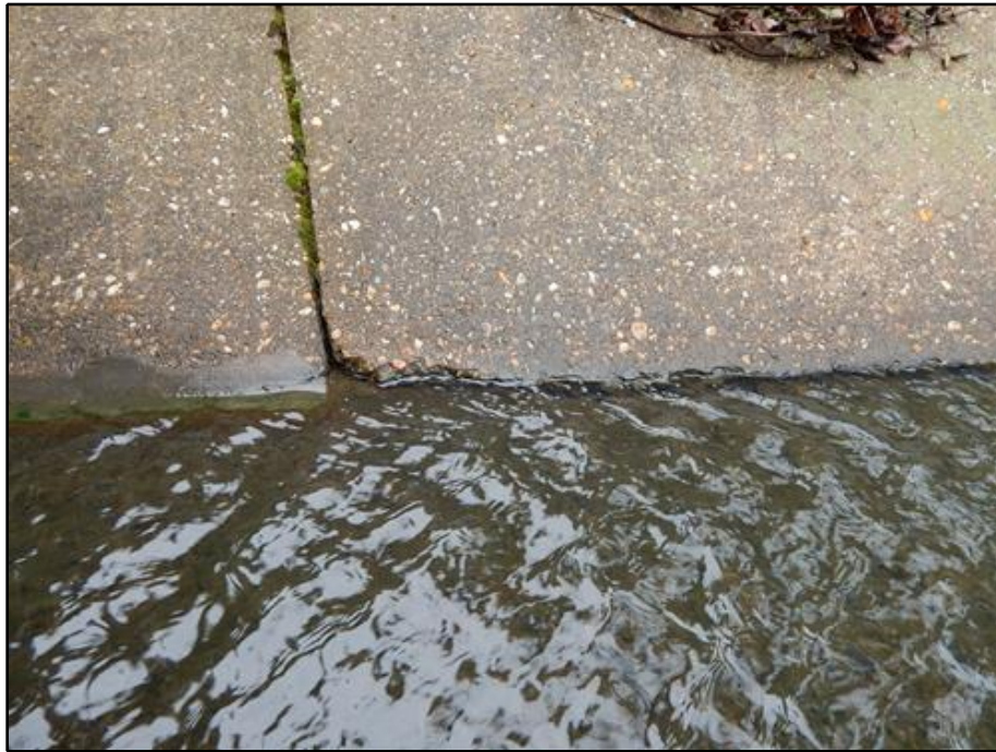
19. Slope Protection - Typical Scaling along Bottom of Slope Protection
