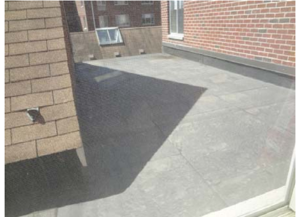
Photo #14: Small sections of roof have rubber roofing
