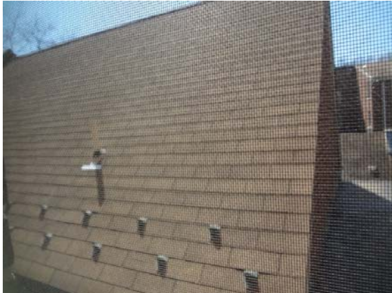
Photo #13: Majority of roof is 20 year 3-tab shingles
