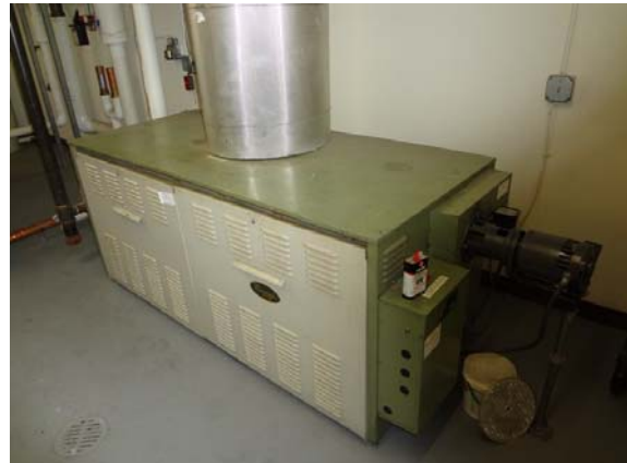
Photo #30: Domestic hot water boiler
