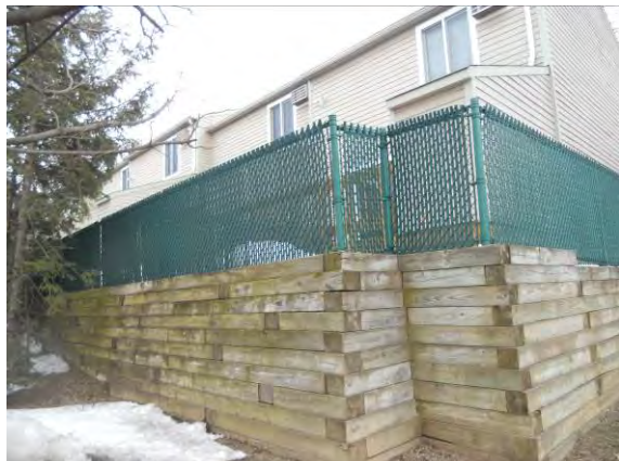
Photo #23: Timber retaining wall and fencing at DeSimone Court
