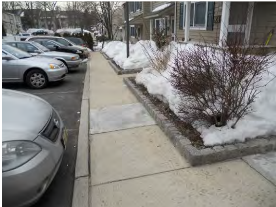
Photo #33: Concrete sidewalk with granite edging at DeSimone Court
