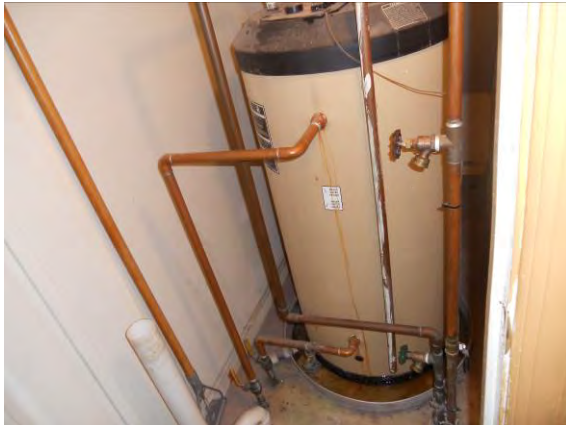
Photo #13: Domestic water heater storage tank with pan filled with water
