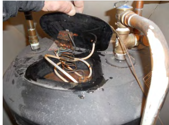
Photo #14: Rusted thermostat at top of domestic water heater storage tank
