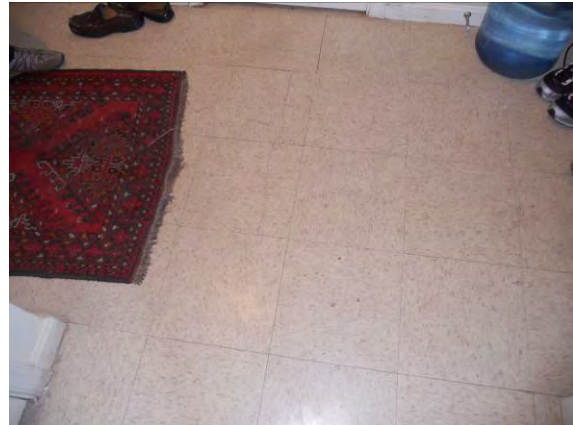
Photo #32: Cracked flooring due to water damaged subfloors ~ 30% units of DeSimone Court
