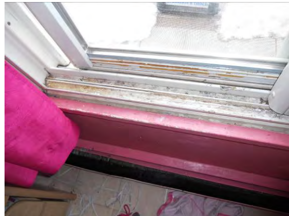
Photo #16: Close up of peeling paint at window frame
