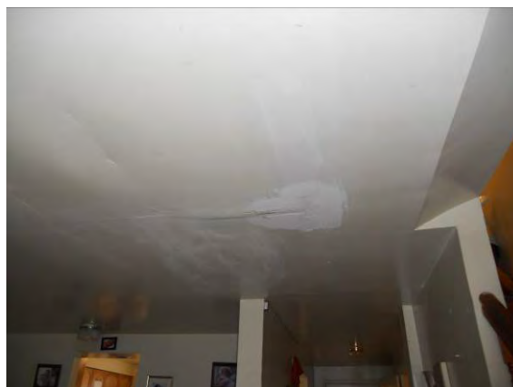
Photo #22: Patched ceiling from prior leak over living room
