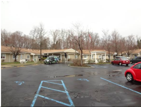
Photo #1: Front view, eastern elevation
