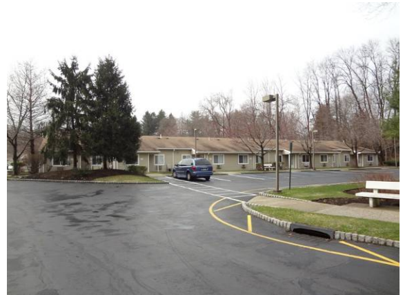
Photo #4: Right side, northern elevation
