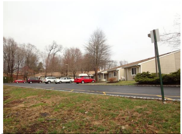
Photo #2: Left side, southern elevation
