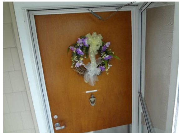
Photo #16: Both doors that provide access to tenant units are solid core wood doors
