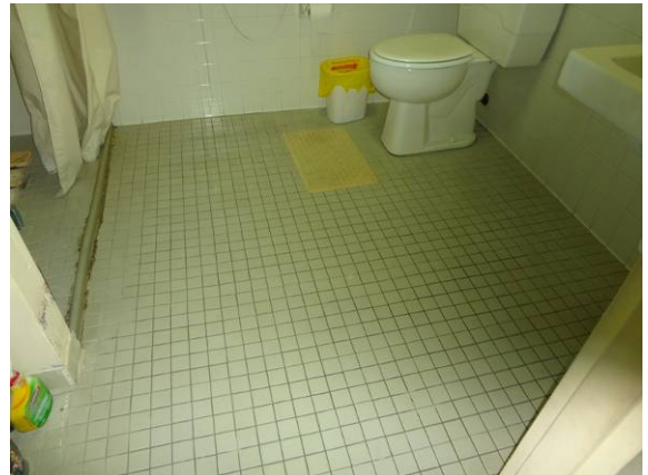
Photo #28: Resident unit bathrooms with roll in showers
