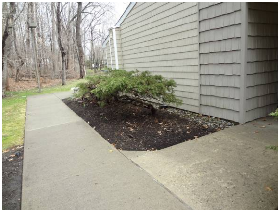
Photo #9: Concrete throughout site is in good condition
