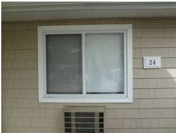
Photo #15: Windows throughout site are sliding double glazed
