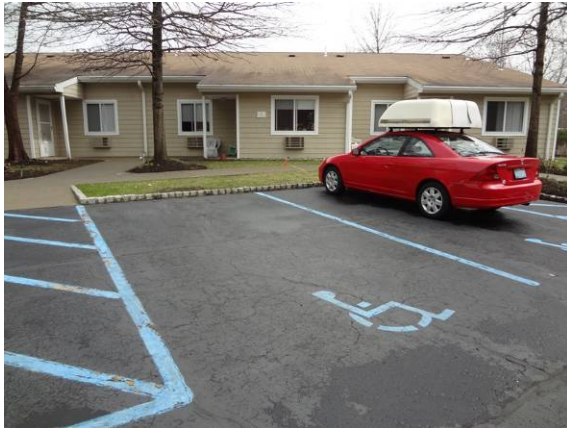
Photo #7: ADA parking throughout site does not have signage
