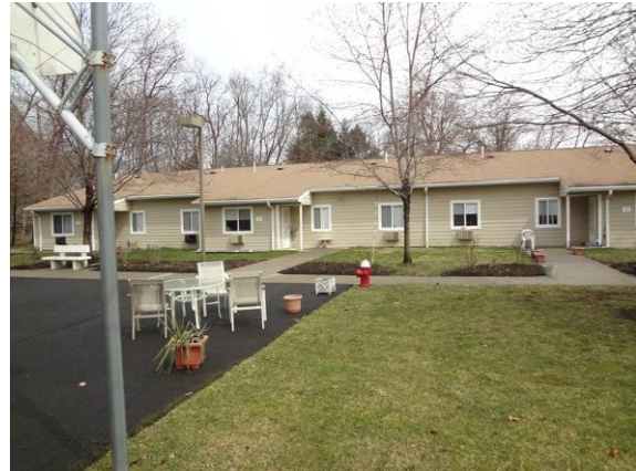
Photo #14: Roofs are in fair condition
