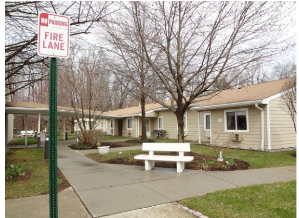
Photo #6: Twenty year, three tab shingles throughout property
