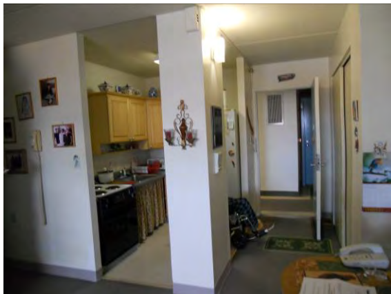
Photo #29: ADA apartment kitchen and entrance with no pull side clearance
