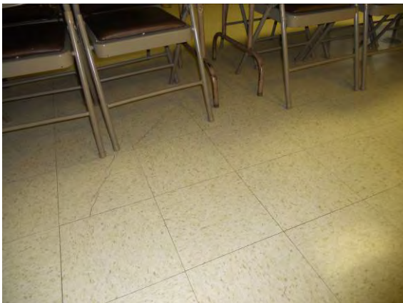
Photo #17: Crack in flooring in community room
