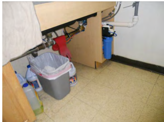
Photo #16: Non insulated drain lines under sink in community room kitchen
