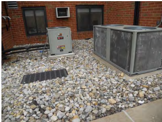
Photo #31: Condensing units
