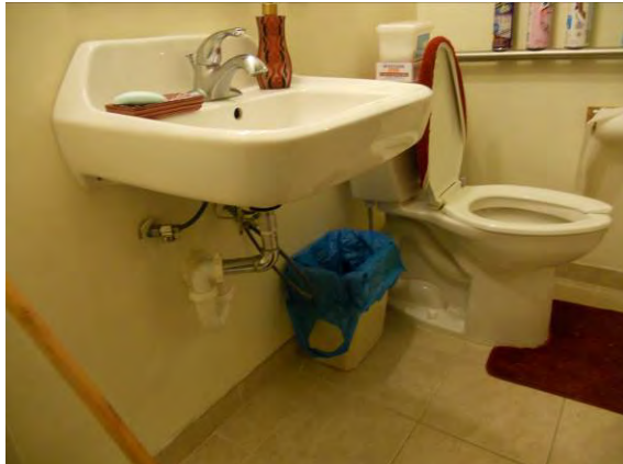
Photo #37: No drain pipe insulation or rear grab bar at toilet in ADA unit
