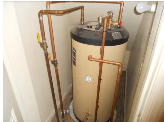
Photo #16: Storage tank for domestic water
