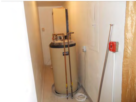
Photo #33: Domestic water storage tank in ADA unit with boiler in background
