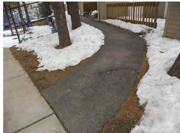
Photo #60: Asphalt sidewalk with isolated heaving from tree roots
