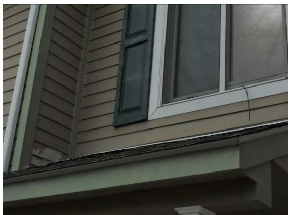
Photo #21: Damaged siding and loose window gasket
