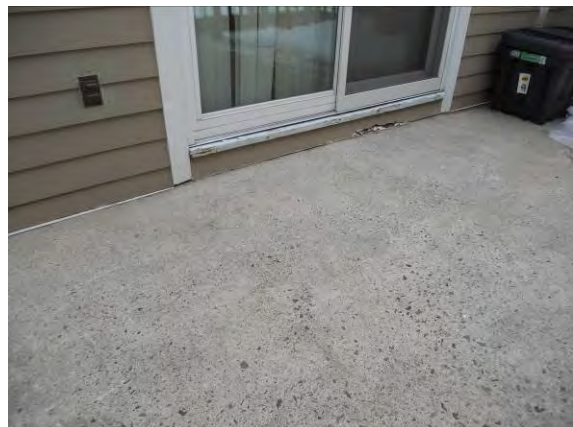
Photo #6: Damaged siding under sliding door
