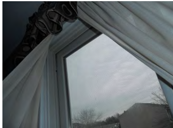
Photo #40: Window sash not sitting flush in frame
