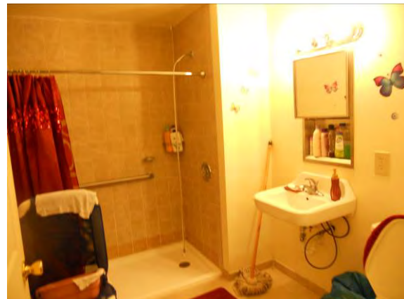
Photo #36: ADA unit bathroom with no drain pipe insulation or hand-held shower mount
