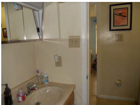
Photo #27: Unit bathroom with non-GFCI test type receptacle
