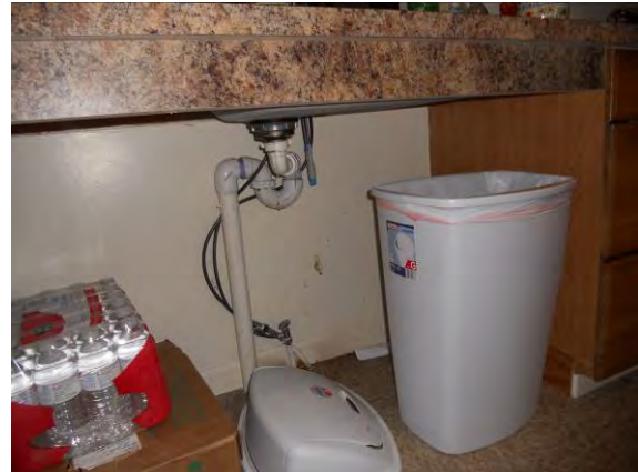
Photo #32: Non-insulated drain pipe in kitchen of ADA unit
