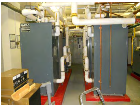
Photo #17: Domestic water storage tanks
