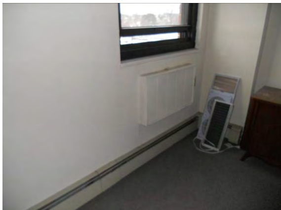
Photo #43: Apartment unit hydronic heat baseboard and covered through the wall air condition unit
