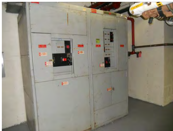
Photo #14: Main electrical switchgear
