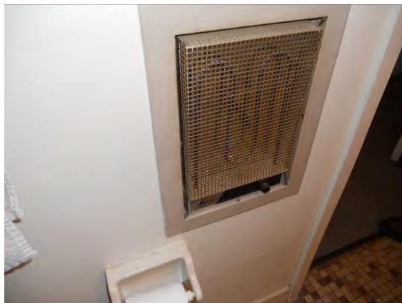
Photo #44: Electric resistance heater in apartment unit bathroom – 5 th floor only
