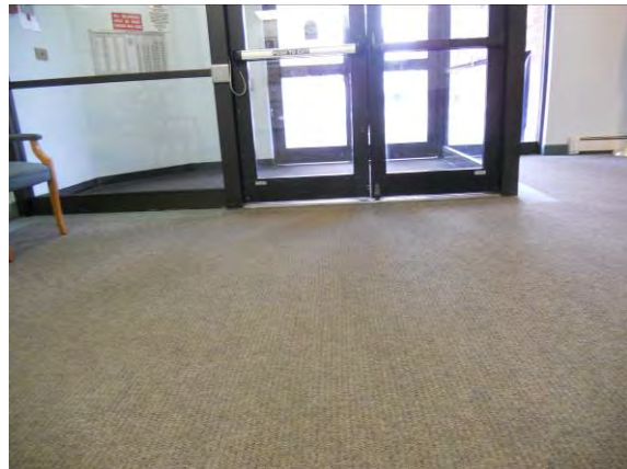
Photo #62: Main lobby entrance seeing daylight under door frame at both sets
