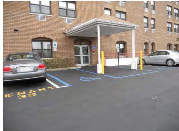
Photo #6: Rear entrance with additional ADA stalls and no access aisle markings
