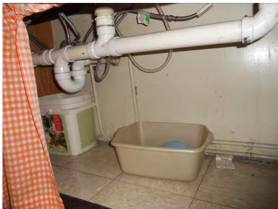
Photo #31: Non-insulated drainage piping under community room kitchen sink
