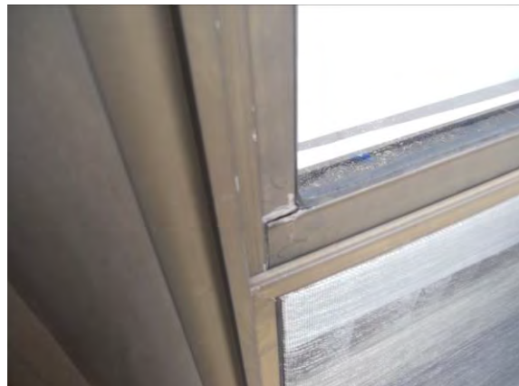
Photo #66: Exterior of window frame showing cracked window frame sealant at joint
