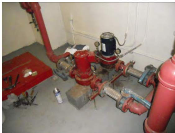
Photo #16: Circulation pumps including newly replaced one
