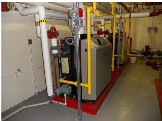
Photo #15: Boilers for domestic water and heat
