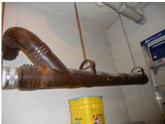
Photo #21: Waste line with corrosion in basement
