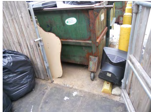
Photo #8: Dumpster, enclosure and bollards with concrete fill pushing up and out of tops
