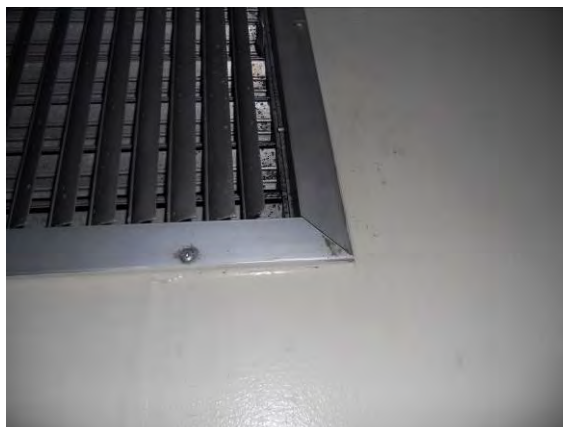
Photo #54: Suspect mold in supply vent in corridor
