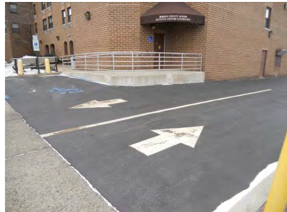
Photo #4: Driveway entrance and front ADA stall with no access aisle markings
