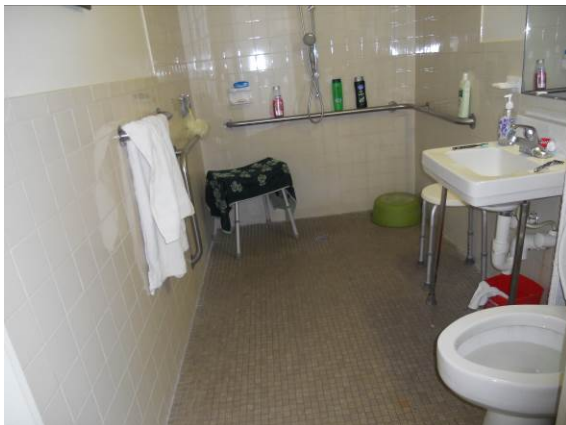
Photo #53: Apartment ADA unit with roll-in shower
