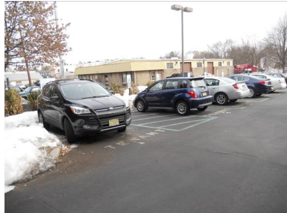
Photo #14: ADA parking with post signage at non-compliant heights
