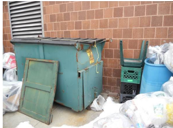
Photo #10: Damaged Dumpster
