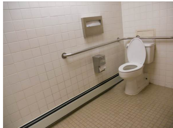
Photo #42: Common area men's restroom
