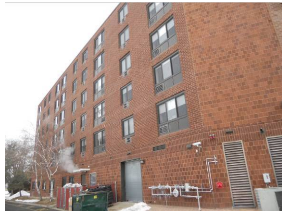
Photo #4: West elevation
