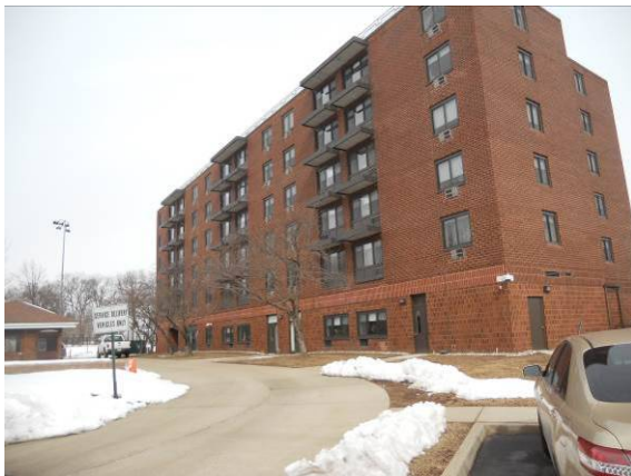
Photo #3: Rear southwest elevation
