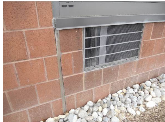
Photo #12: Separating construction joint
