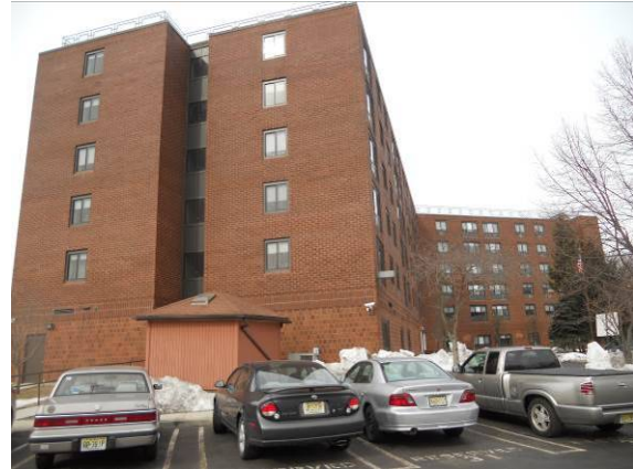
Photo #2: Southeast end elevation
