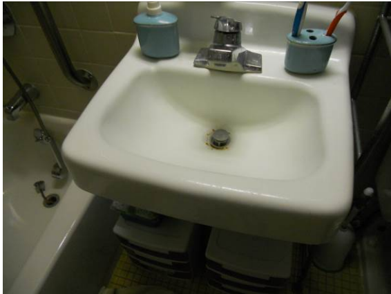
Photo #55: Apartment unit lavatory condition
