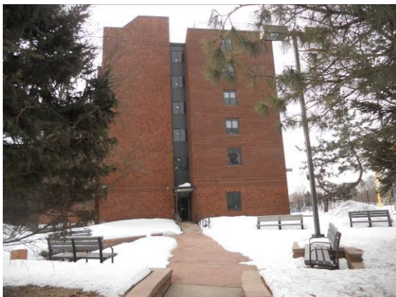
Photo #5: North elevation
