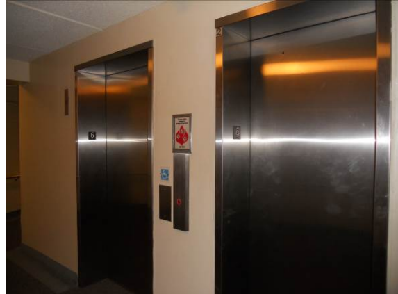
Photo #20: Elevator lobby
