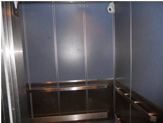
Photo #21: Elevator cab interior
