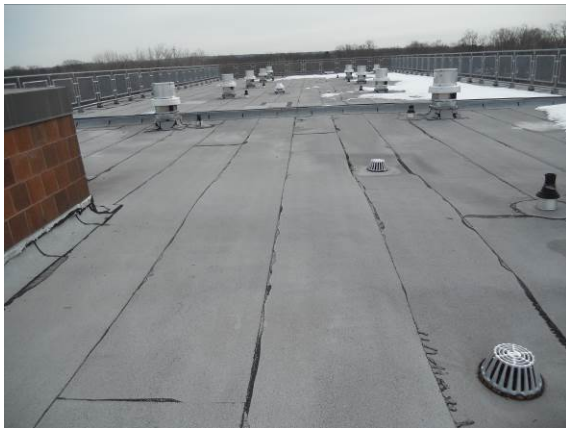
Photo #15: Roof overview
